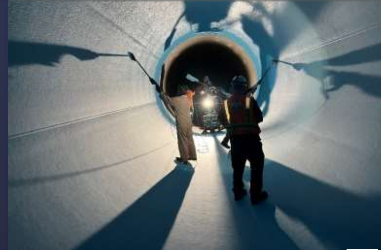
Final coating of pipe after lining repair
