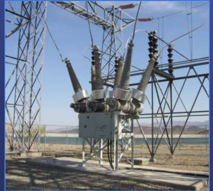
230 kV Circuit Breaker
