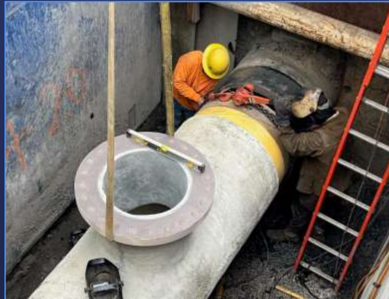
Installing Closure Piece
