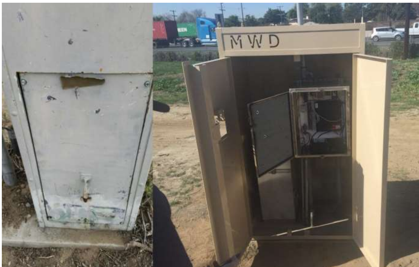
Newly reinforced meter cabinets protect vulnerable electronic components well into the future
