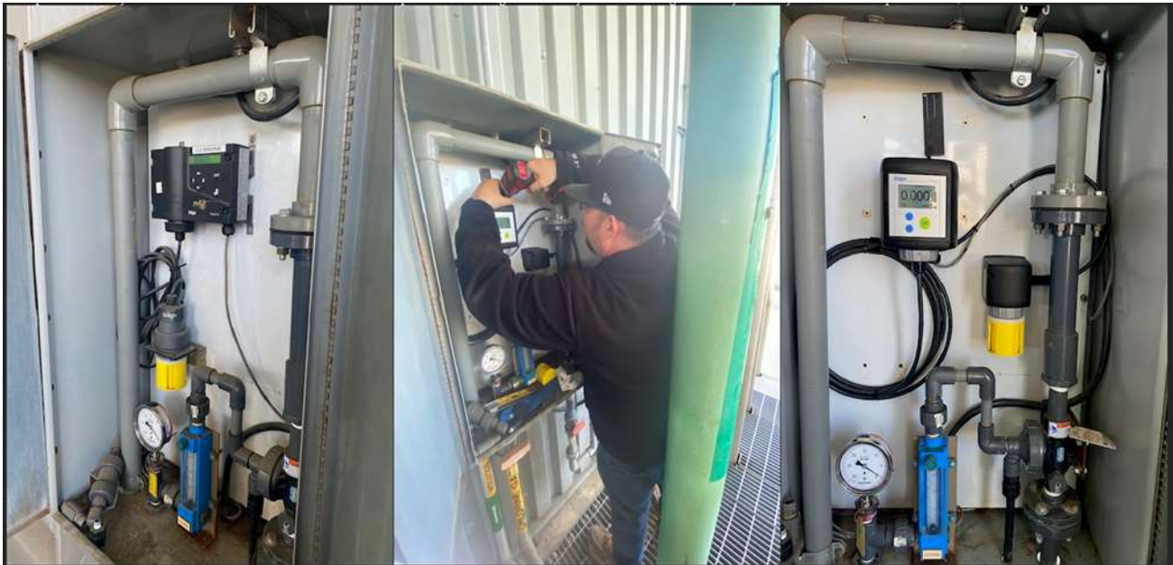
Failed chlorine leak detector (left); staff installing new chlorine leak detector (center); and newly installed chlorine leak detector (right) at the Weymouth plant
