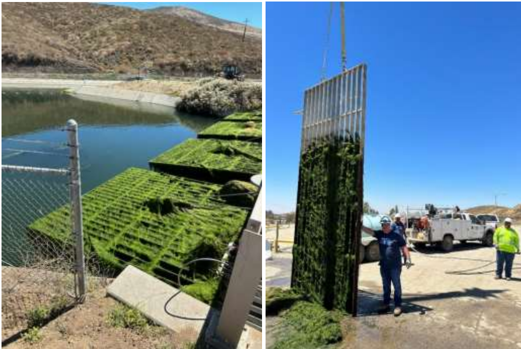
Staff removing algae from debris racks at the San Diego Canal
