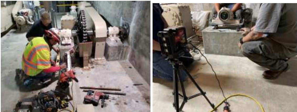
The contractor core drilling pillow block pedestals (left) and performing alignment procedure (right) at the Jensen plant
