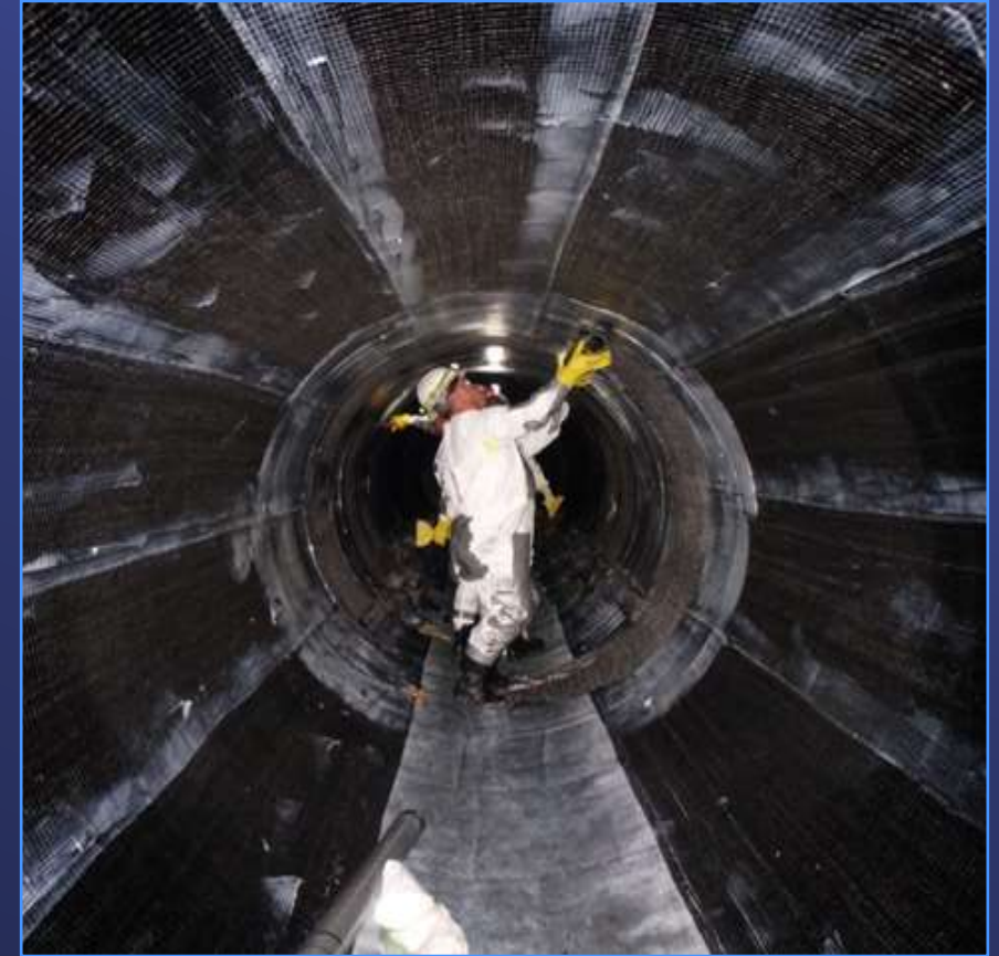
Previous Carbon Fiber Repair Second Lower Feeder
