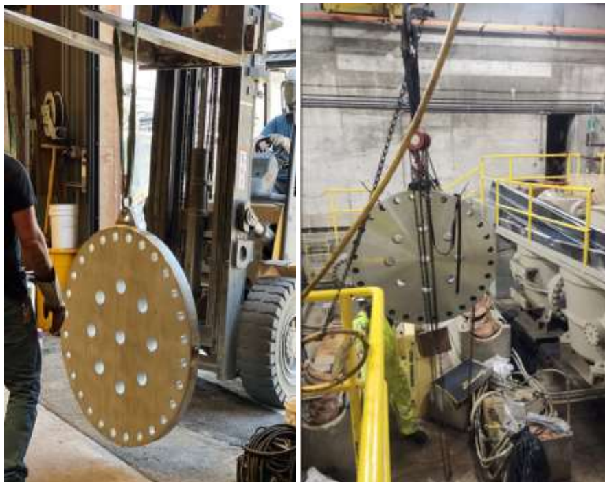
Two multi-orifice plates being installed at Covina PCS
