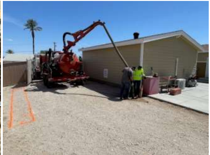
Footing formed to protect utility (left) and staff potholing buried utilities (right) at a Desert housing unit
