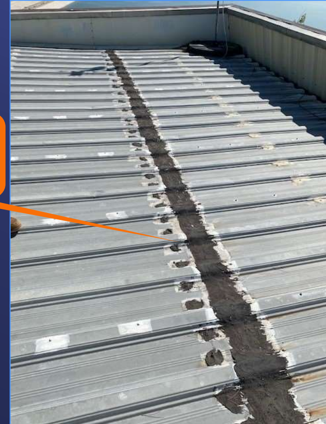
Deteriorating Metal Roof & Temporary Roof Repairs
