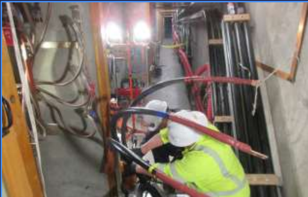
Switch house cable installation
