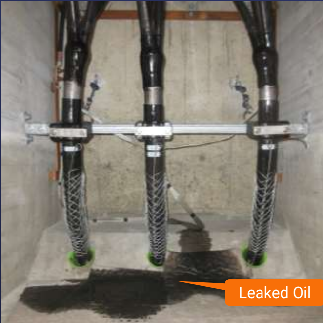
Leaking Termination
