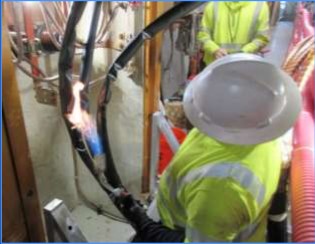
Application of heat to the termination kit
