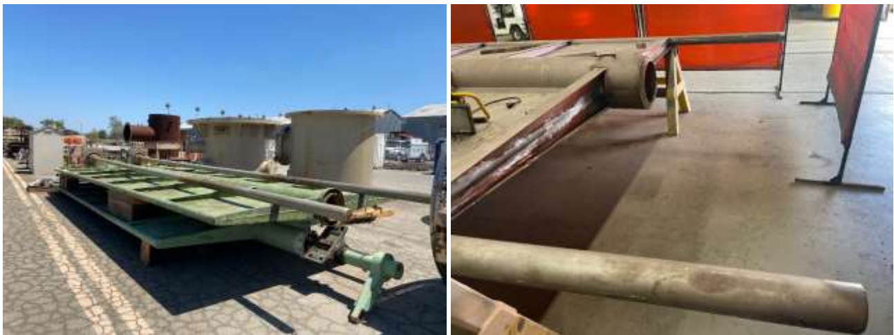
As received condition of wing gates (left) and removal of corroded gate components (right) for DWR
