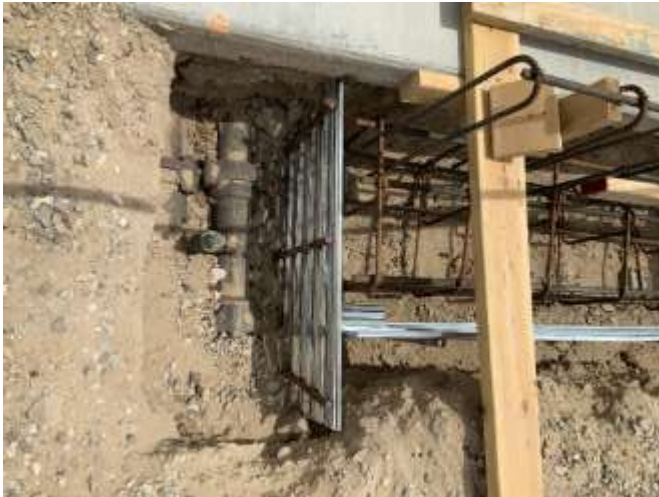
Footing formed to protect utility (left) and staff potholing buried utilities (right) at a Desert housing unit
