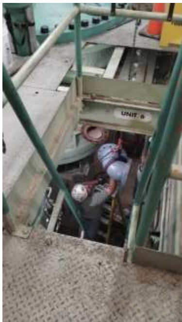
Staff installing rebuilt discharge valve bypass system components at a Desert facility
