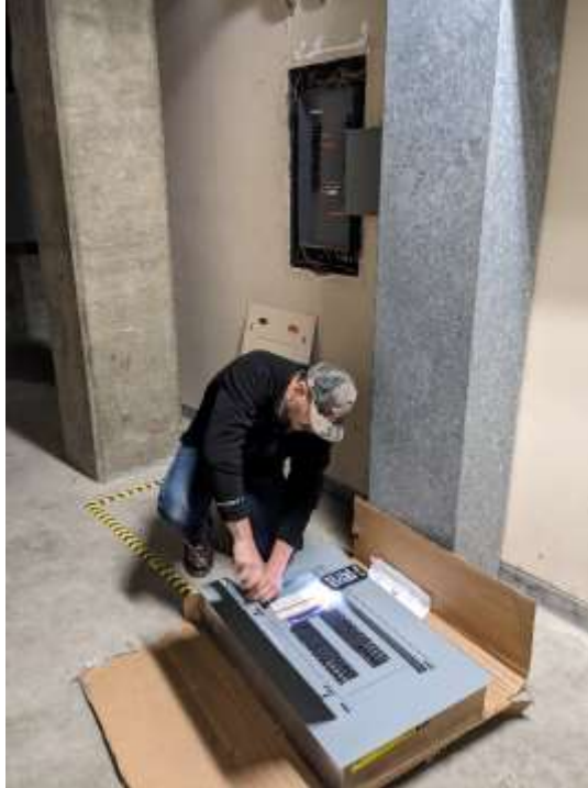
Staff preparing a new breaker panel for installation at the Diemer plant
