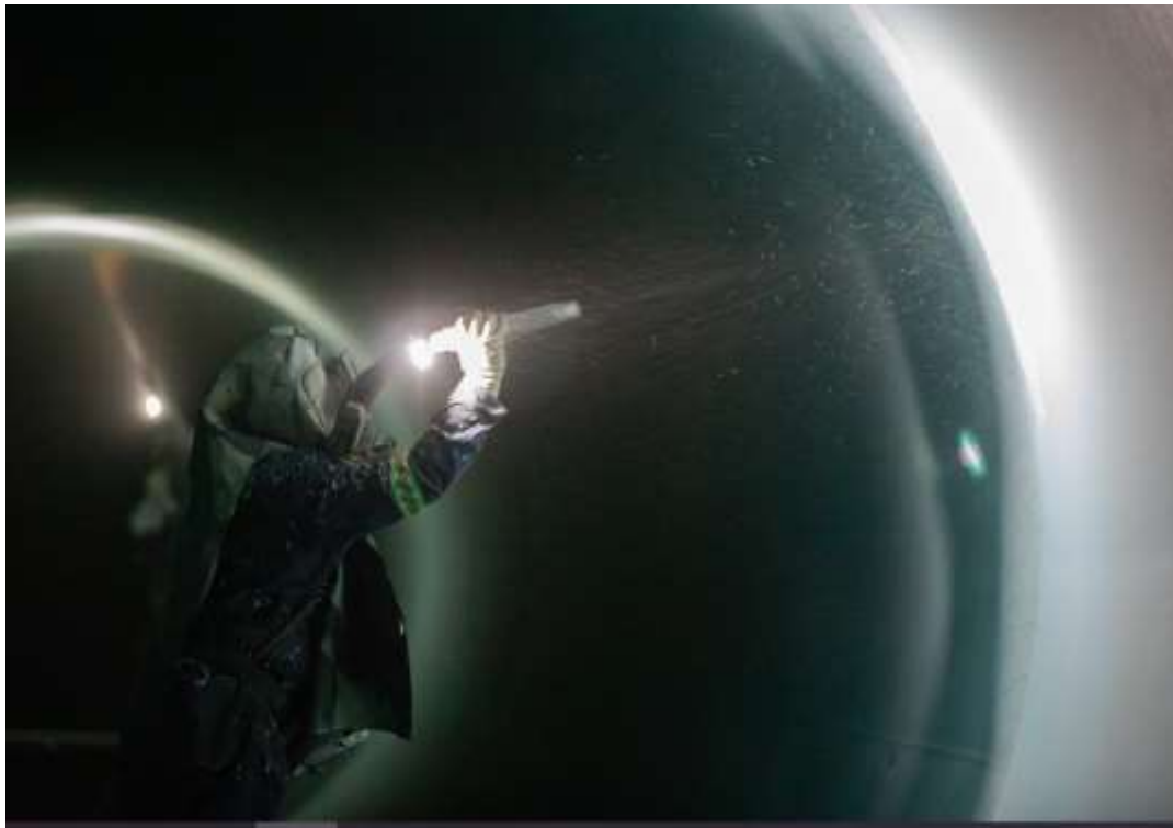
Etiwanda Pipeline Relining—Applying Polyurethane Coating Lining
