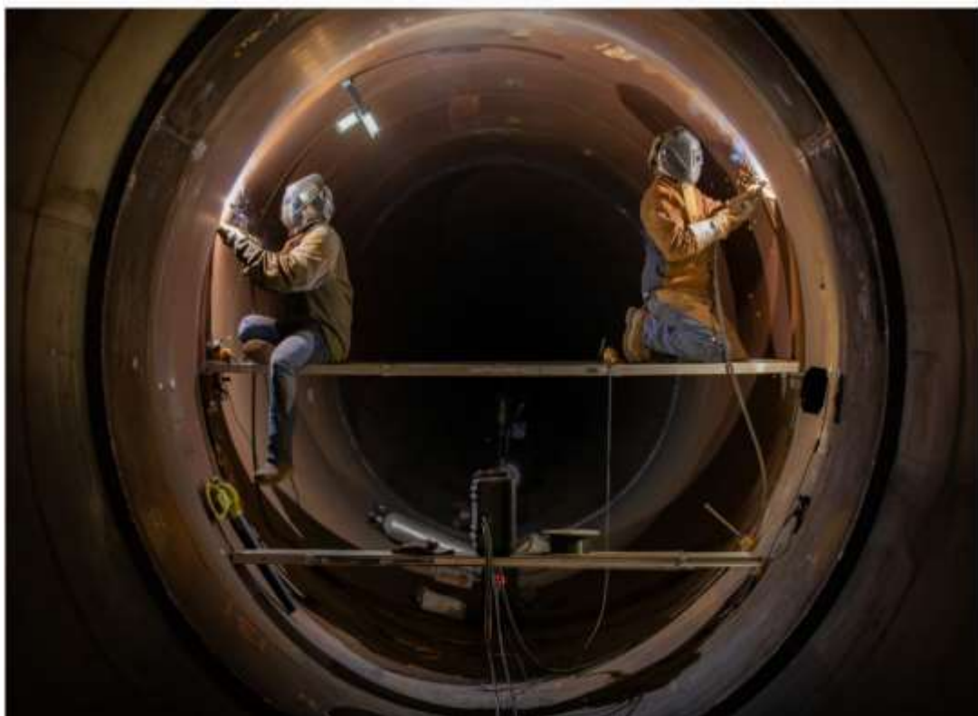
Etiwanda Pipeline Relining—Welding Steel Pipe Reducers
