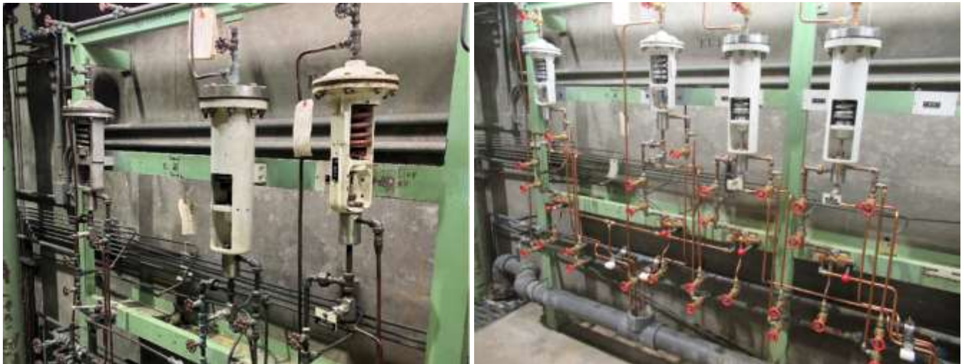
Before (left) and after (right) rehabilitation of the pilot rack at Oak Street PCS
