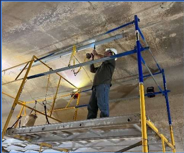
Typical transducer installation in aqueduct
