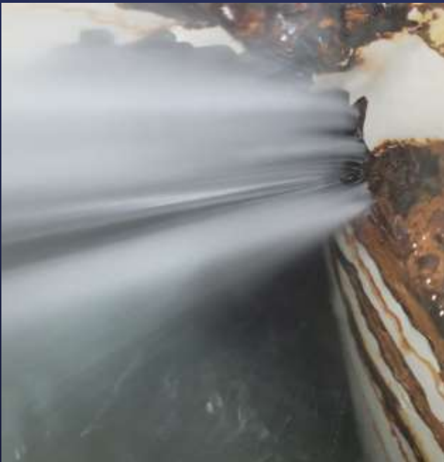
Leak on DWR's 12" Bypass Line at Northpark Valve Vault
