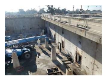
Weymouth Basins 5–8 and Filter Building No. 2 Rehabilitation Removal of original gates from Basin 7
