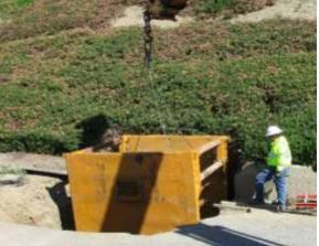
Staff excavating between structures (left) and installing a shoring box (right) at the Diemer plant
