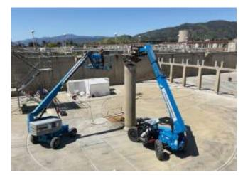
Weymouth Basins 5–8 and Filter Building No. 2 Rehabilitation Removal of original clarifier equipment from Basin 7
