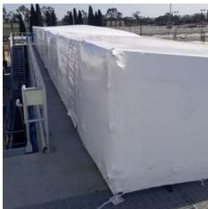
Installation of an enclosure over bioreactors to support SCAQMD air permit source testing at the demonstration plant
