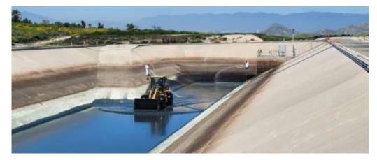
Staff hosing down debris and using a front loader to push solids towards the pump for removal at the Mills plant
