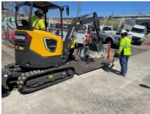
Staff using an electric mini excavator for a new duct bank along the Palos Verdes Feeder
