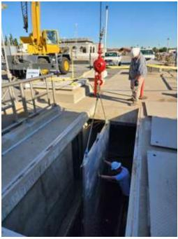
Staff using a crane to lower the isolation gate (left) and guiding the isolation gate (right) into the Effluent Channel at the Weymouth plant
