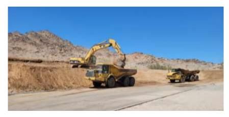
Excavation work to facilitate an electrical system rehabilitation project at Iron Mountain pumping plant
