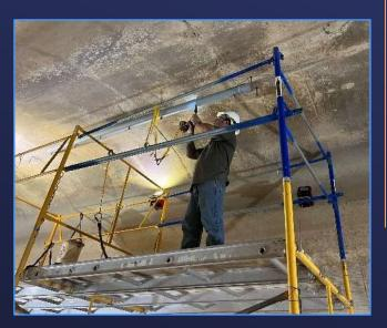
Typical transducer installation in aqueduct
