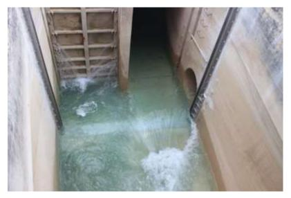
Blocker gate installed stopping water flow in first barrel of Whitewater Siphon
