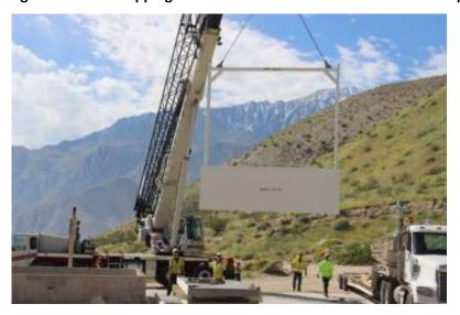
Transition weir gate being placed into position at Whitewater Siphon
