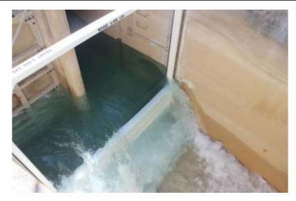
Transition weir gate installed to back up water at Whitewater Siphon and increase storage deliveries
