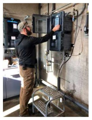
Staff repairing the Finished Water Reservoir Inlet's ammonia analyzer at the Skinner plant
