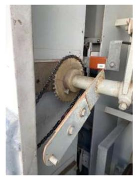
Disconnect switch with new operating chain installed at Lake Mathews HEP
