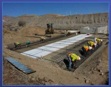
Typical Concrete Protective Slab
