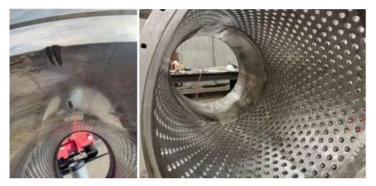
Damage discovered on outer valve body (left) and completed weld repairs (right) for Red Mountain PCS
