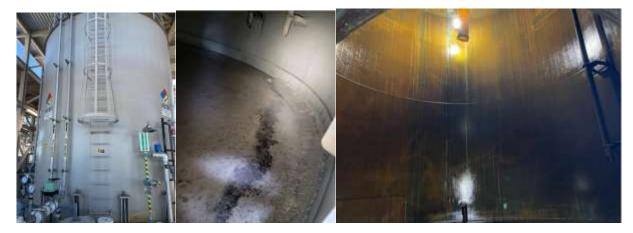
Outside of sulfuric acid tank (left); tank inside before cleaning (center); and inside tank after cleaning (right) at the Diemer plant
