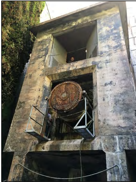
Photo 1. Existing valve house. The discharge valve is located in the lower floor of the valve house.
