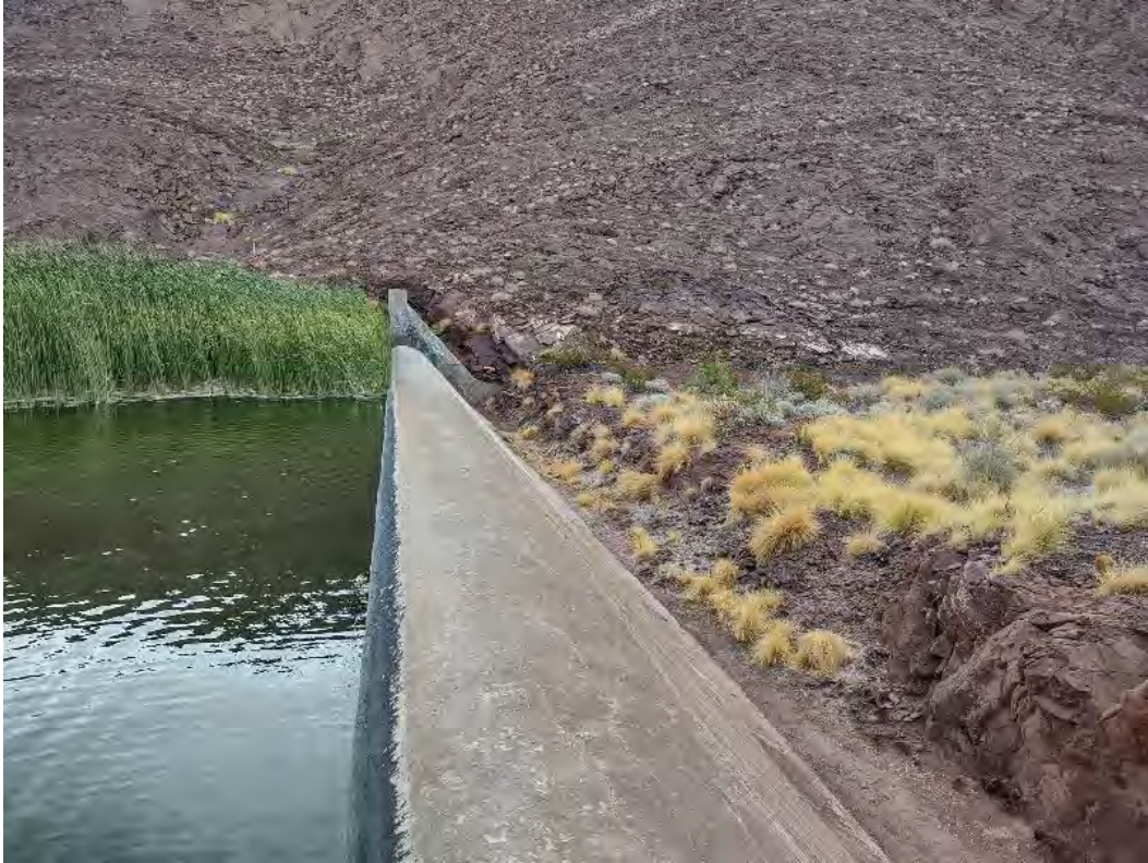
Figure 22. Northern end of ogee spillway structure looking north-northeast. Source: HELIX
