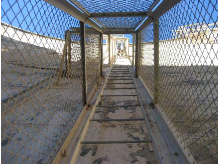
Figure 16. Ladder ascent on the downstream face of dam. Source: Metropolitan
