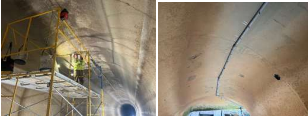
Staff installing conduit (left) and the completed installation (right) along the top of the Hayfield Tunnel
