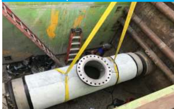
Pipe Segment Installation
