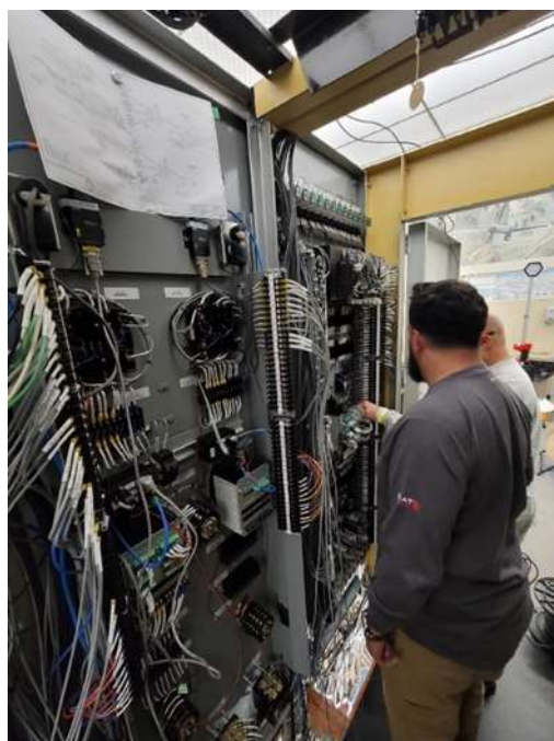
Staff verifying final wiring of new panels and relays at Hinds pumping plant
