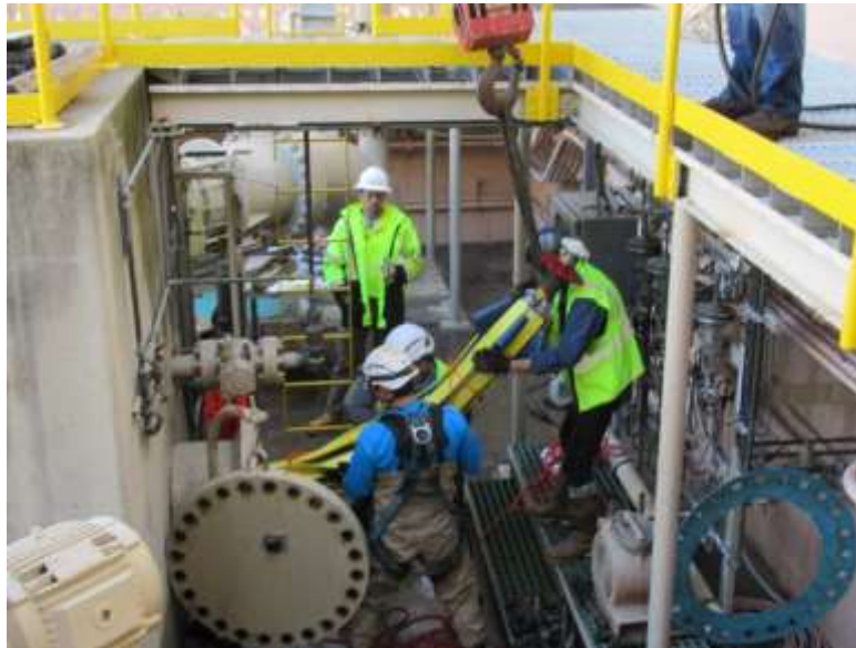
Metropolitan and contractor staff removing pipe-diver at Sepulveda PCS
