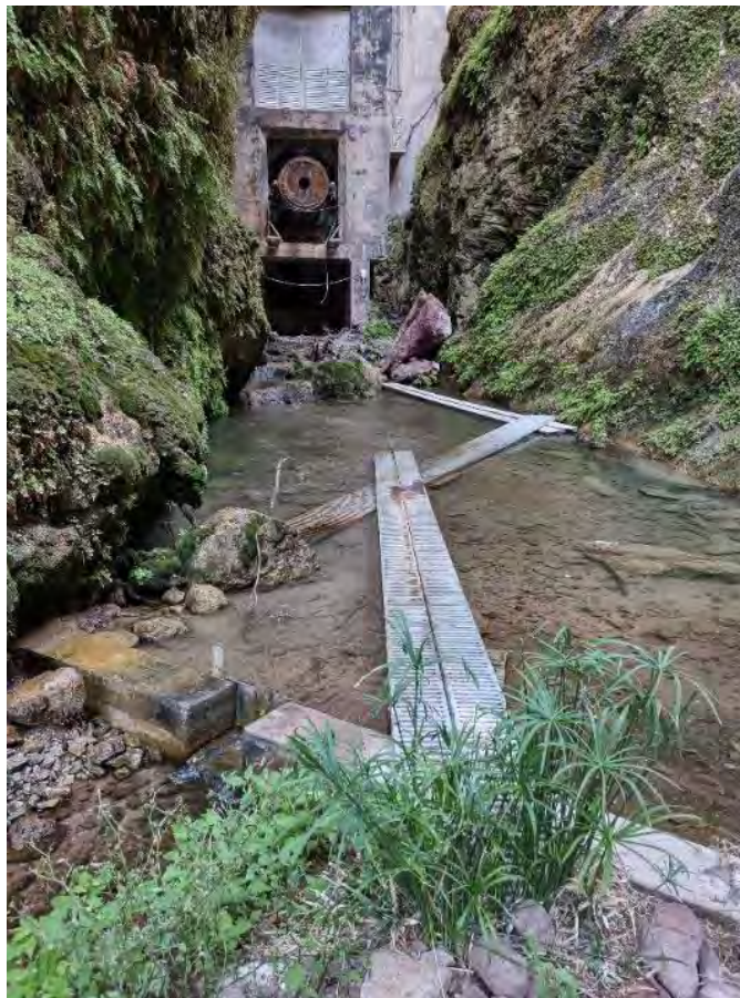
Figure 17. Valve with the Howell-Bunger valve, louvred doors and metal platforms, and main weir and catwalk panels in foreground, looking west. Source: HELIX
