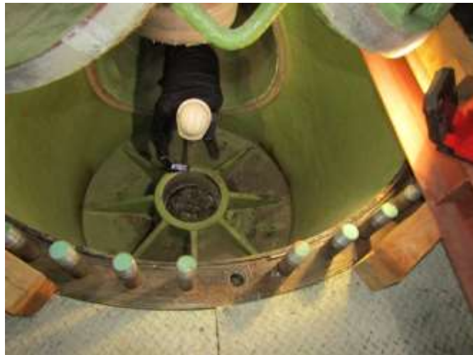
Staff performing measurements of the discharge valve at Eagle Mountain pumping plant
