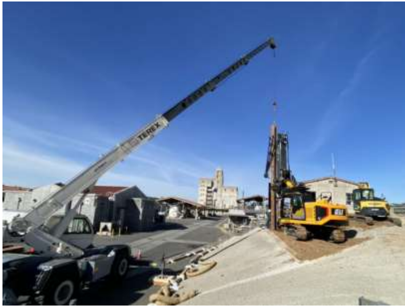
Weymouth Basins 5-8 and Filter Building No. 2 Rehabilitation—Installing crane pad
