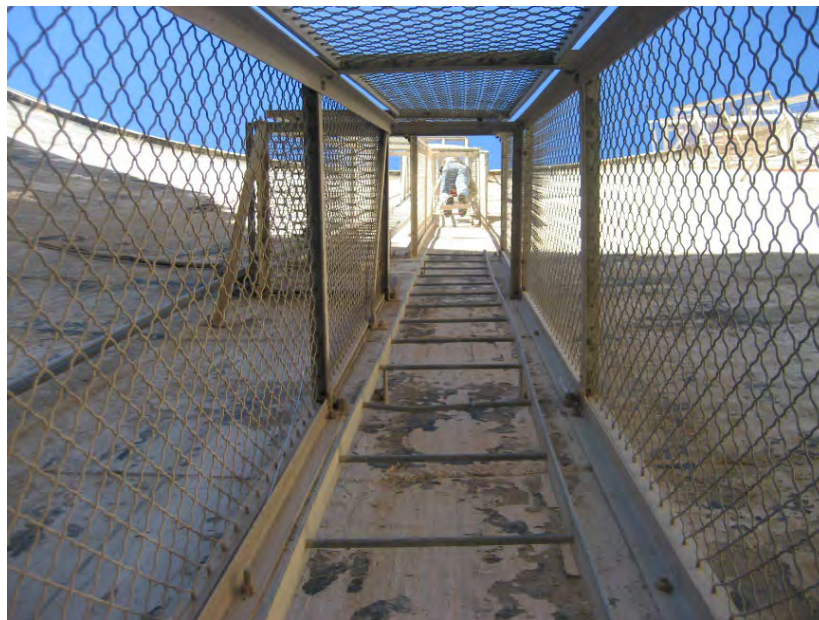
Figure 5. Ladder ascent on the downstream face of dam. Source: Metropolitan
