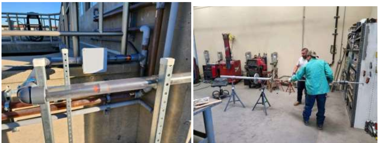
Double containment piping (left) and new containment lance (right) for fluoride injection feed line at the Weymouth plant
