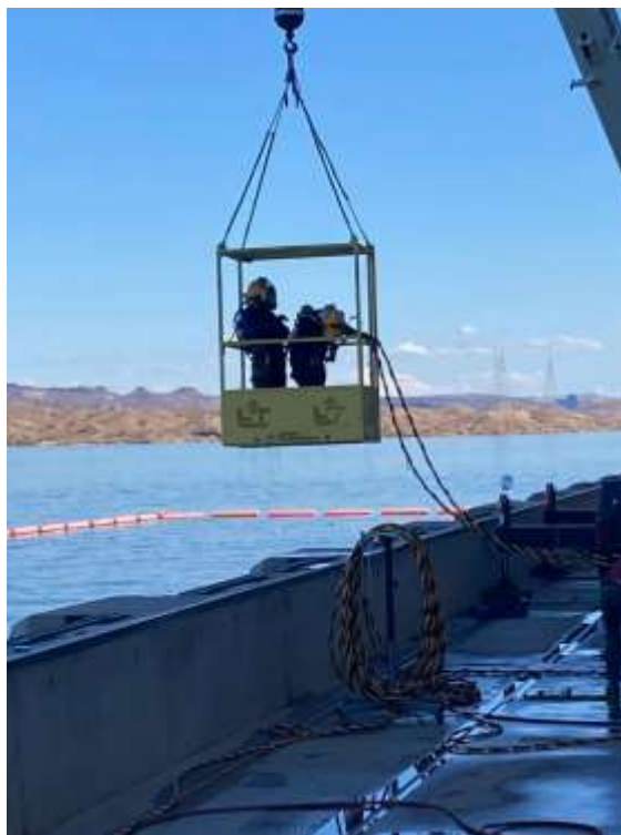
Staff preparing to perform underwater cleaning at Intake pumping plant
