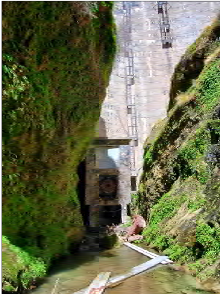
Photo 3. Existing valve house with ladder to the upper right and catwalk to the bottom center. A new galvanized steel walkway would replace the catwalk, and a steel grate platform would be constructed in front of the valve house. The walkway would connect to the platform by a new concrete staircase.
