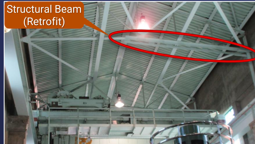
Seismic Retrofit
