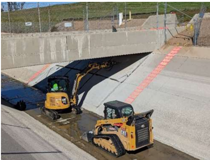
Staff removing (left) and replacing damaged concrete panels (right) on the San Diego Canal
