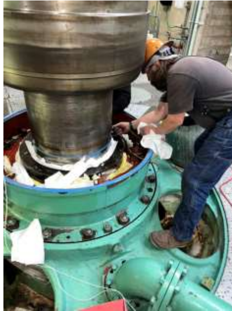
Staff replacing an RTD on pump bearing at Eagle Mountain pumping plant
