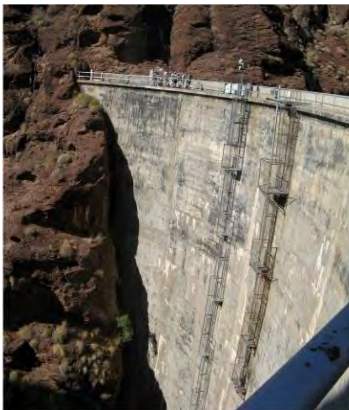
Figure 15. Downstream face of Copper Basin Dam, with attached main ladder (left) and plumb line ladder (right), looking southwest. Source: Metropolitan
