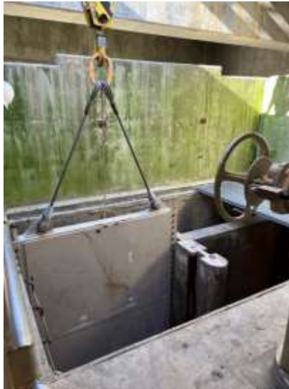
A large gate lowered into the CRA defines the beginning of the Casa Loma Siphon clearance
