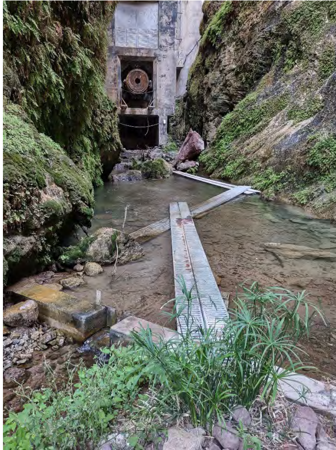
Figure 6. Valve with the Howell-Bunger valve, louvred doors and metal platforms, and main weir and catwalk panels in foreground, looking west. Source: HELIX
