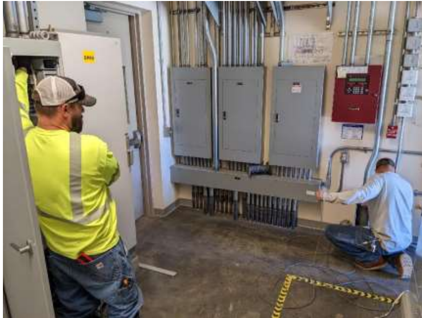
Staff upgrading hazmat storage area sensor cables at the Diemer plant
