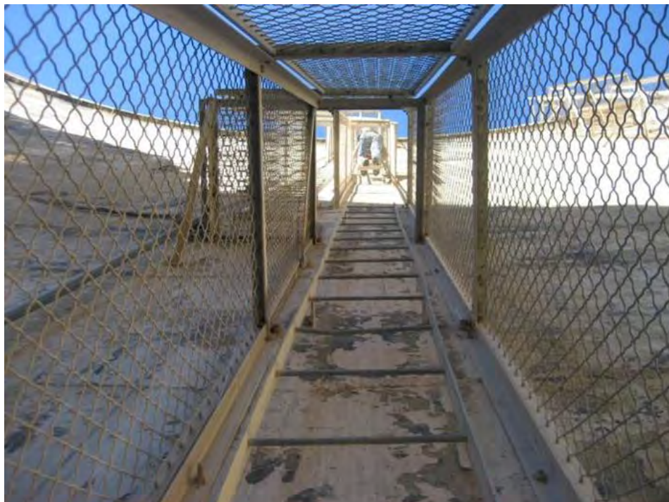
Figure 4. Ladder ascent on the downstream face of dam. Source: Metropolitan
