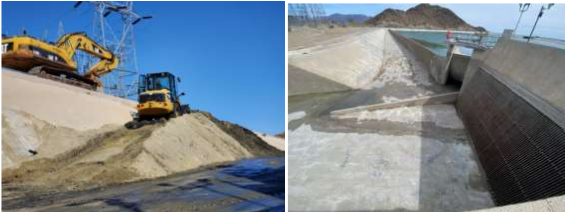
Eagle Mountain inlet channel before (left) and after cleaning (right) with heavy equipment
