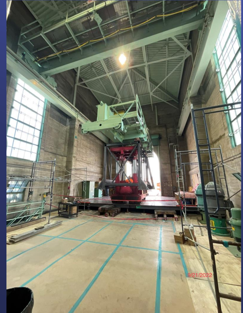
New Crane Girder Installation @ Gene
