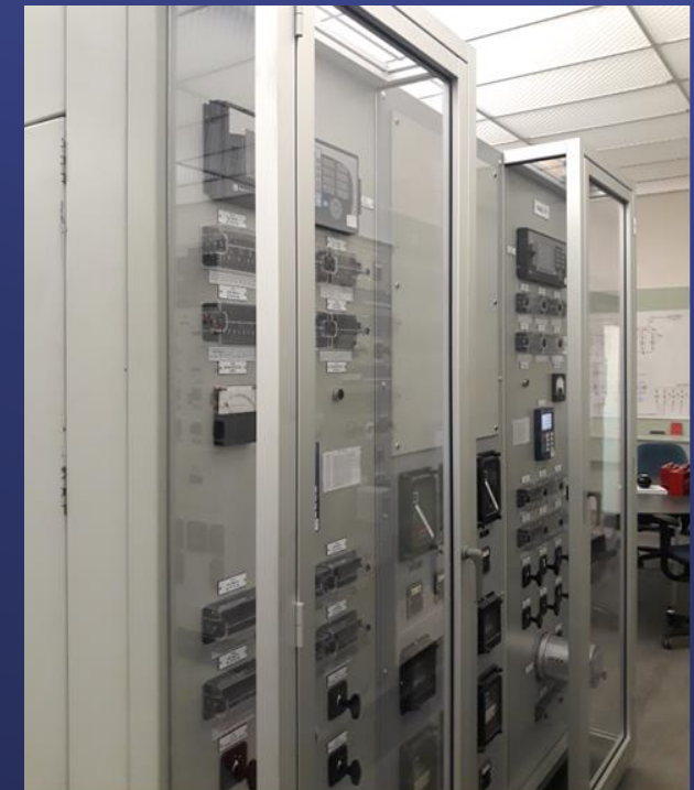
Protective barrier for BES asset at Eagle Mtn pump plant (installed in 2022)
