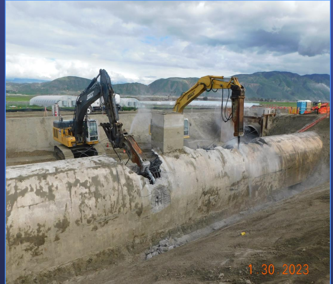
Demolition of existing siphon at tie-in location
