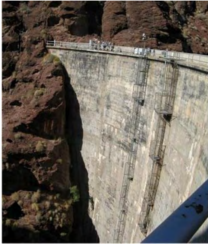
Figure 3. Downstream face of Copper Basin Dam, with attached main ladder (left) and plumb line ladder (right), looking southwest. Source: Metropolitan
