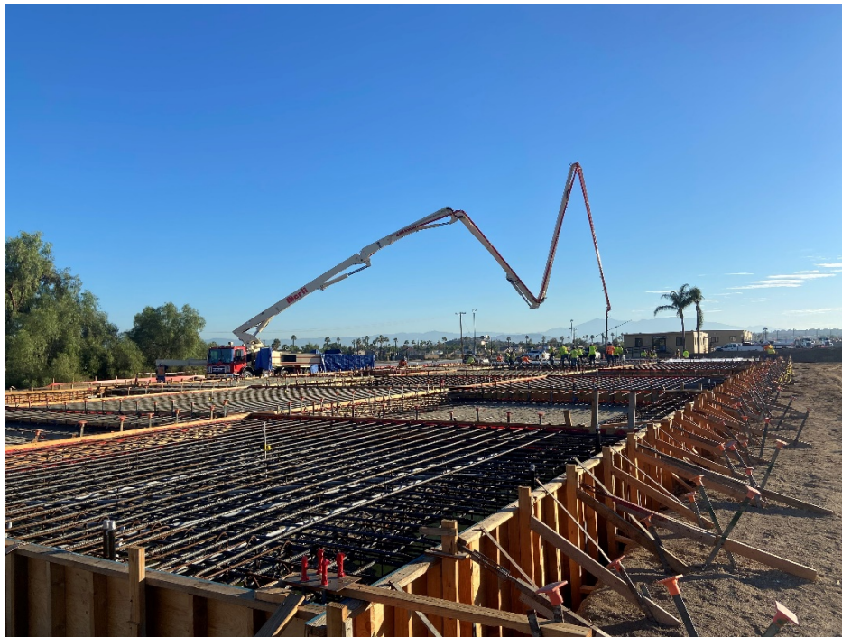
Contractor placing concrete for Lake Mathews PCCP Valve Storage Building pad
