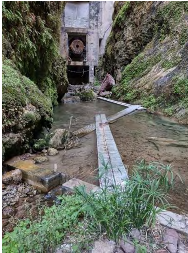
Figure 5. Valve with the Howell-Bunger valve, louvred doors and metal platforms, and main weir and catwalk panels in foreground, looking west. Source: HELIX
