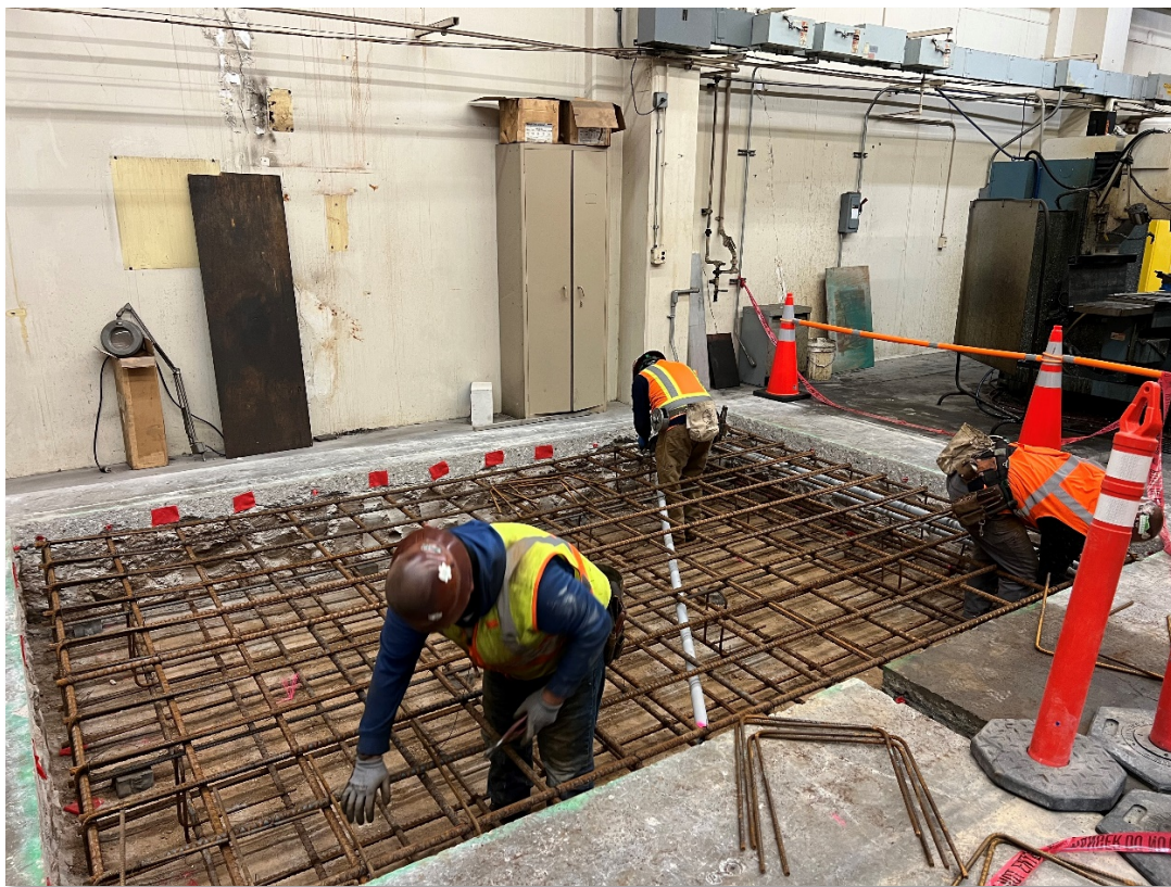
Contractor installing rebar for press brake foundation at La Verne Shop
