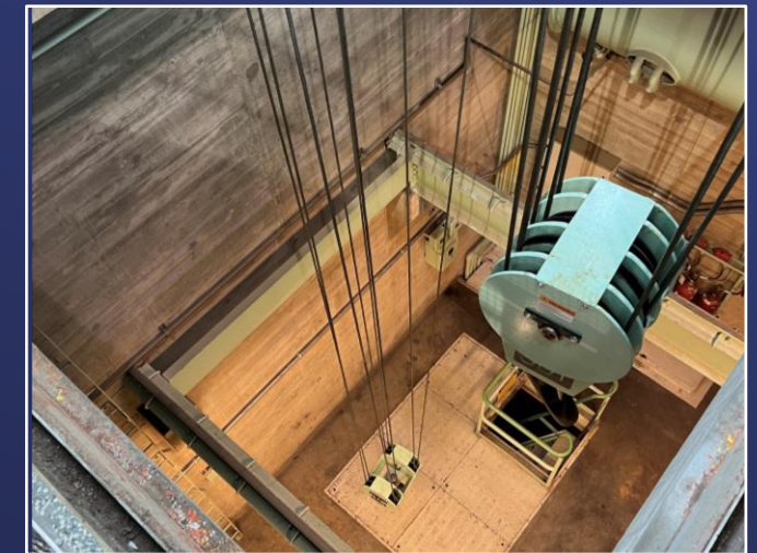
Hoists Below Motor Room Floor
