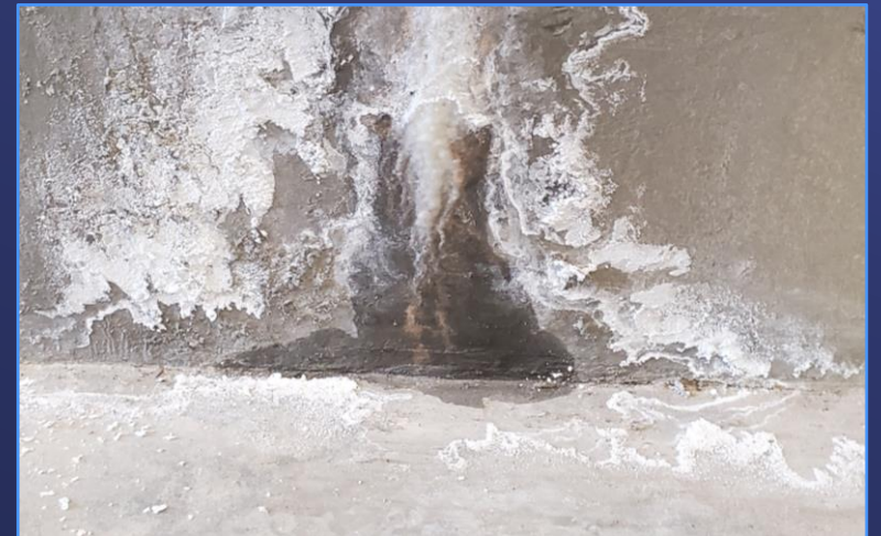
Close up of Leak on Contactor 1
