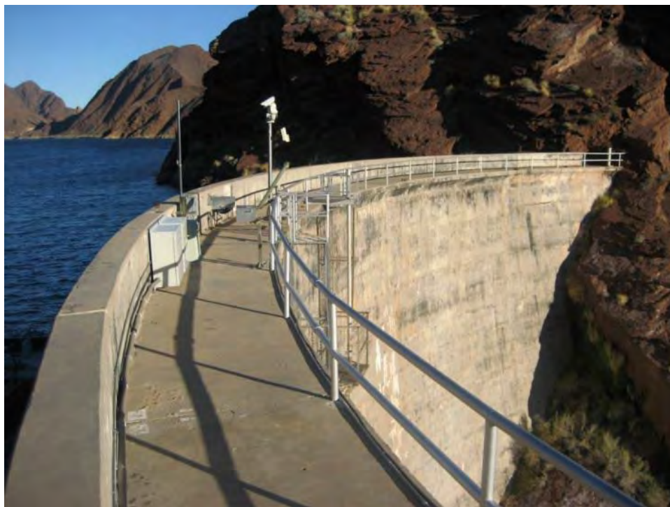
Figure 14. Pedestrian deck and handrail on the crest of Copper Basin Dam, looking northeast. Source: Metropolitan
