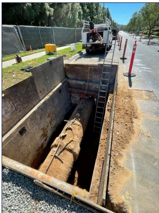
Excavation and shoring completed in preparation for pipe access cutout at one of the Orange County Feeder Relining sites
