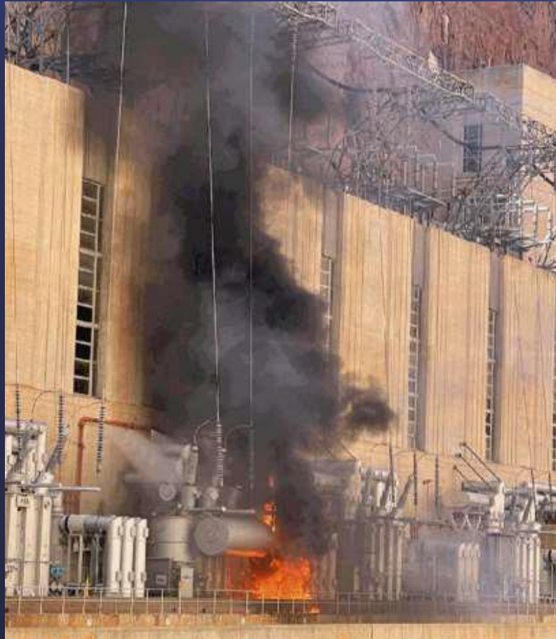
Transformer fire due to 230kV bushing failure
