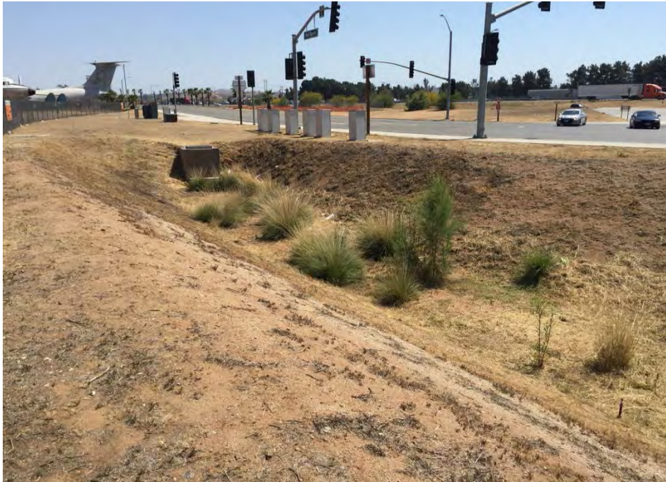
Photograph 1. Existing earthen dirt storm channel along Van Buren Boulevard just east of I-215 and north of the March Air Reserve Base, facing southwest.
