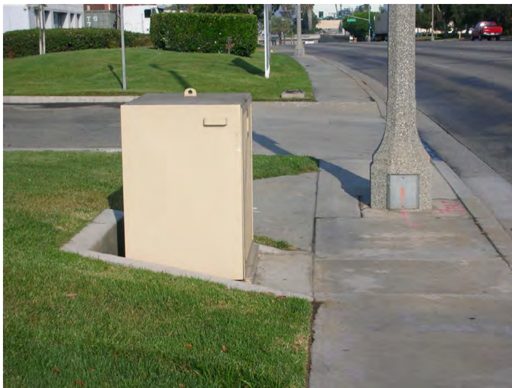
Figure 4. Typical Aboveground Valve Enclosure
