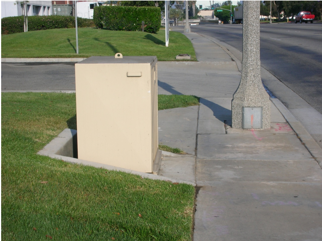
Figure 3-6. Typical Above-ground Valve Enclosure
