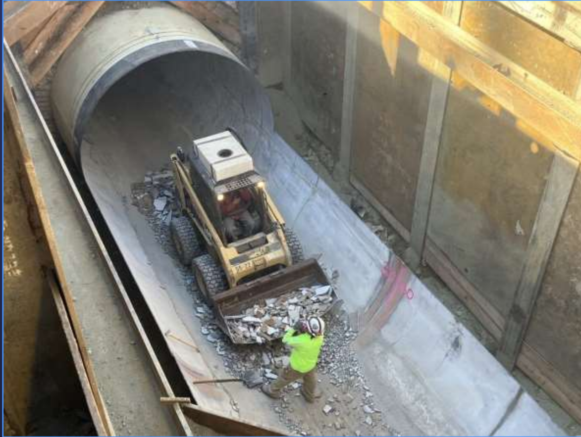
Removal of damaged cement mortar lining
