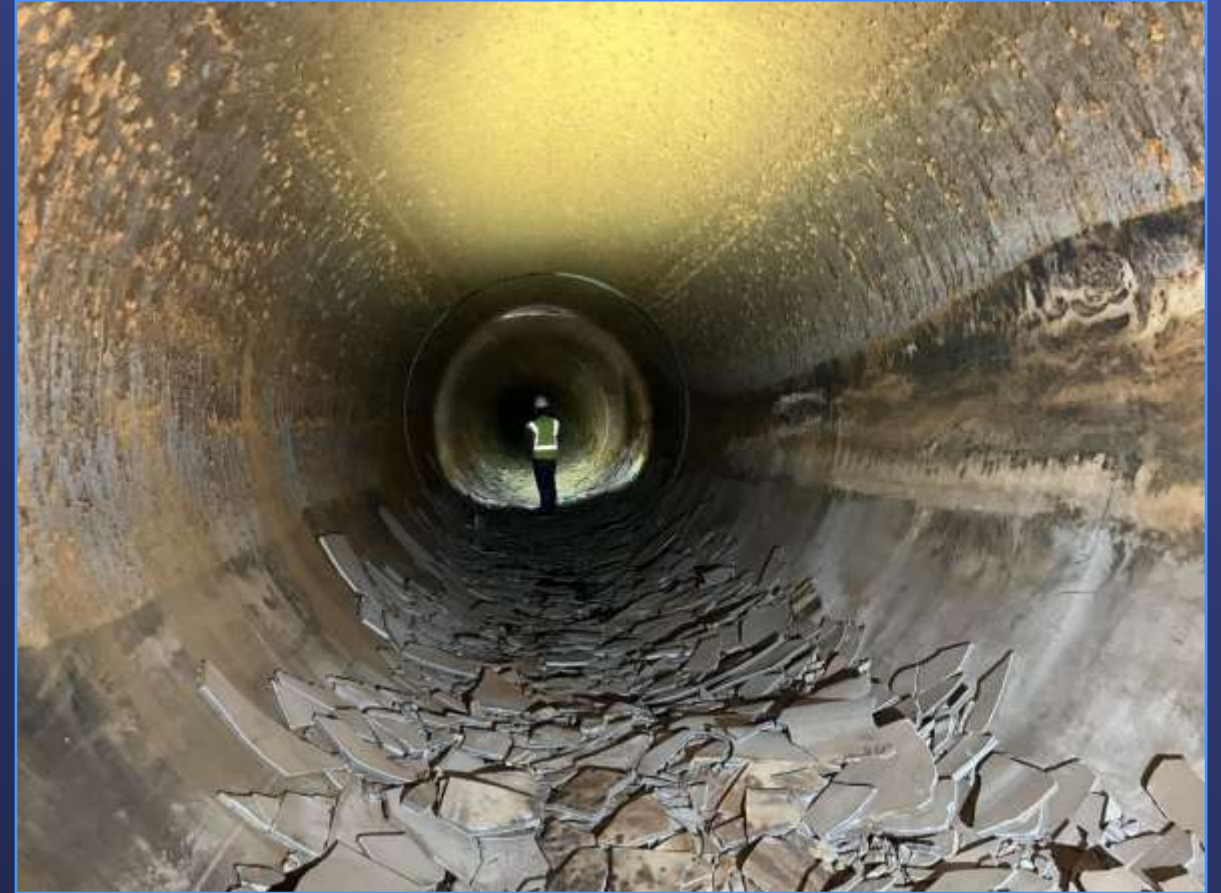
Removal of damaged cement mortar lining
