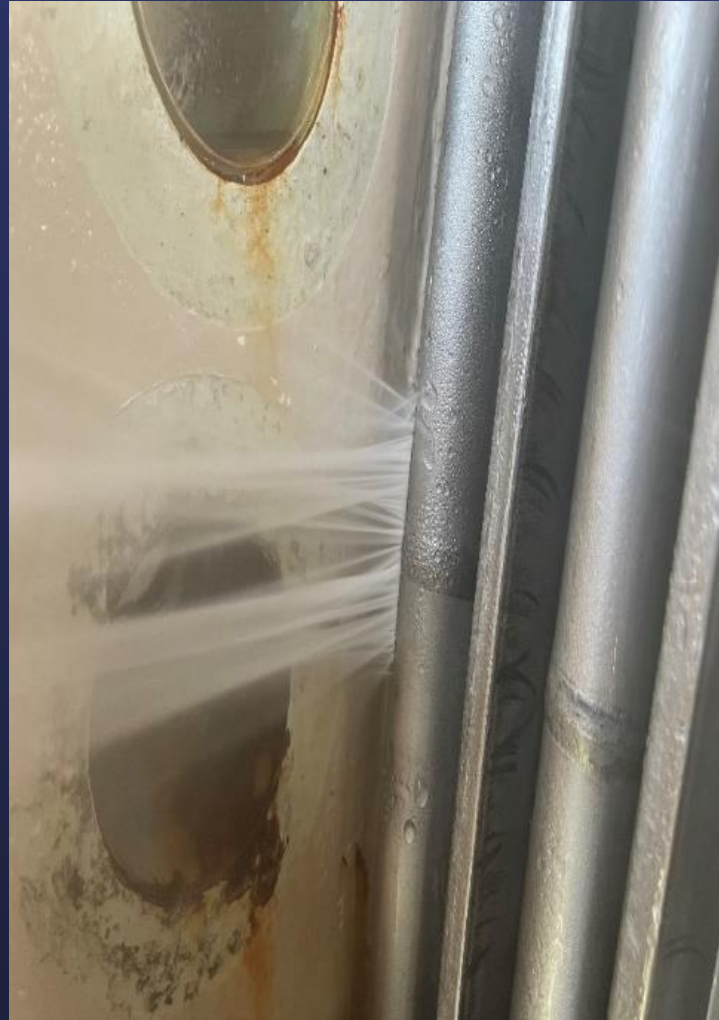
Initial leak on bellows joint
