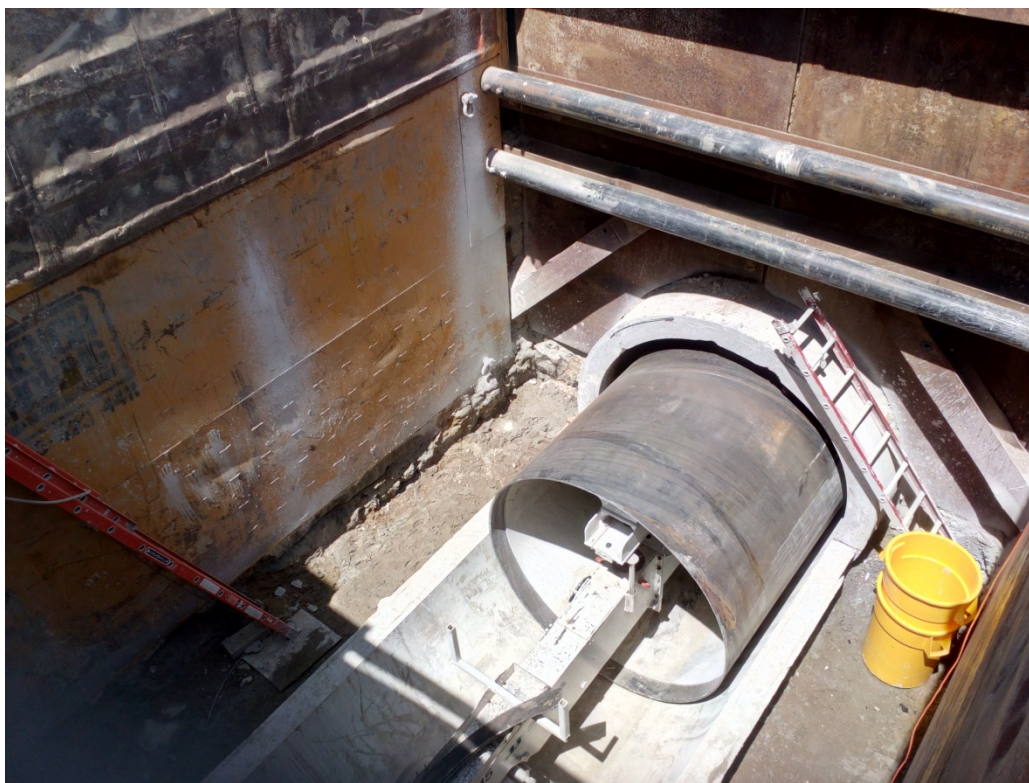
Figure 3-4. Steel Sliplining with Non-Collapsed Pipe in Progress
