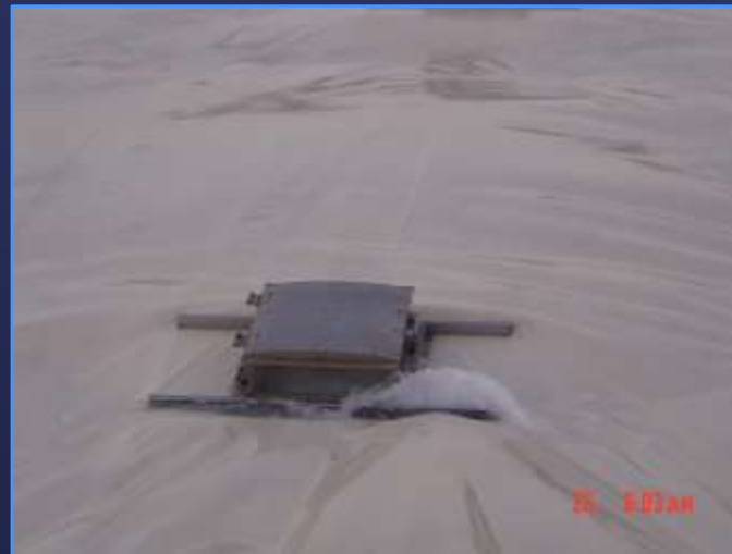
Cover tear releasing water
