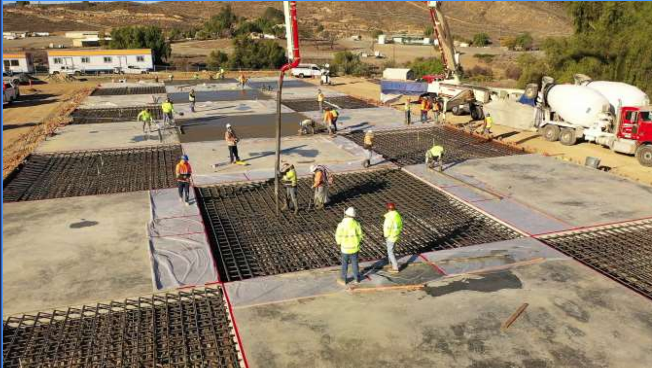
Checkerboard placement of concrete foundation slab
