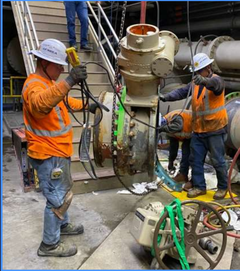
Removal of valves during ½-plant shutdown
