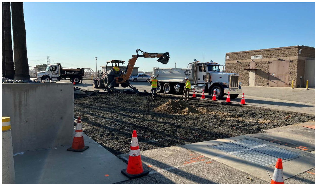
Contractor excavating equipment pad area at the Jensen plant
