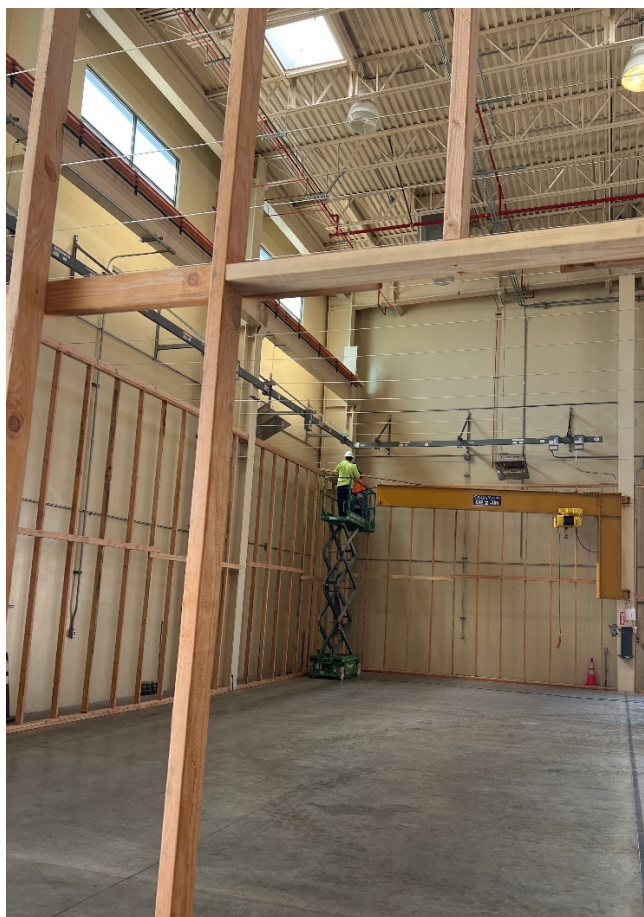
Construction of containment wall structure for vertical machine area
