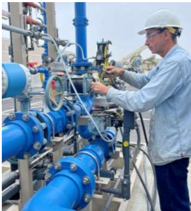
Staff repairing an air leak on tubing to an MBR valve actuator at the PWSC demonstration plant
