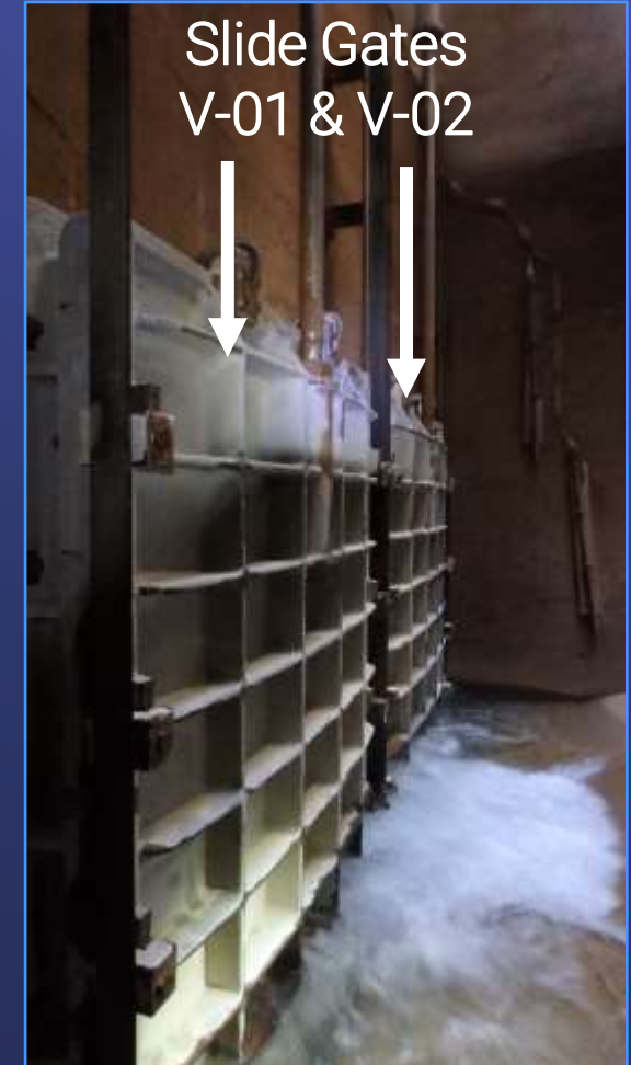
Leakage Past Closed Slide Gates
