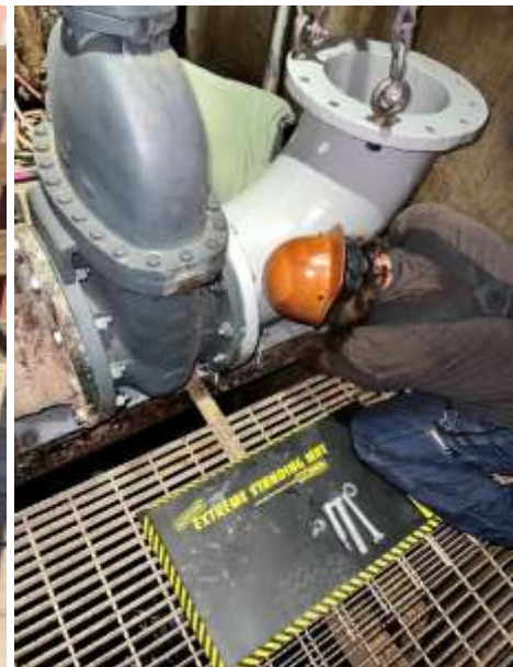
Before (left) and after (right) blasting and coating of circulating water pump components for Eagle Mountain pumping plant
