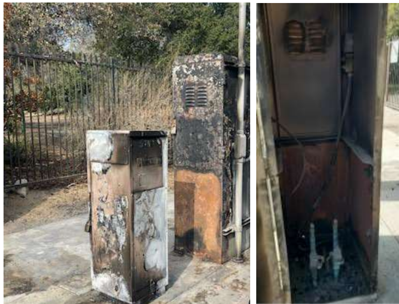
Fire damaged AMR cabinet at the LA-04 service connection
