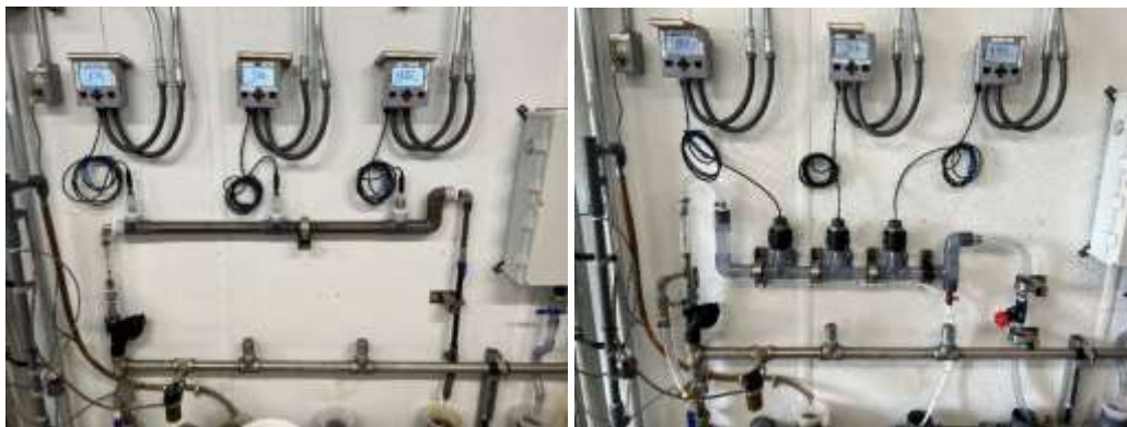
Previous (left) and modified (right) water quality probe manifold at the Jensen plant
