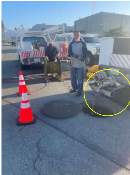
Staff using an electric cable puller at a deep vault at the Weymouth plant
