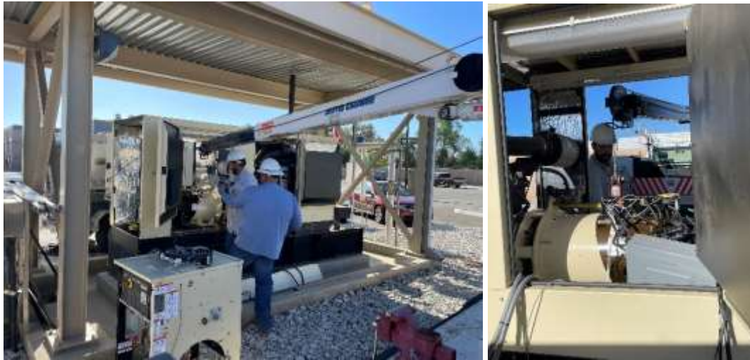
Staff installing the rebuilt generator at the Chemical Unloading Facility
