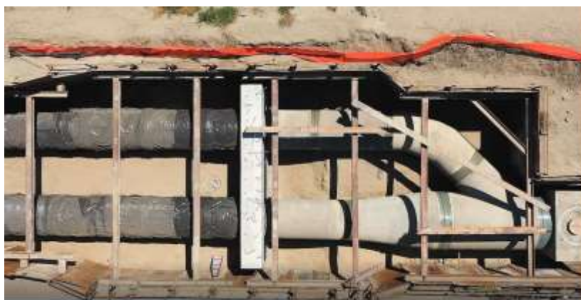
Casa Loma Siphon Seismic Upgrades—ERDIP and steel pipe transition at thrust block and wye
