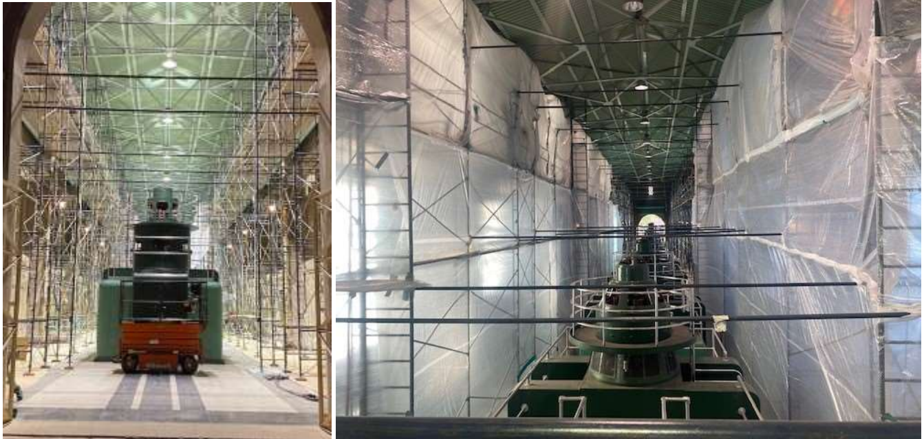
Overhead crane replacement at Gene pumping plant
