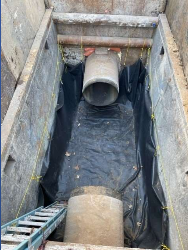
Pipe Access Pit – Pipe Section Removed
