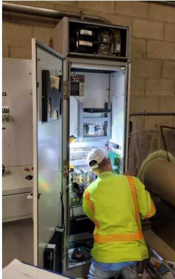
Staff troubleshooting an RTU at the OC-70 service connection
