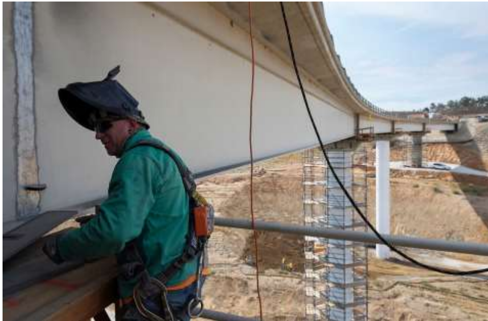
Worker prepares to use a tack welder at the tower bridge. Photo credit: California Department of Water Resources
