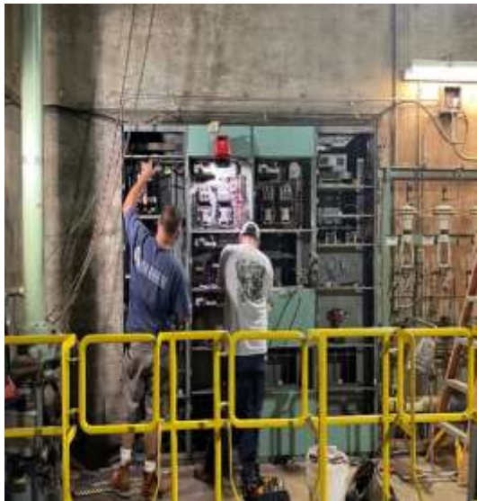
Staff isolating the MCC (left) and removing cables (right) for demolition at the San Gabriel PCS
