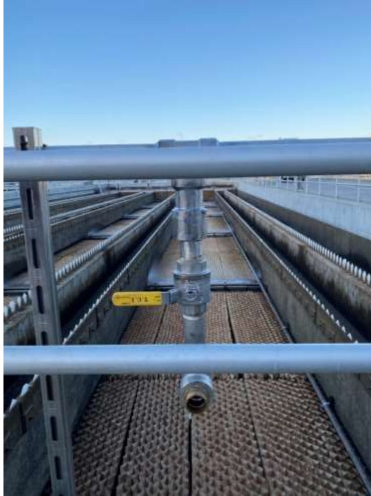
Stainless steel valve and hose connection installed at the Skinner washwater reclamation plant
