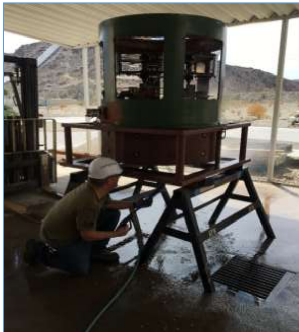
Staff cleaning a 12,500hp motor excitation housing at the Eagle Mountain pumping plant
