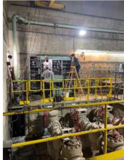
Staff isolating the MCC (left) and removing cables (right) for demolition at the San Gabriel PCS
