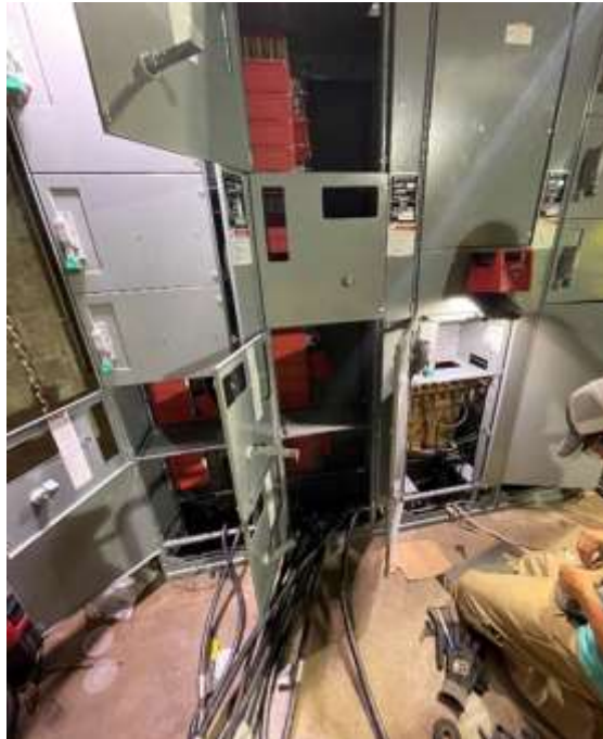
Staff installing new cables to the MCC at the San Gabriel PCS
