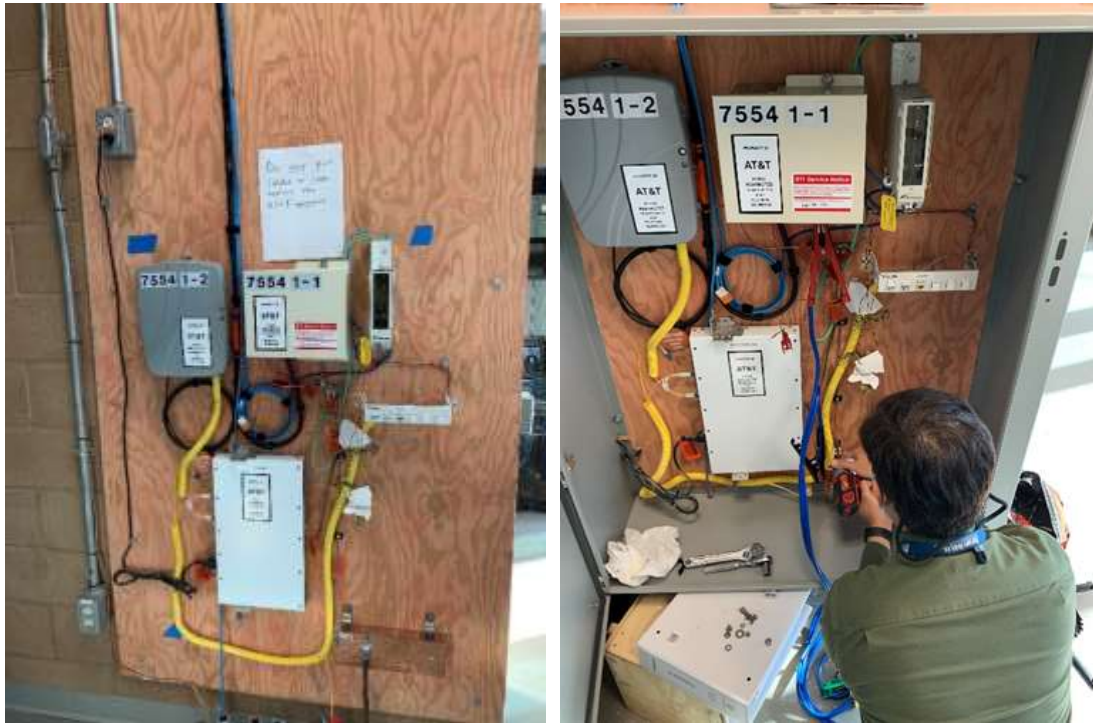
Telecommunication equipment before (left) and after (right) replacement at the Greg Avenue pump station
