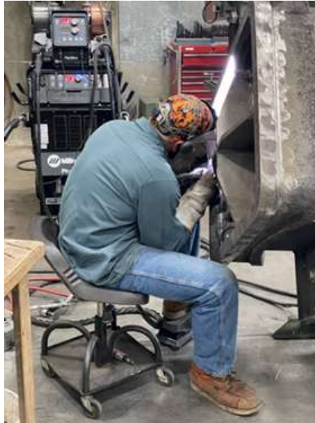
Staff welding new flange to the existing scroll case door for DWR's Gianelli facility
