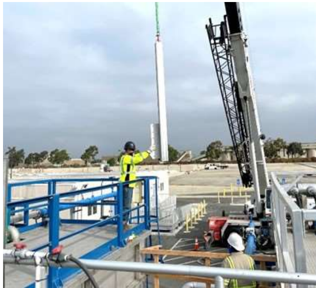
Staff assisting with lowering fall protection anchor posts to install onto the MBR tank at the demonstration facility
