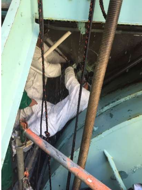
Staff installing new pipe on the Lower Feeder influent pipeline at the Diemer plant
