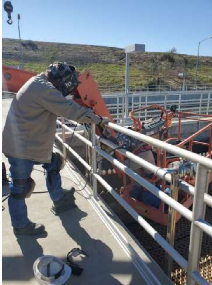
Staff welding and installing a valve from a manlift at the Skinner washwater reclamation plant
