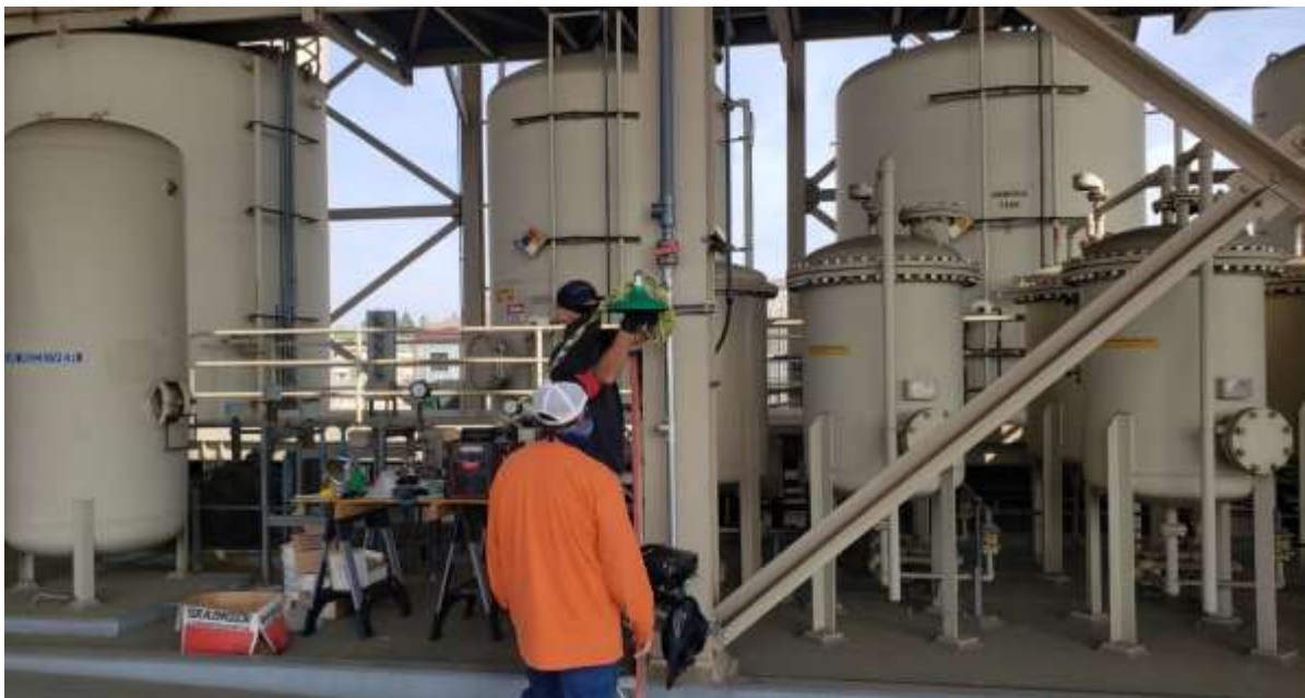
Staff installing additional safety showers in a chemical tank farm at the Weymouth plant
