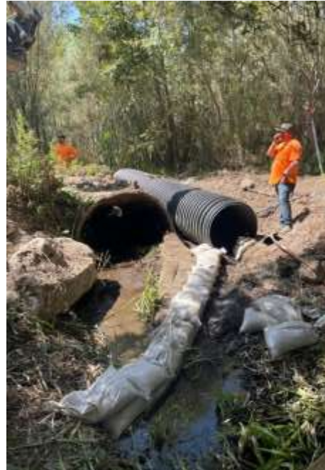
Removal of Culverts and Stream Restoration at Stickleback River Ranch, Mitigation Site for Impacts from the Foothill Feeder Inspections and Maintenance Programs
