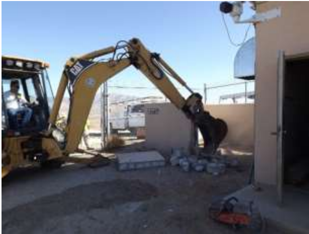
Staff demolishing a cinder block wall (left) and excavating (right) to install a new propane tank at the Cactus City communications site
