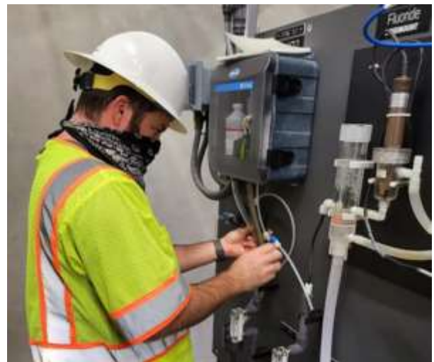
Instructor demonstrating maintenance procedures (left) and staff replicating these procedures (right) for performance testing at the new Water Quality Instrumentation Building at the Weymouth plant
