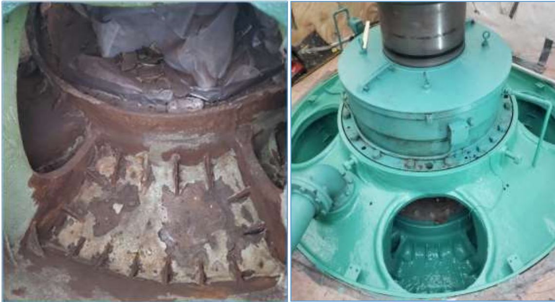
Before (left) and after (right) corrosion and coating repairs on the pump headcover at the Eagle Mountain pumping plant
