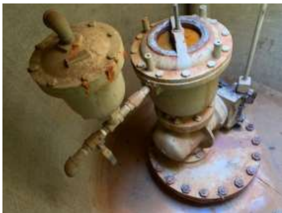
Rialto Pipeline air release vacuum valve assembly before (left) and after (right) coating work
