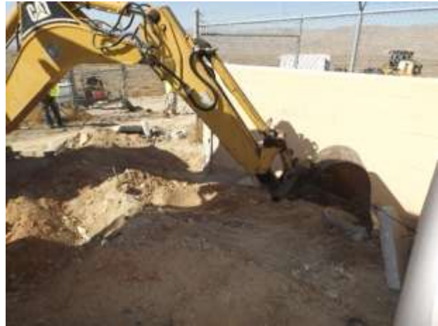
Staff demolishing a cinder block wall (left) and excavating (right) to install a new propane tank at the Cactus City communications site
