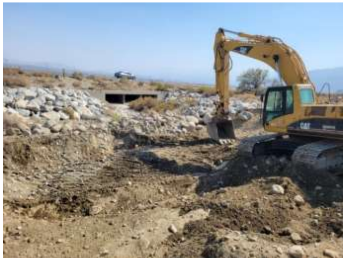
Staff shaping a drainage channel with an excavator along the CRA
