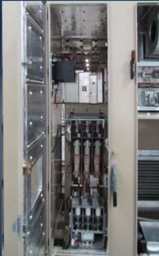
Disconnect Switch with Fuses
