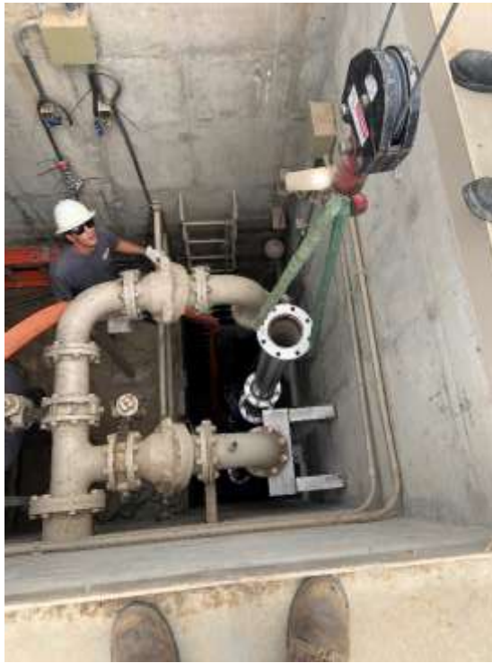
Staff installing a pump in underdrain structure on the Perris Bypass Pipeline
