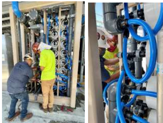
Reverse osmosis permeate piping being modified to improve access to equipment at the demonstration facility
