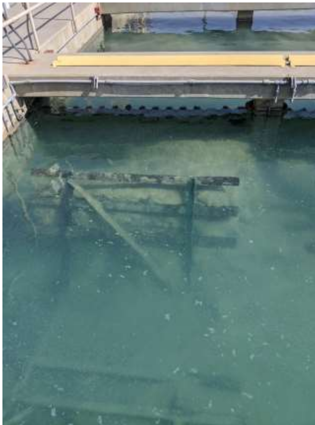
Filter media buildup on washwater reclamation plant flocculator at the Diemer plant
