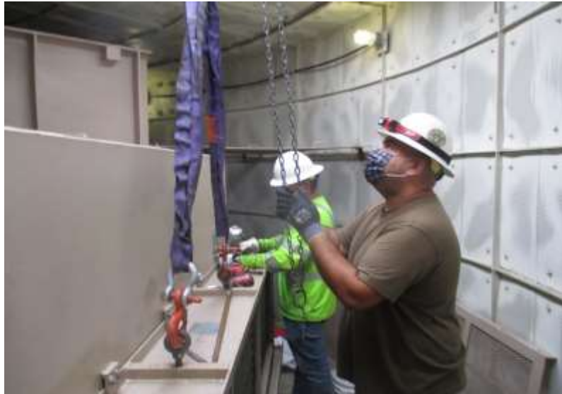
Staff removing air coolers with an overhead crane lift at Etiwanda HEP
