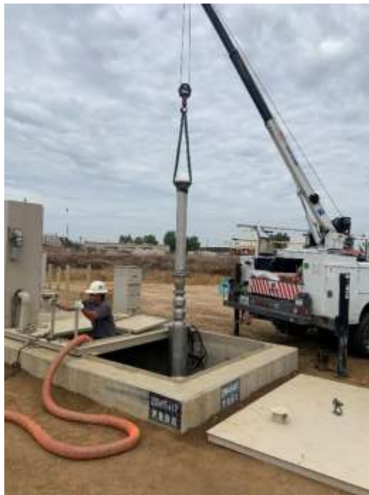
Staff replacing a pump in the underdrain structure on the Perris Bypass Pipeline
