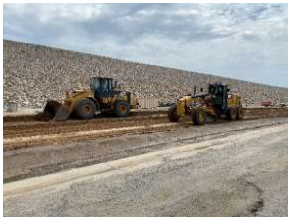
Motorgrader prepping subgrade (left) and receiving aggregate base material (right) at Lake Mathews
