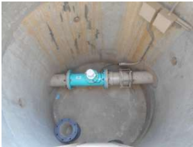
Perris Bypass Pipeline valve structure before coating
