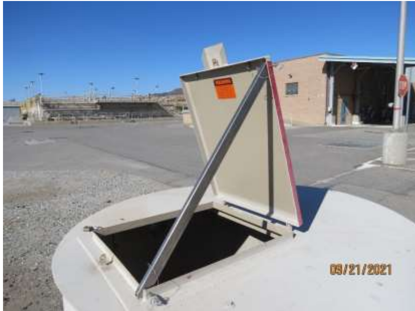
New propping rod for use on valve structure lids in the distribution system
