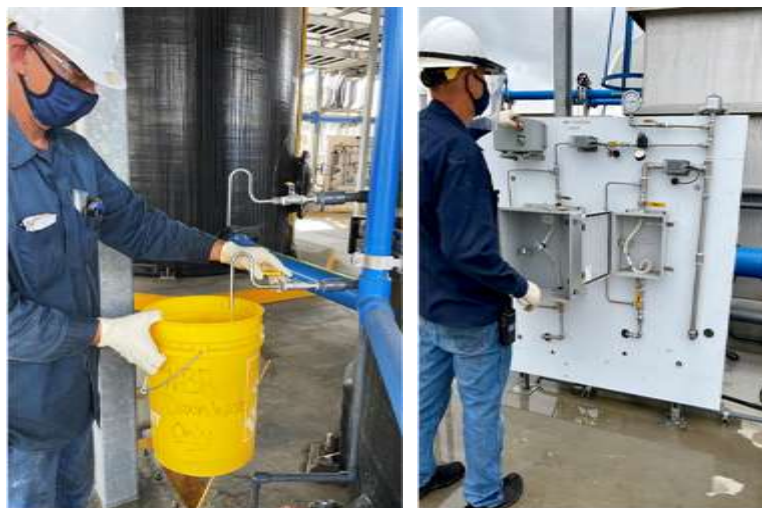
Staff flushing a new sample tap (left) and completing disinfection and flushing of the membrane bioreactor sampling skid (right) at the demonstration facility
