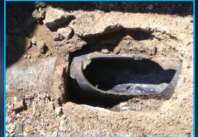
Damaged Wastewater Line
