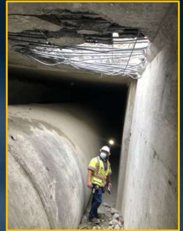
Upper Feeder beneath damaged protection structure
