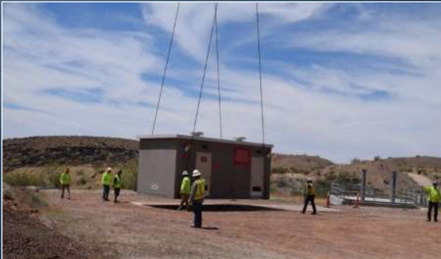
CRA Flow Meter Installation
