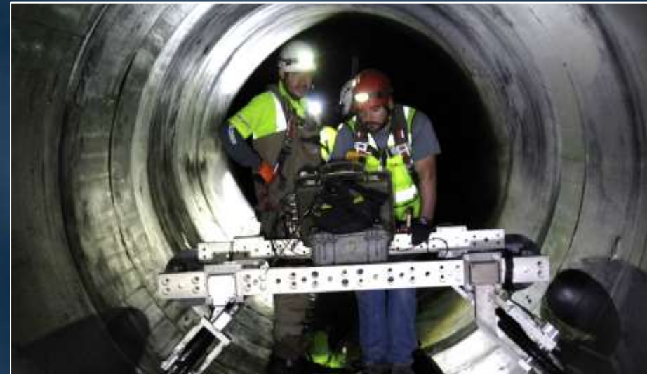
Sepulveda PCCP Inspection
