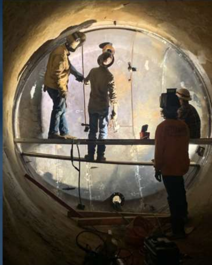
Welding of 133-inch bulkhead
