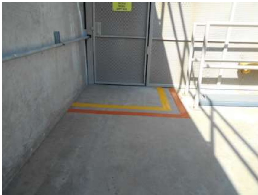
Recoated PSM lines for the chlorine process area at the Skinner plant
