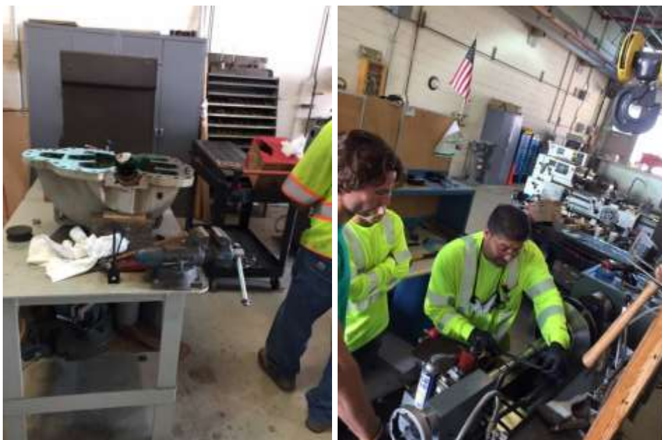
Dismantled pump case (left) and staff checking pump shaft tolerances (right) at the Diemer plant
