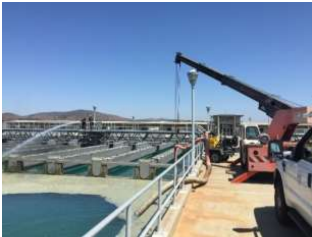
Staff removing material layer from a sedimentation basin (left) and dumping coal from the reclamation plant (right) at the Diemer plant
