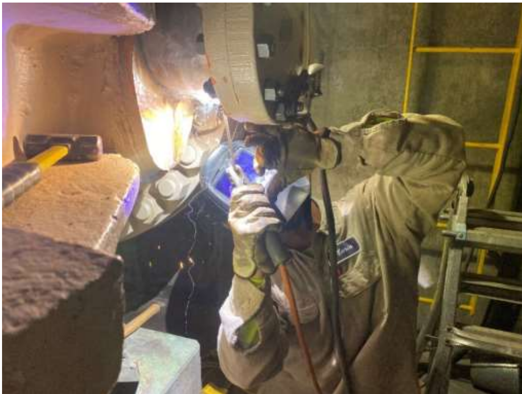
Staff welding a patch plate on the pipe at the Santiago Pressure Control Structure
