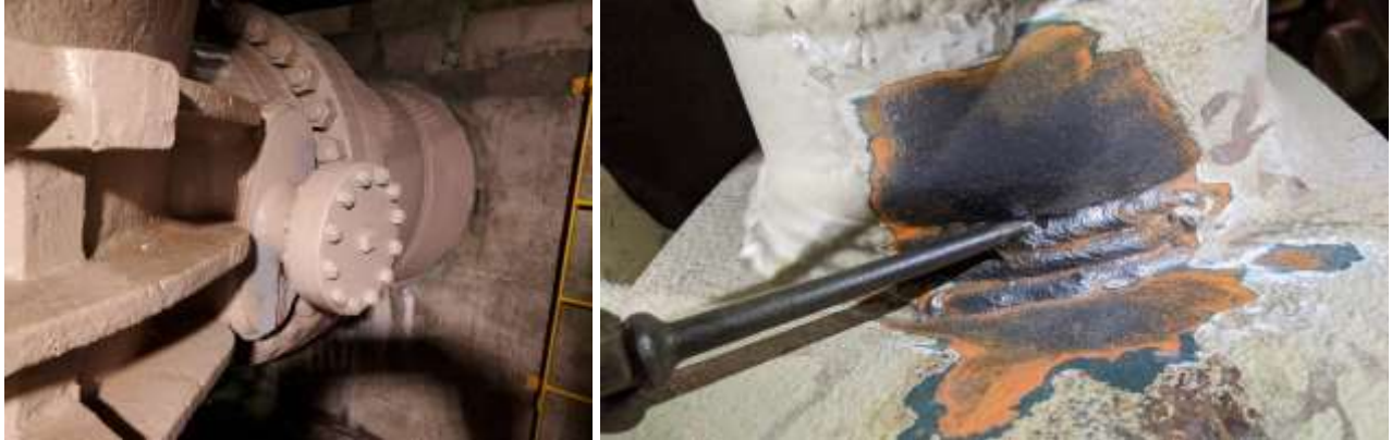
Pinhole leak at Santiago PCS on the East Orange County Feeder No. 2
