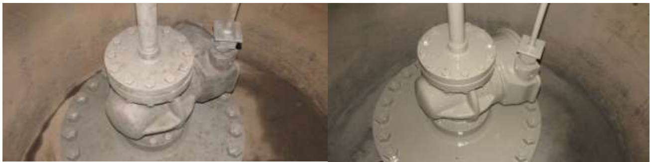
Sandblasted (left) and newly coated pump well valve (right) on the Allen-McColloch Pipeline
