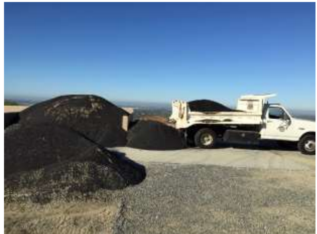
Staff removing material layer from a sedimentation basin (left) and dumping coal from the reclamation plant (right) at the Diemer plant
