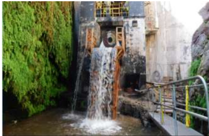
Gene Wash Reservoir Discharge Structure Rehabilitation—Draining the sluiceway to seat the isolation device
