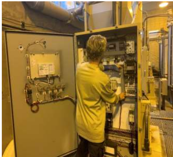
Staff installing the HMI display panel for the dry polymer mixer at the Skinner plant
