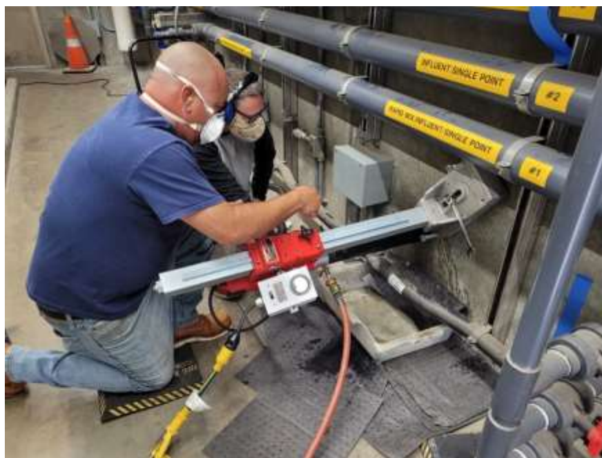
Staff core drilling at the Weymouth plant
