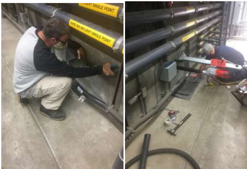
Staff verifying dimensions and locations (left) and preparing for initial core drill (right) at the Weymouth plant
