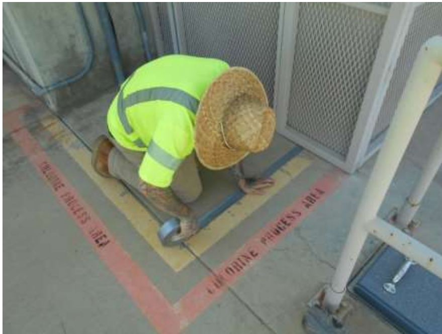
Staff preparing to recoat delineation markings for the chlorine process
