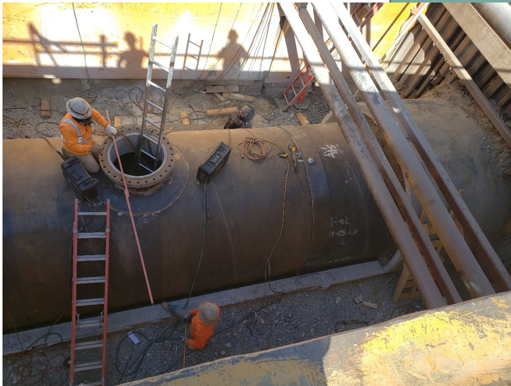
Closure piece with manway installation on Lake Perris Bypass Pipeline
