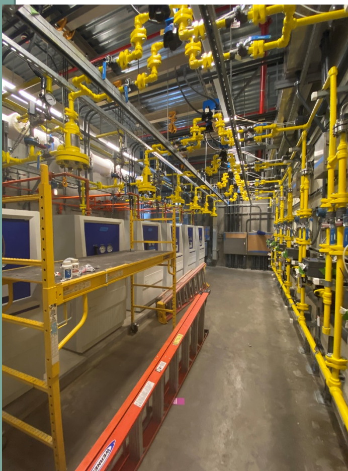
New evaporator and liquid chlorine piping at Weymouth Plant
