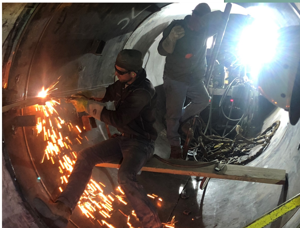
Pipe segment being welded on Allen-McColloch Pipeline
