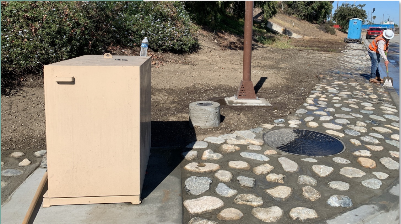
Completed manway restoration on Second Lower Feeder Reach 2
