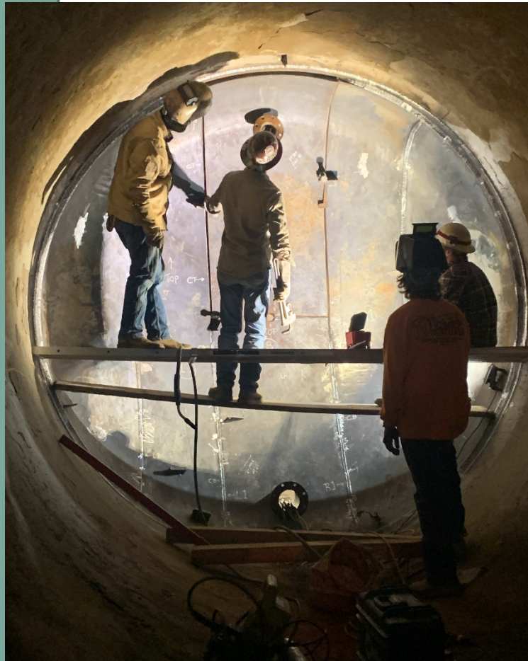
Welding of 133-inch bulkhead on Lakeview Pipeline
