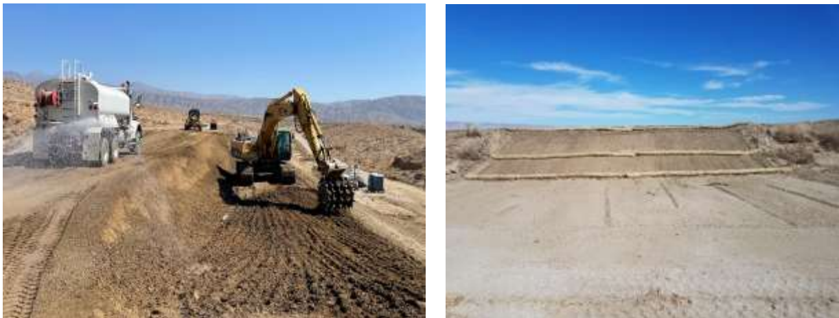
Staff placing and compacting fill materials (left) and completed berm repair (right) of San Andreas retention basin
