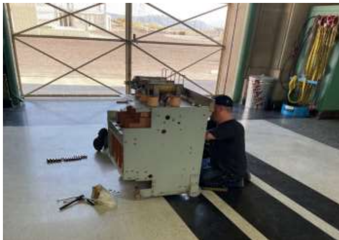
Staff performing preventative maintenance on a 2,300V circuit breaker at Eagle Mountain pumping plant
