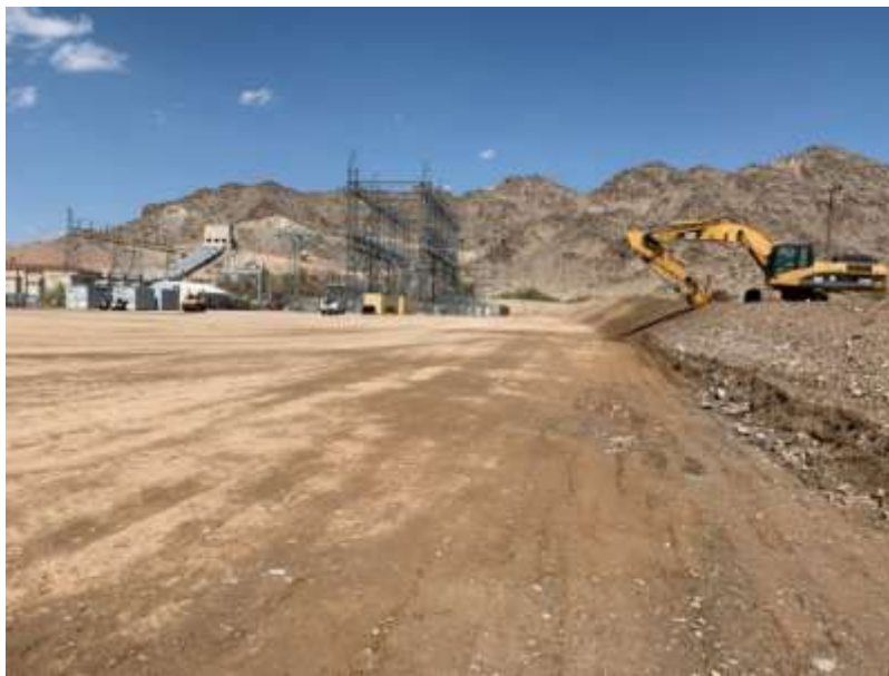
Staff using heavy equipment to create access and drainage improvements at Iron Mountain pumping plant
