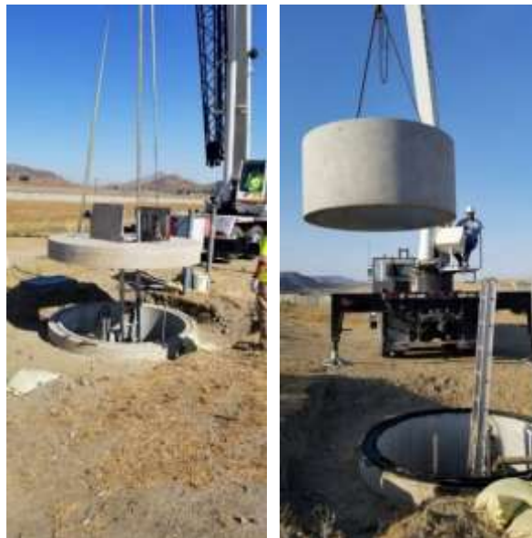
Staff replacing hatch for DVL Forebay underdrain structure to improve access and worker safety
