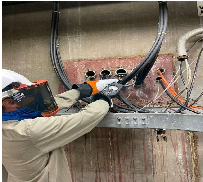
Staff locating a ground fault at the Mills plant
