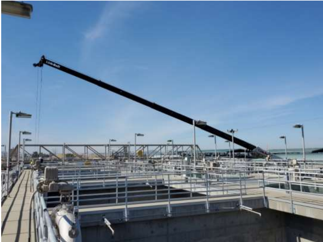
Crane extended to hold man basket for Module 7 surface wash header repair at the Skinner plant
