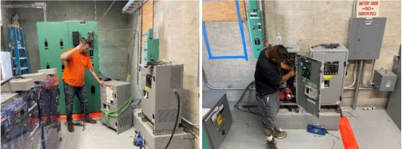
Staff placing new battery charger into position (left) and wiring new battery charger (right) at Hinds pumping plant
