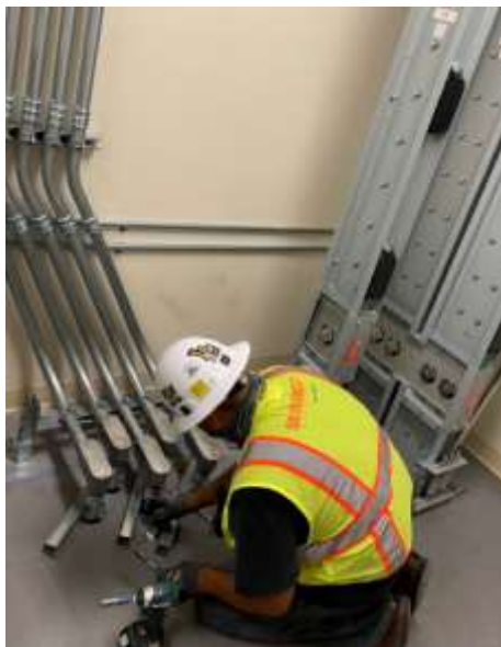
Headquarters Building Improvements—2 nd floor electrical conduit installation
