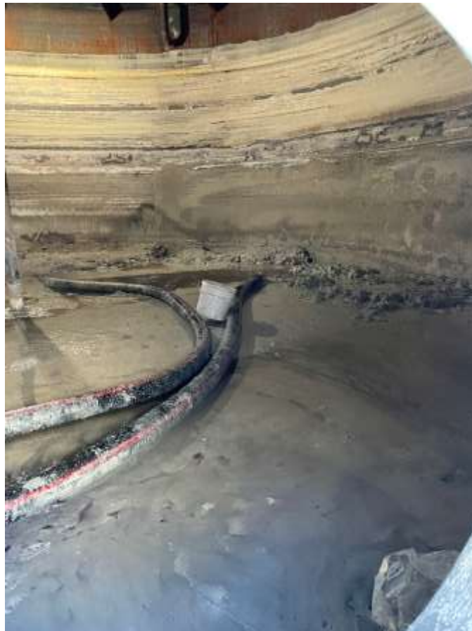
Sludge removal progress on 6-foot deep concrete-like sludge in a chemical tank at the Jensen plant
