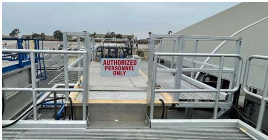
Safety handrail improvements providing ease of access to the MBR system equipment at the demonstration facility
