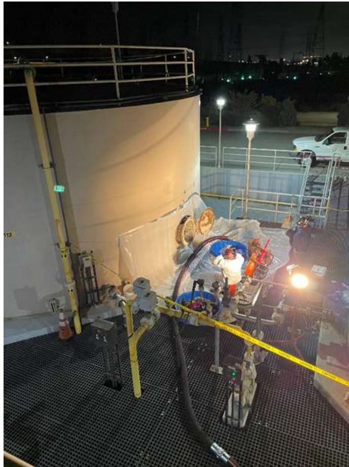
Hazardous waste vendor working in the decontamination zone to clean a chemical tank at the Jensen plant
