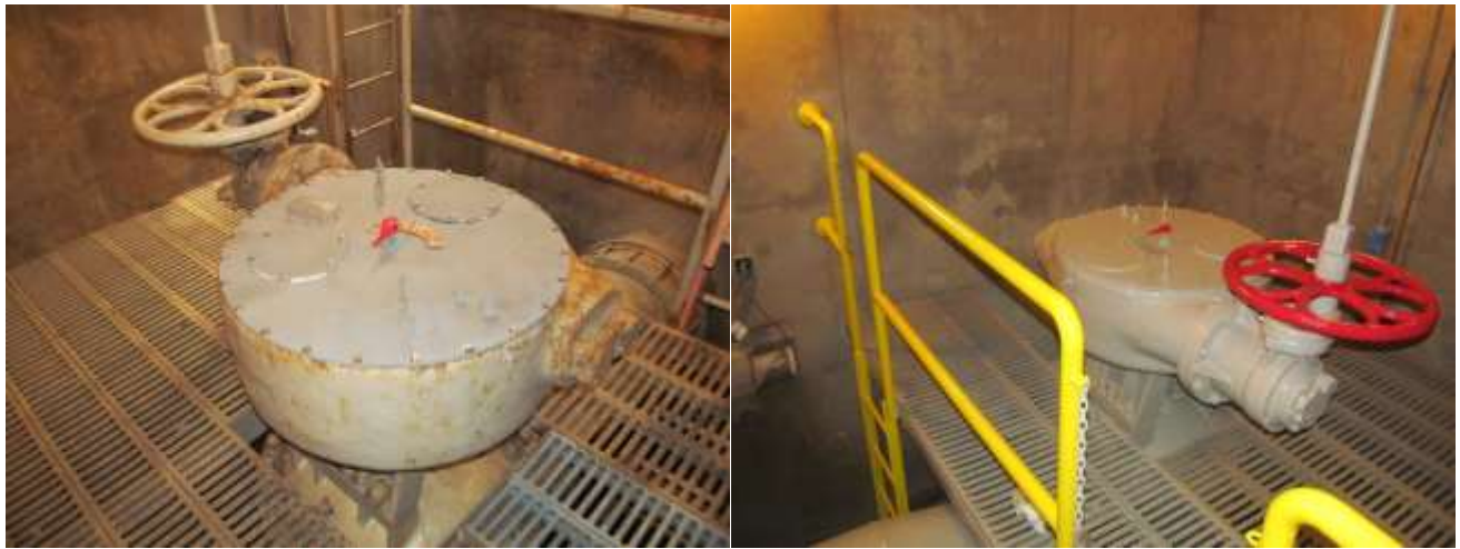
Turnout valve before (left) and after (right) coating at the OC-39 service connection on the East Orange County Feeder No. 2
