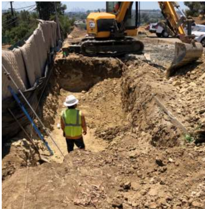
Garvey Reservoir Erosion Improvements Areas 6, 7, 8, 10, and 11—Excavation for Area 7 retaining wall
