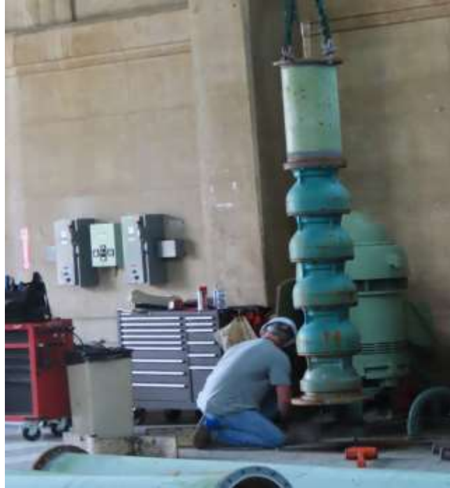
Staff removing a vertical turbine pump for repair at Hinds pumping plant
