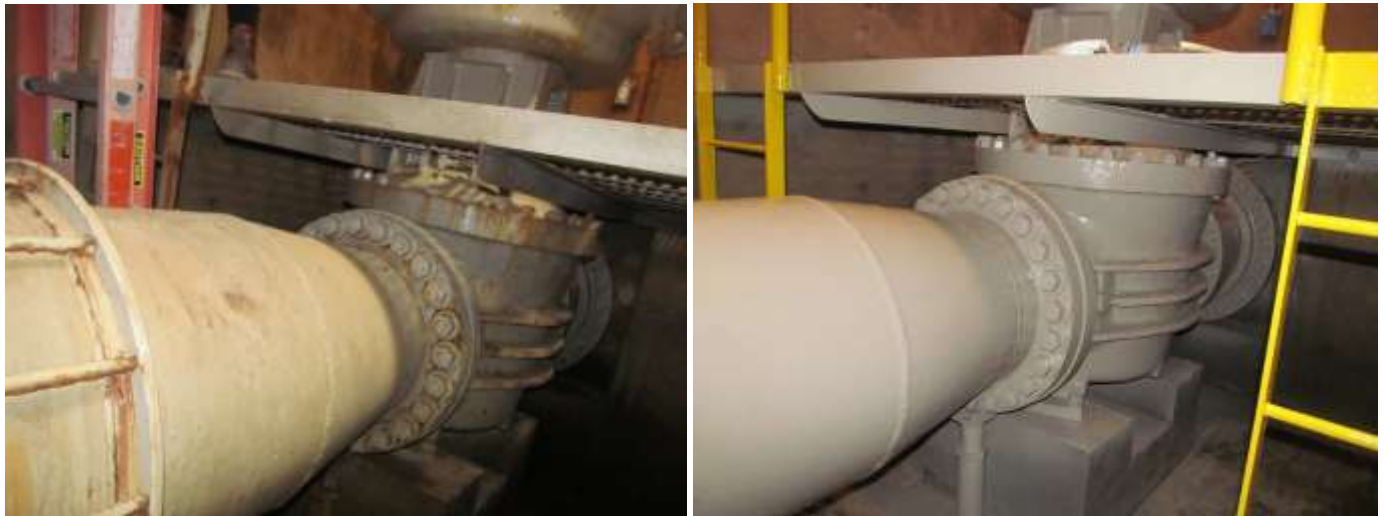
Meter piping before (left) and after (right) coating at the OC-39 service connection on the East Orange County Feeder No. 2
