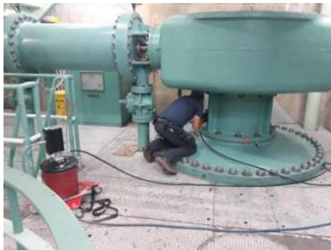
Staff lubricating the pump discharge valve at Eagle Mountain pumping plant
