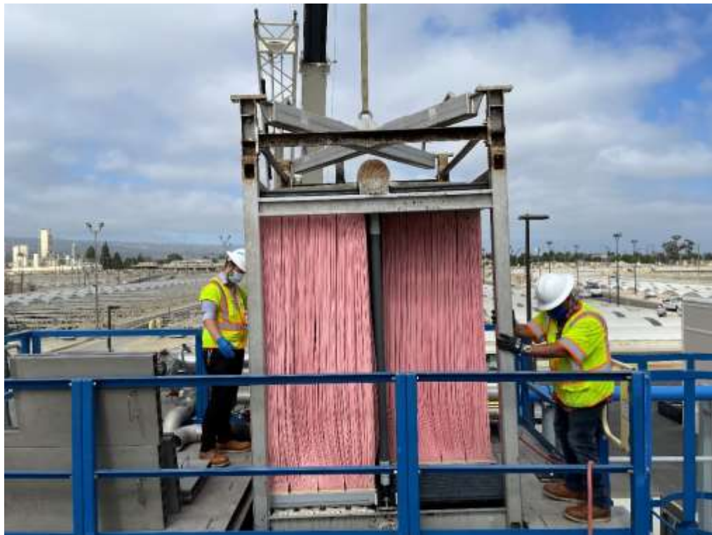
Staff remove a membrane cassette for additional fiber cutting at the demonstration facility
