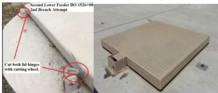
Old substructure lids were vulnerable to cutting at the hinges. New reinforced lids have no exposed hardware.
