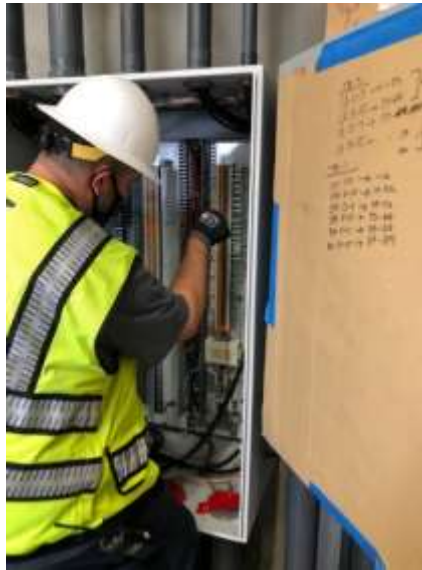
Staff connecting signaling cables from the RTU to the field terminals at the new water quality instrumentation building at the Weymouth plant
