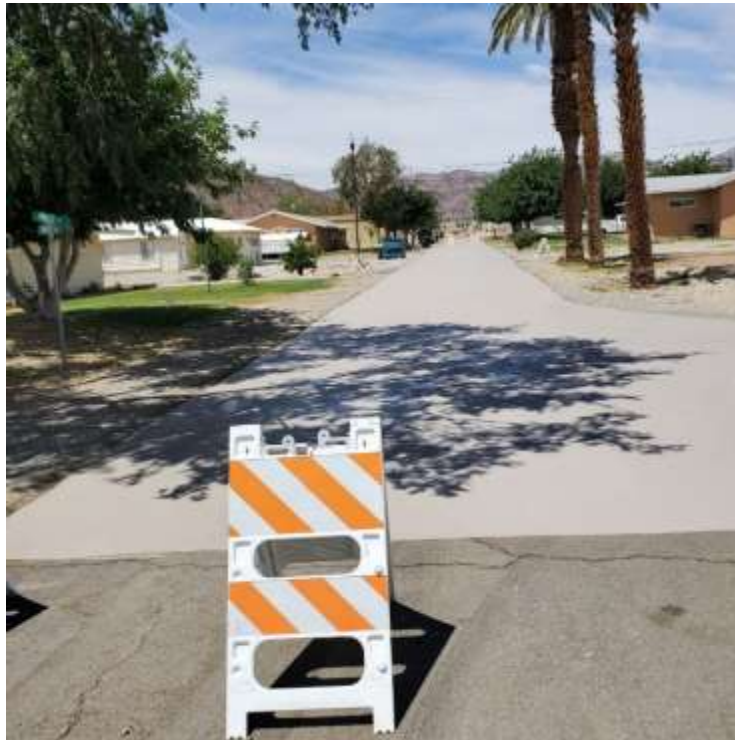
“Cool-Seal”-covered road at Eagle Mountain pumping plant
