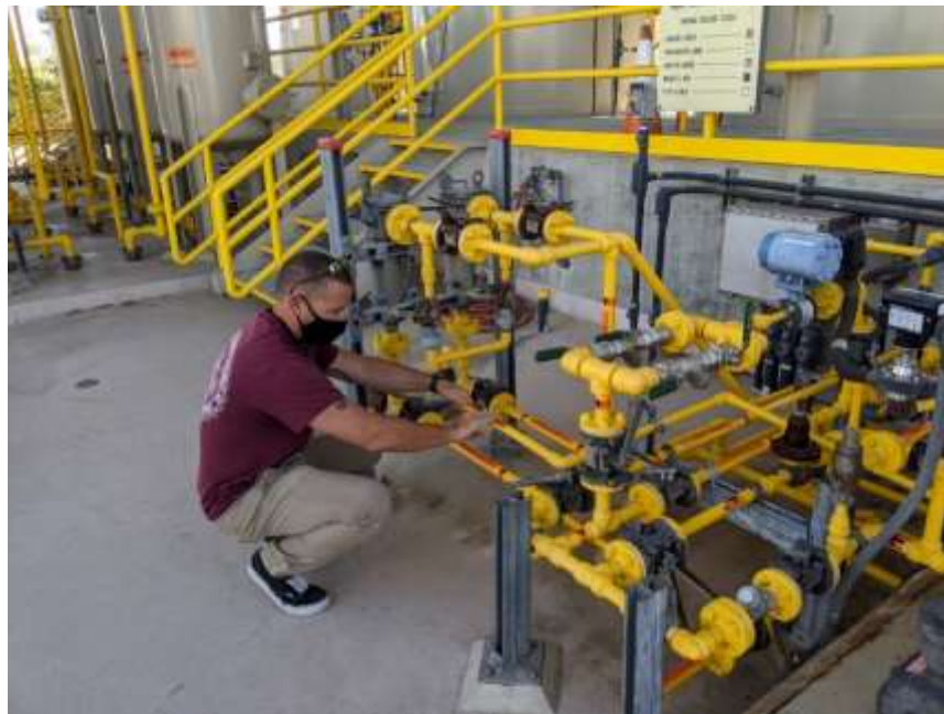
Staff installing new piping labels at a chemical tank farm
