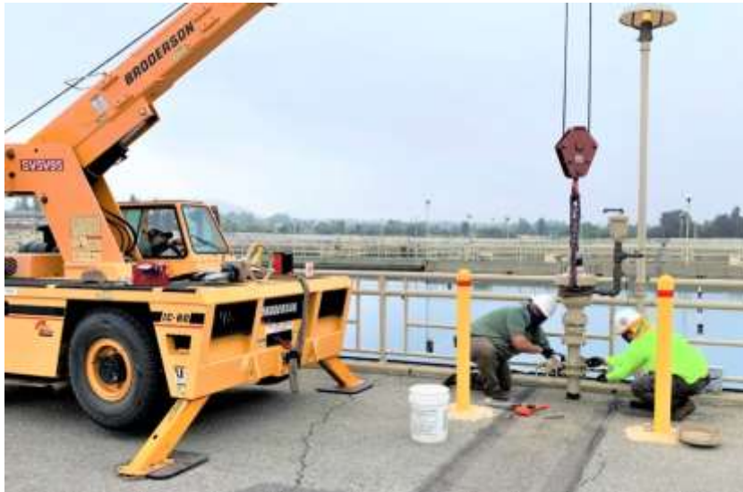
Staff removing an inoperable valve from the domestic water system at the Weymouth plant
