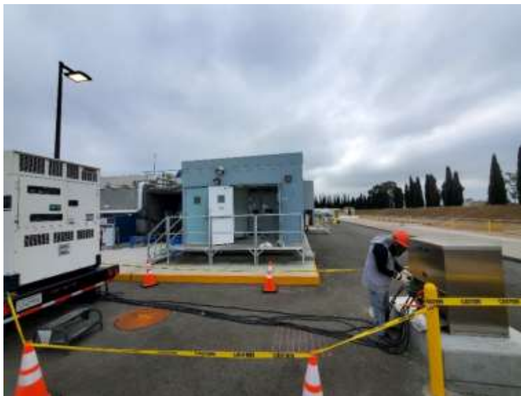
Staff verifying correct voltage and rotation at the generator power inlet at the RRWAPC
