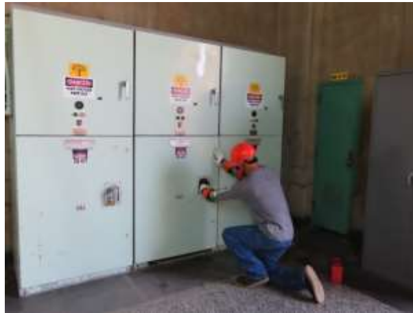
Staff securing a 2,300V circulating water pump at Hinds pumping plant
