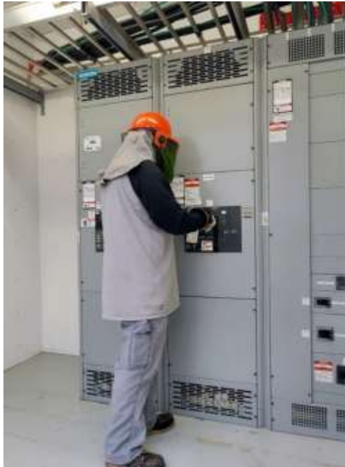
Staff applying locks and tags at an electrical breaker (left) and staff adjusting generator voltage (right) at the RRWAPC
