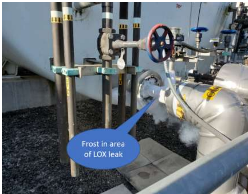
LOX leak with insulation removed at the Skinner plant
