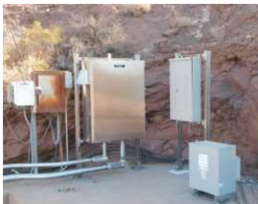
Gene Wash Reservoir Discharge Structure Rehabilitation —New control panel at the crest of the dam
