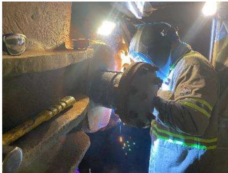
Staff welding patch plate inside the sectionalizing valve structure of the East Valley Feeder
