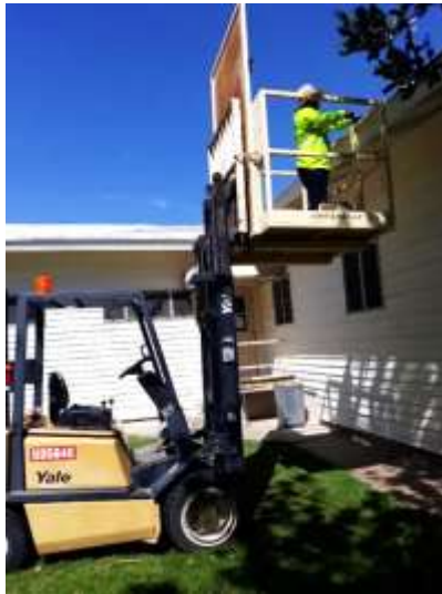
Staff applying a coating to the recreation hall roof at Eagle Mountain pumping plant
