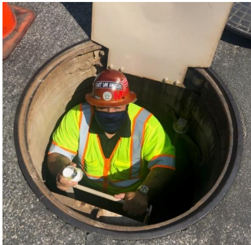
Engineer Victor Galvez working a pipeline shutdown
