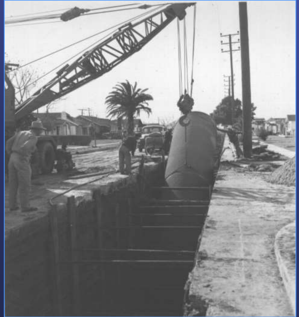
Middle Cross Feeder Construction - 1955
