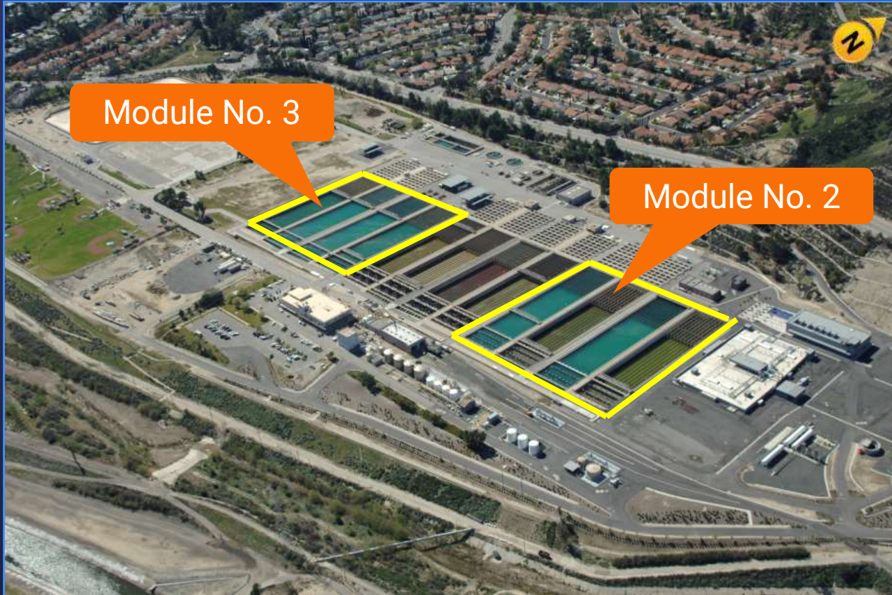
Jensen Modules 2 & 3 Sedimentation Basins
