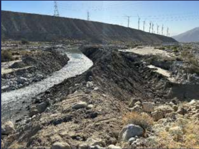
Whitewater Channel Repair
