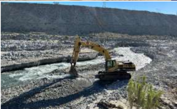
Whitewater River Repairs
