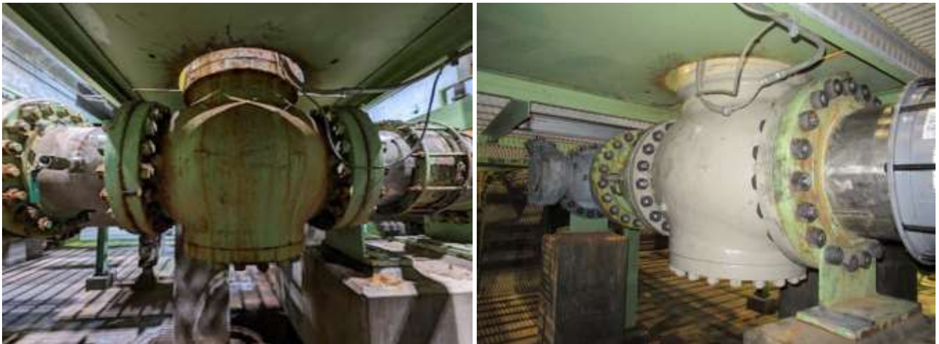
Leaking globe valve before (left) and after (right) refurbishment at Oak Street PCS
