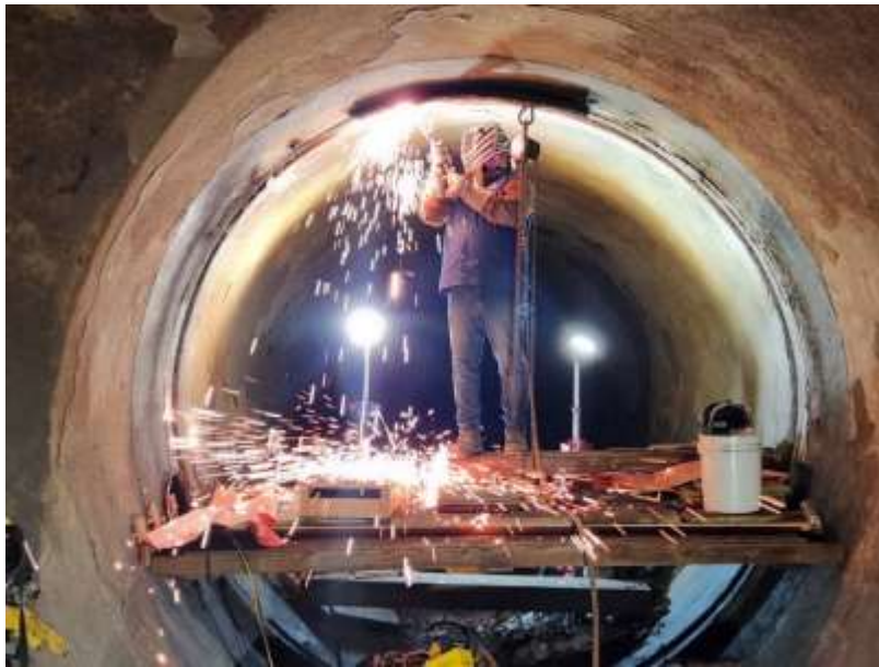
Staff torch cutting the remaining pieces of the large bulkhead installed at Perris PCS
