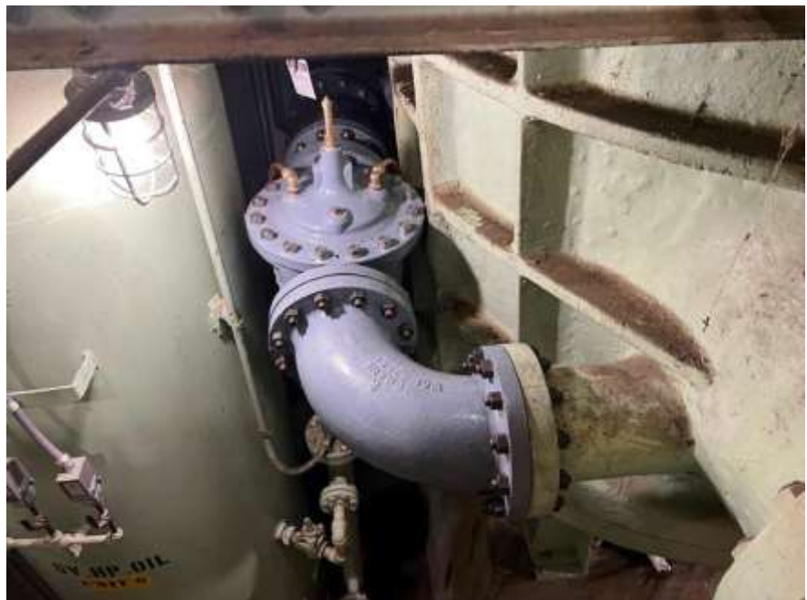
Staff installing rebuilt discharge valve bypass system components at a Desert facility
