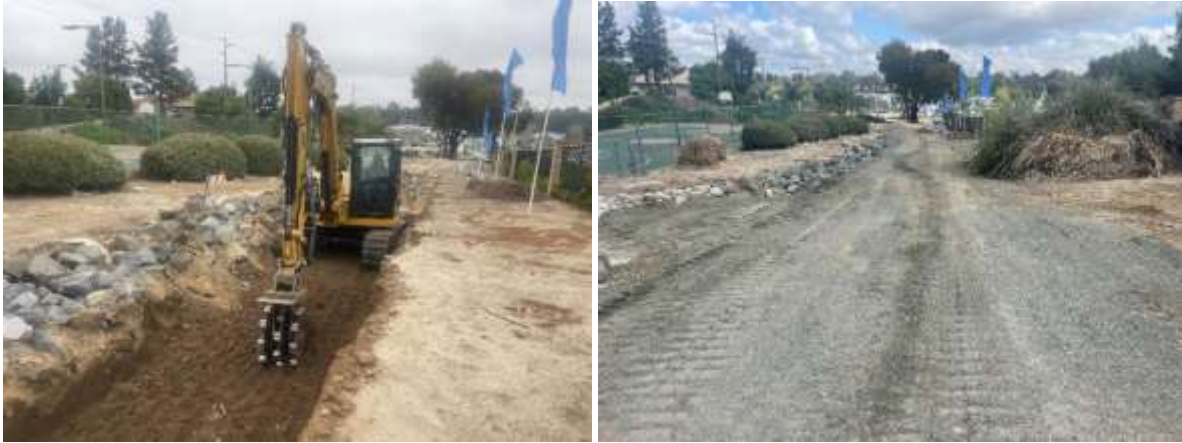
Staff using an excavator to compact fill material (left) and a completed section of road (right) along San Diego pipelines
