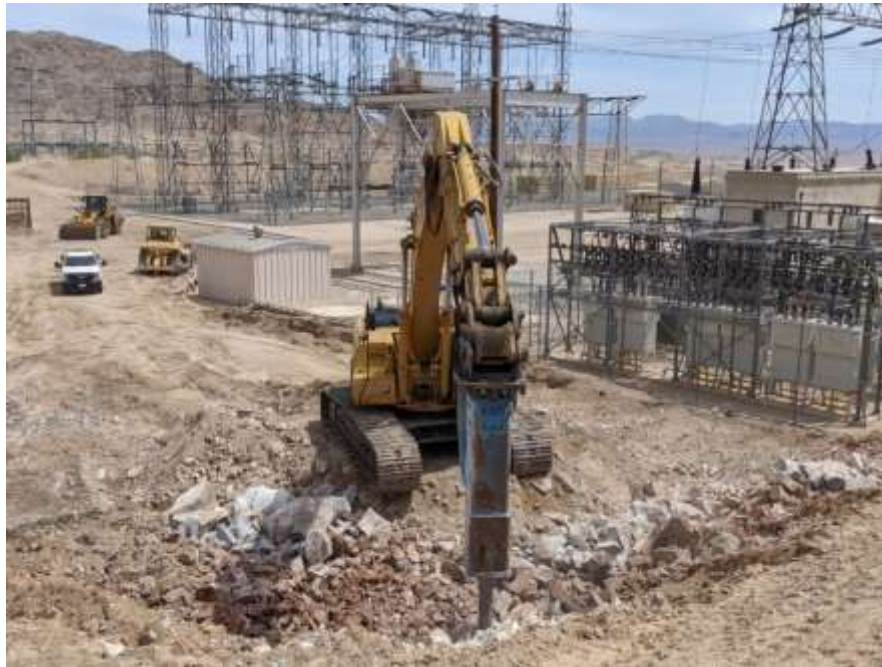
Staff hammering through rock and excavating at Iron Mountain pumping plant for the switch rack rehabilitation project
