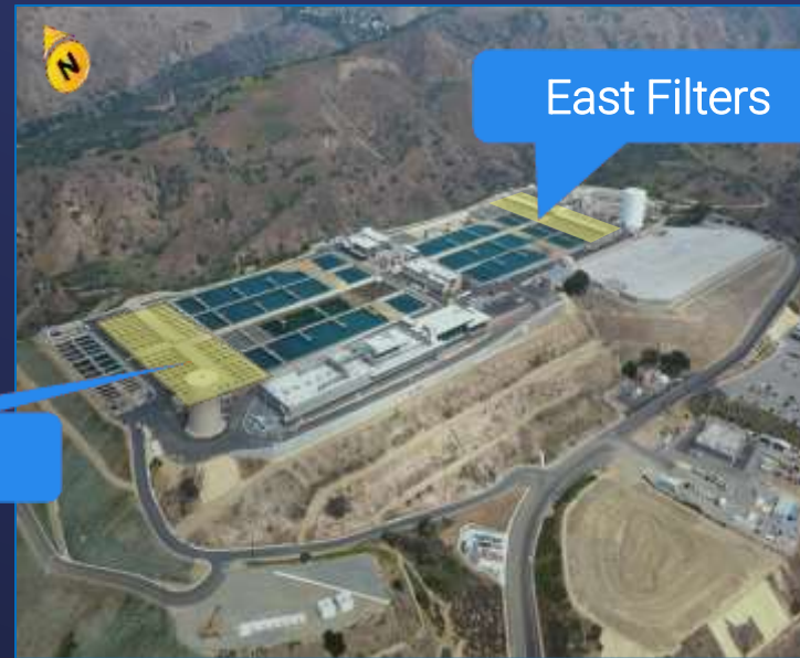
Diemer filter valve replacement
