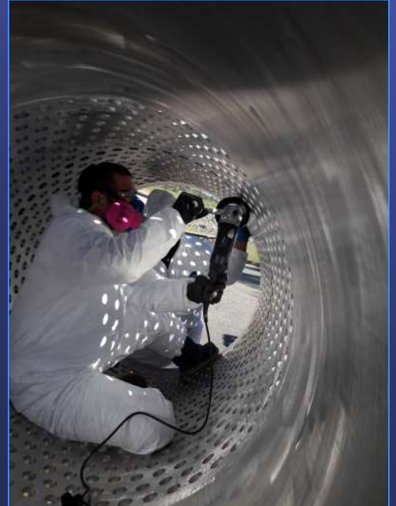
Inside Sleeve Valve Repair
