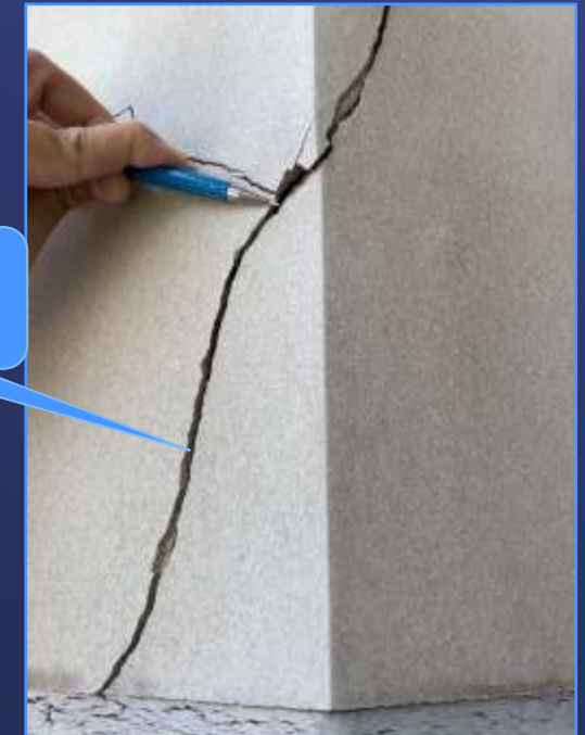
Crack at Column
