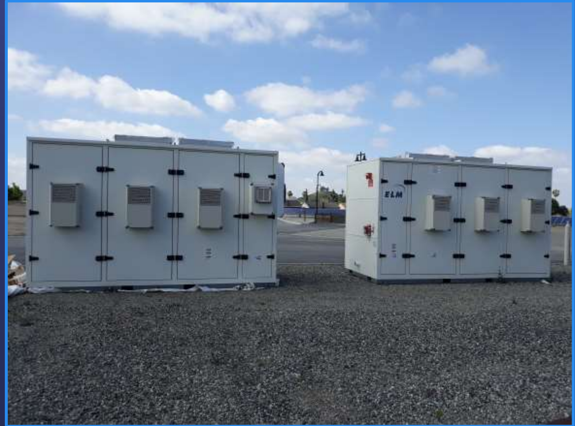
Battery Cabinets at Weymouth Plant
