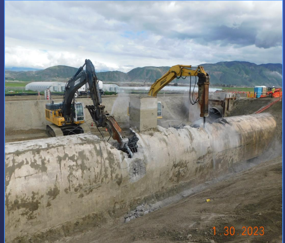
Demolition of existing siphon at tie-in location
