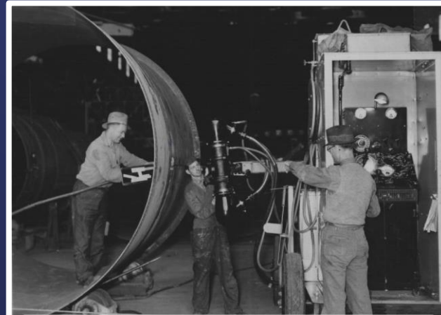
X-Ray machine testing integrity of welds on the steel pipe of Upper Feeder (1936)
