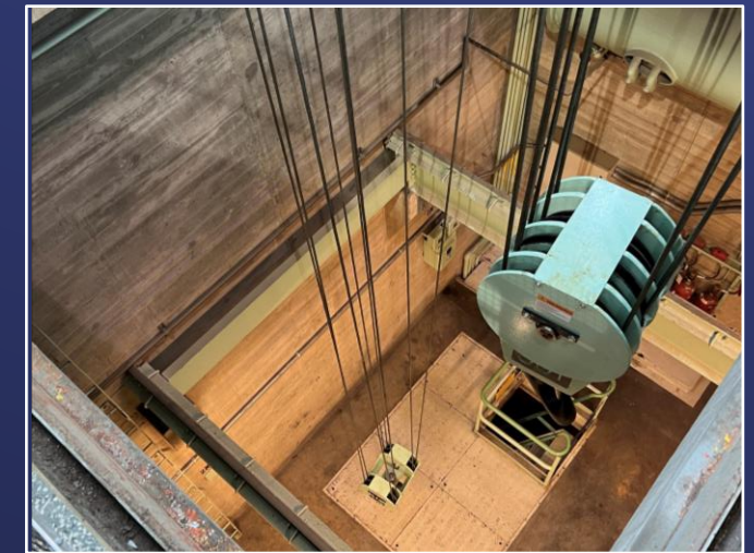
Hoists Below Motor Room Floor
