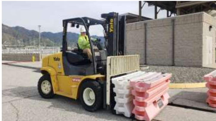
Staff installing traffic control barriers to protect the temporary solids handling pipeline
