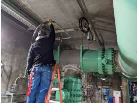
Staff preparing for repairs of the backwash header at the Diemer plant
