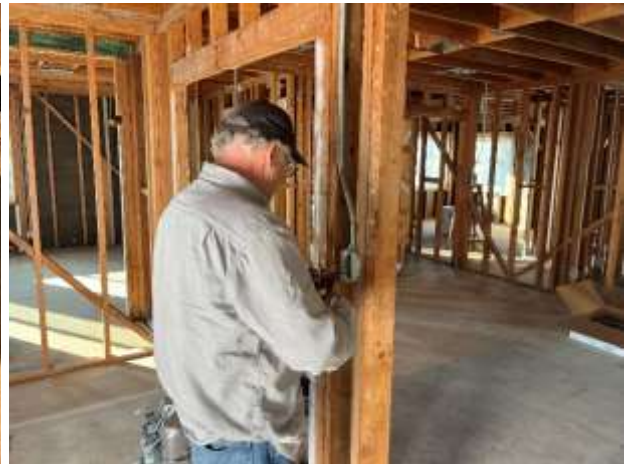
Staff installing recessed can lighting (left) and wiring a new light switch (right)
