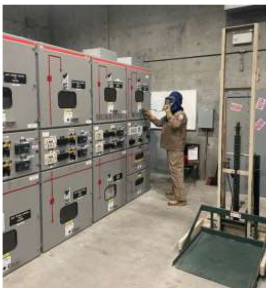
Staff performing high-voltage switching to accommodate arc flash data gathering at the Skinner plant
