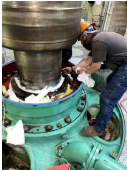
Staff replacing an RTD on a pump bearing at Eagle Mountain pumping plant
