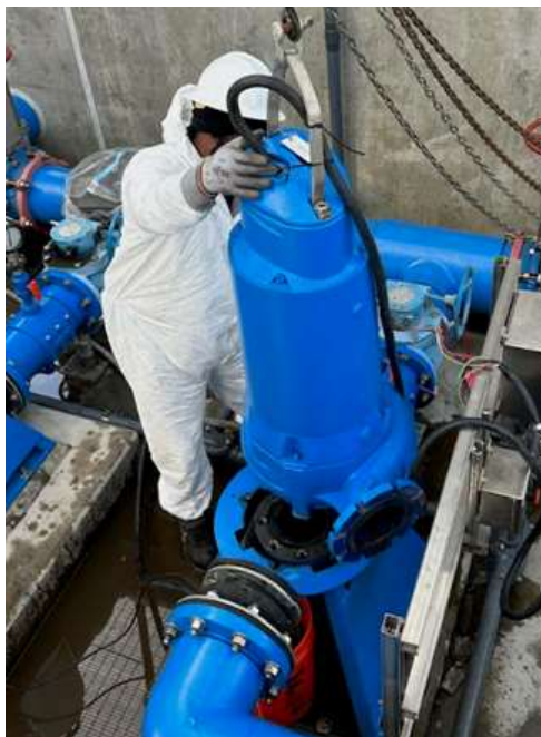
Staff installing a replacement return activated sludge pump at the PWSC demonstration plant
