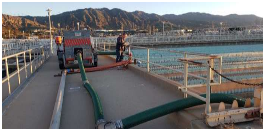
Staff reviewing installation of a temporary solids handling pipeline at the Jensen plant
