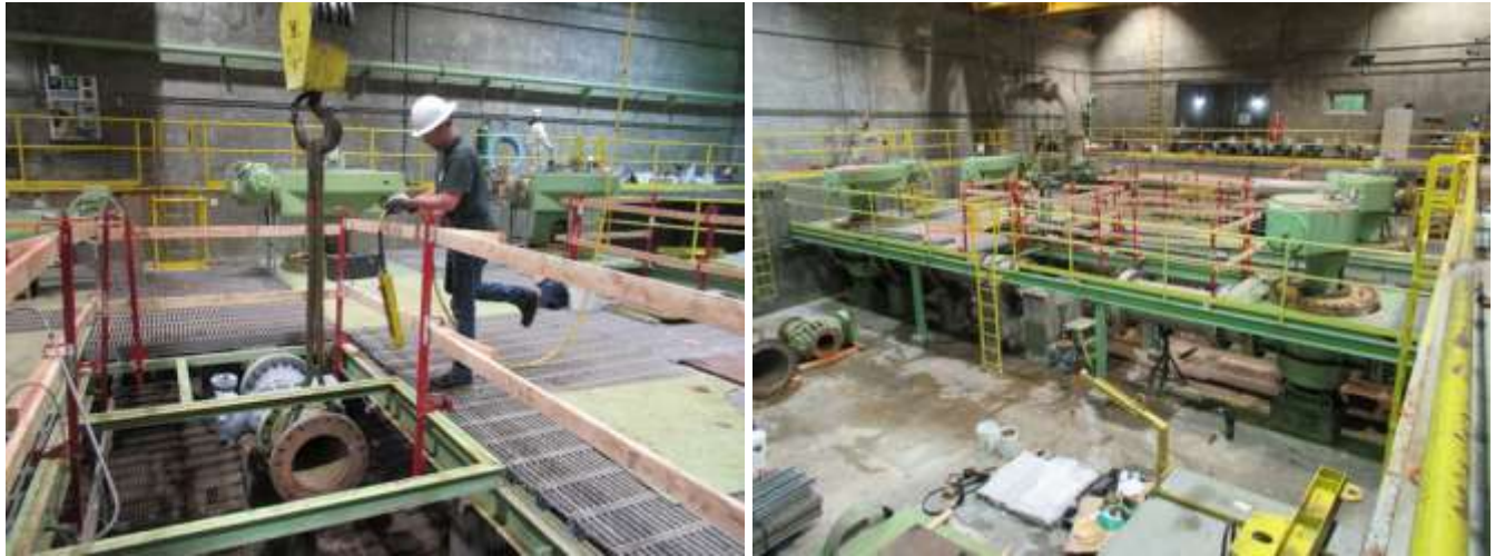
Staff replacing valves at Oak Street PCS
