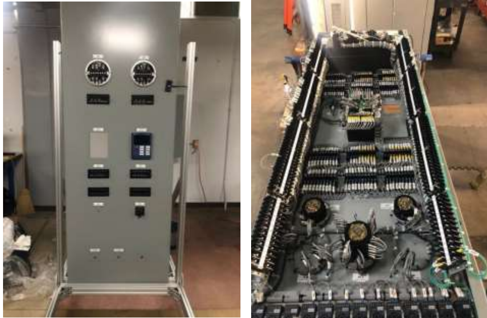
Front of transformer protection panel (left) and completed wiring in the back of the panel (right) at Hinds pumping plant
