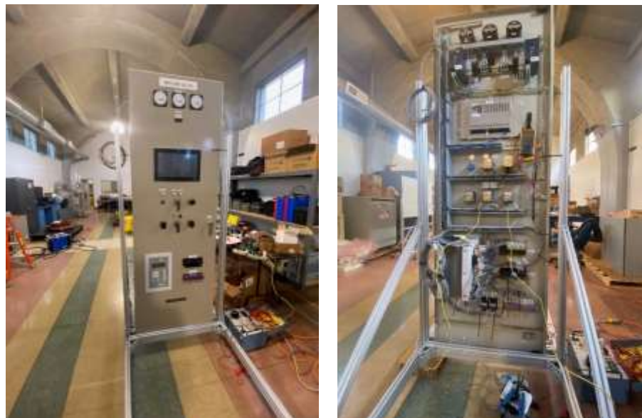
Front of AVR Panel (left) and completed wiring in the back of the panel (right) at Red Mountain HEP
