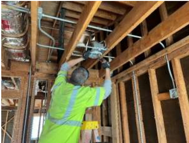
Staff installing recessed can lighting (left) and wiring a new light switch (right)
