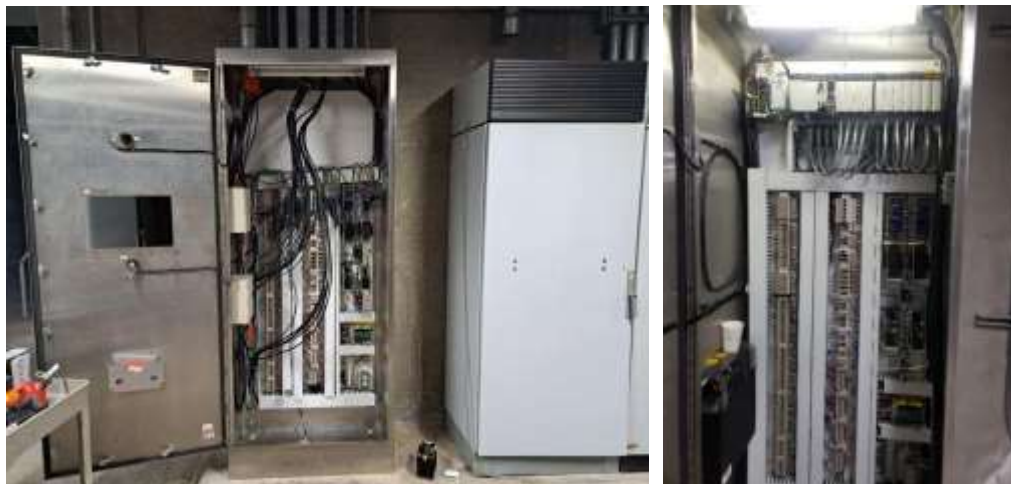
Previous PLC control panel (left) and new Allen Bradley PLC 5000 controller (right) at the Mills plant
