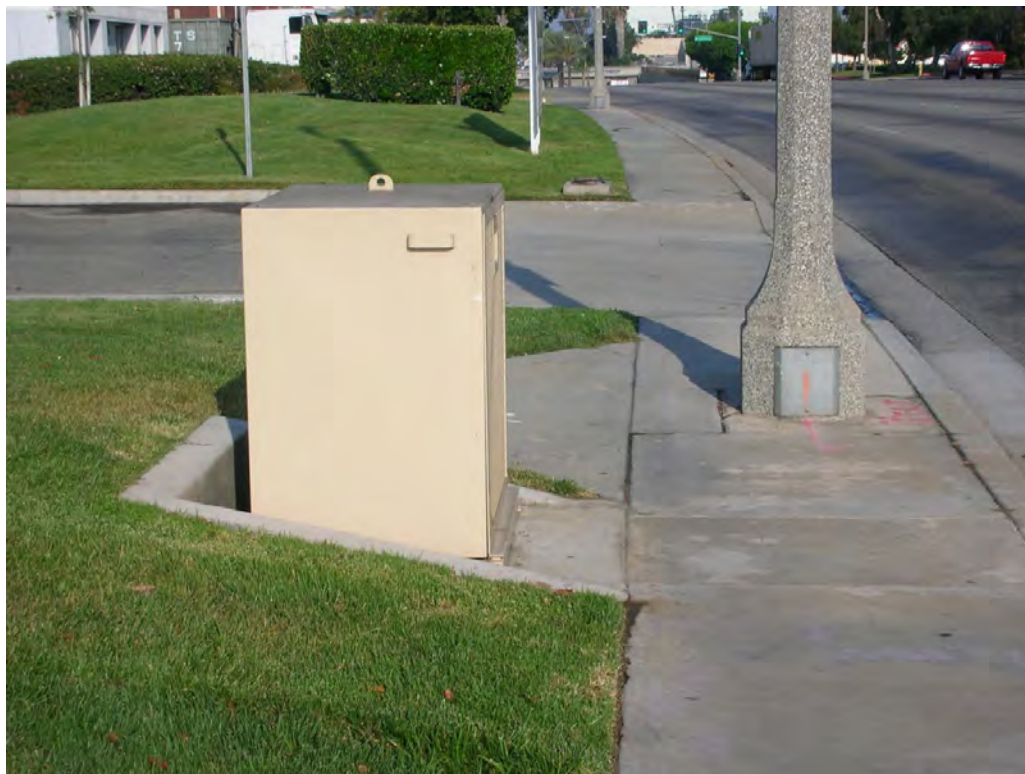
Figure 4. Typical Aboveground Valve Enclosure
