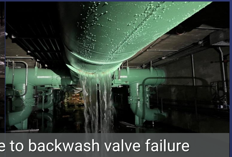
Repairing filter piping
