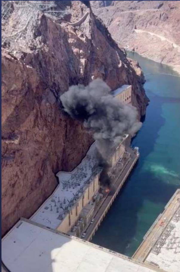
Explosion at Hoover Dam July 19, 2022
