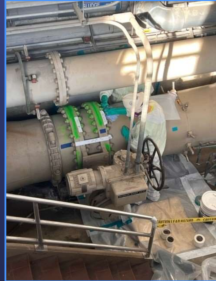
Lead Paint Abatement of backwash flow control valve
