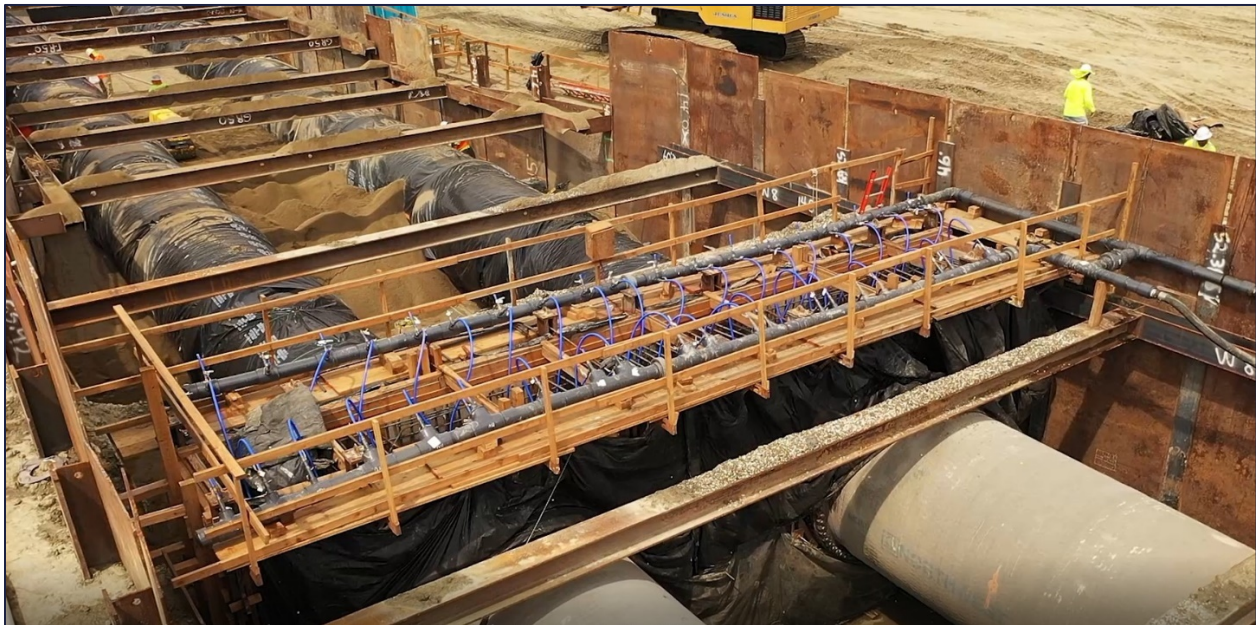
ERDIP to steel pipe transition thrust block construction with concrete temperature control system
