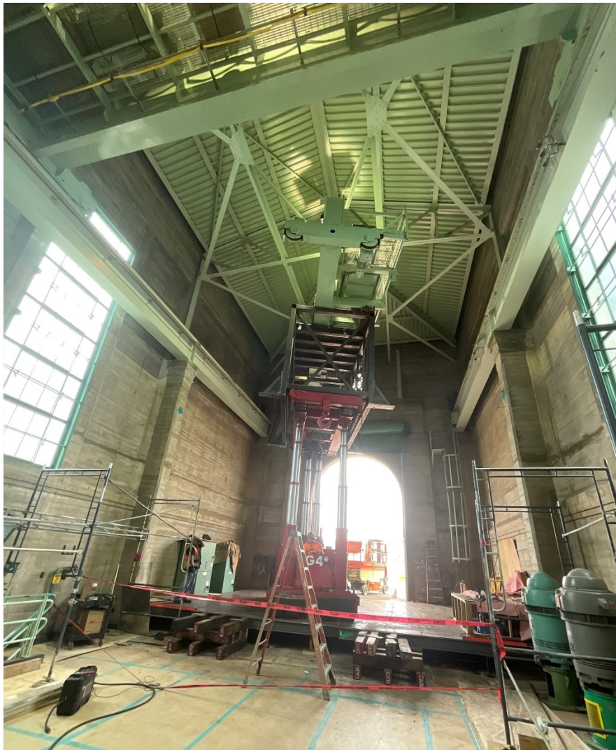
Contractor installing new crane girder at Gene Pumping Plant
