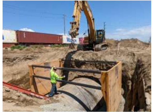
Installing shoring to repair minor leak on Upper Feeder near Fontana area
