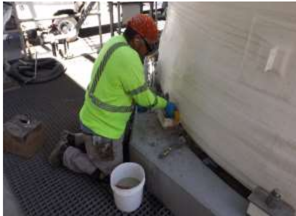
Staff grouting tie-down boxes to secure a chemical tank at Lake Mathews
