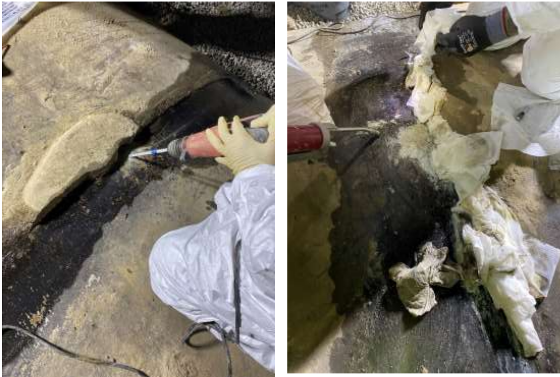
Staff drilling into pipe joints (left) to install injection ports (right) on the Upper Feeder
