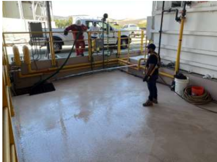
Containment area rinsed during chlorine scrubber maintenance at the Diemer plant
