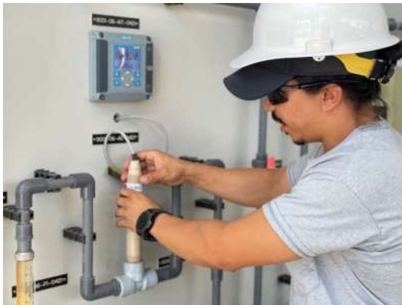
Staff replacing a pH probe on the UV effluent at the PWSC demonstration plant
