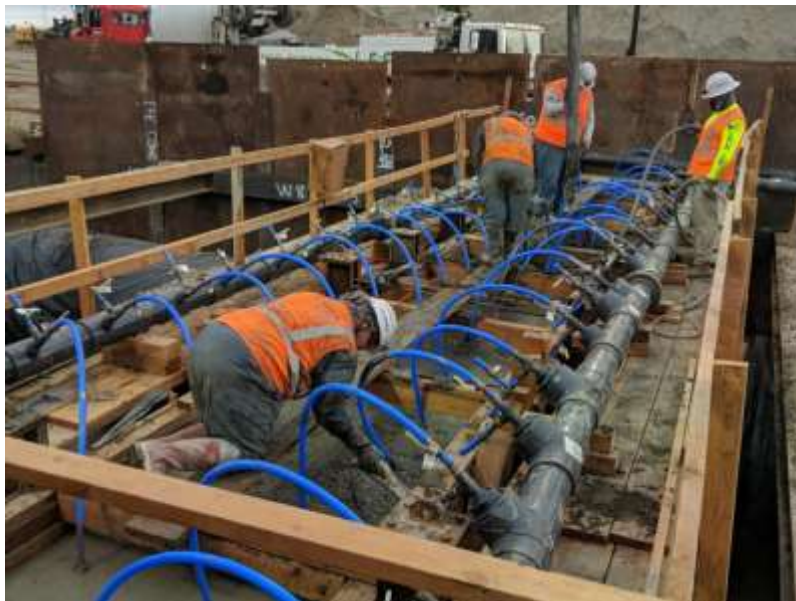
Casa Loma Siphon Seismic Upgrades—Thrust Structure No. 1 Concrete Finishing
