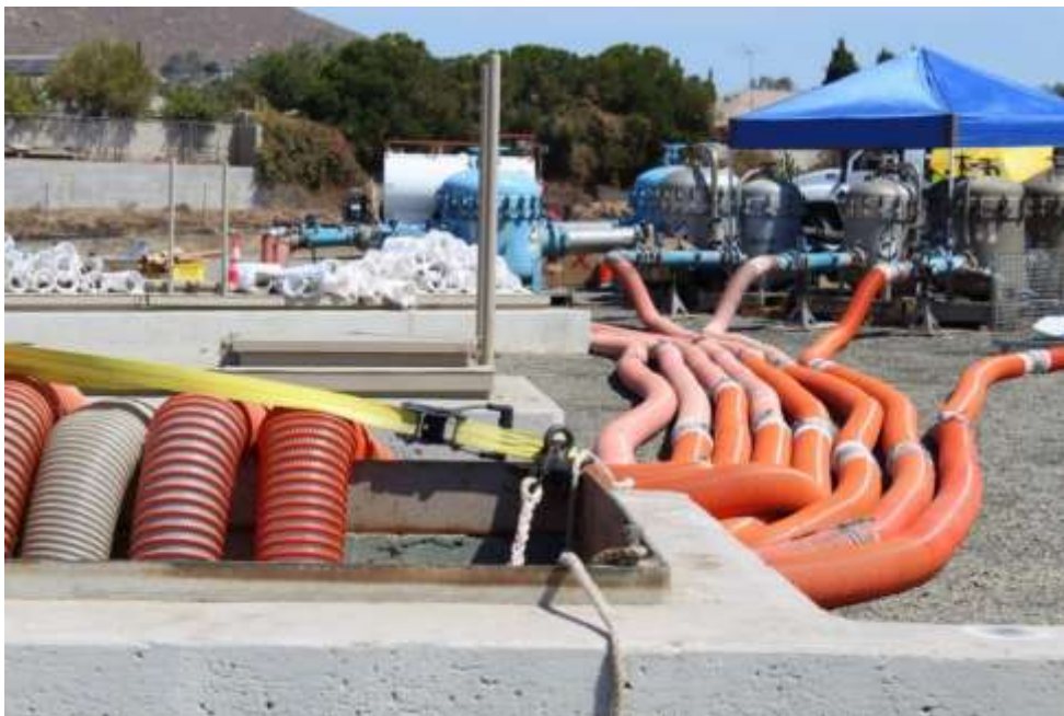
Staff set up a large-volume quagga mussel filtration system to safely dewater the Upper Feeder during the shutdown
