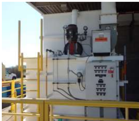
Chlorine scrubber at the Diemer plant
