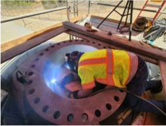
Staff welding thimble on the Upper Feeder at the Santa Ana Bridge crossing
