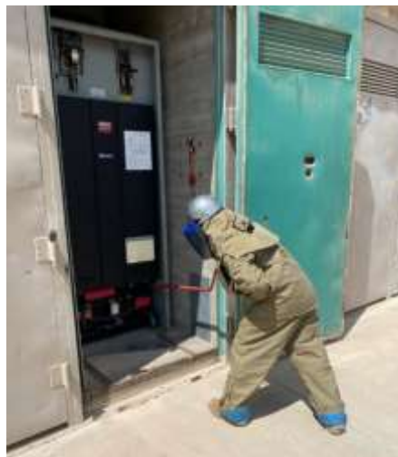
Staff racks out a 6.9kV circuit breaker to safely secure a pump for maintenance
