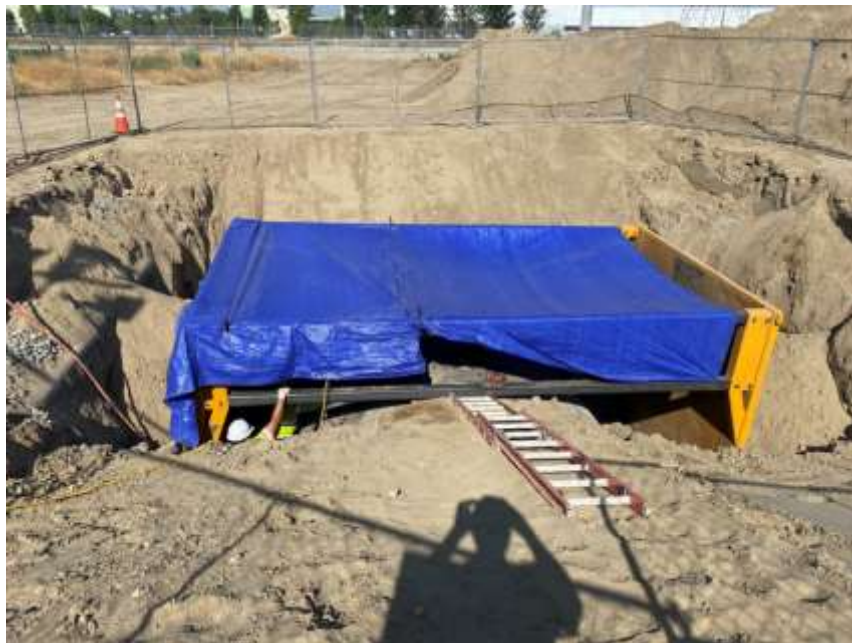
Staff excavated minor leak site on the Upper Feeder in the city of Rancho Cucamonga
