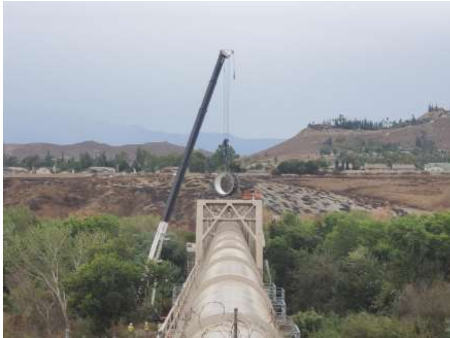
Contractor installing new slip joint for the Upper Feeder at the Santa Ana River bridge
