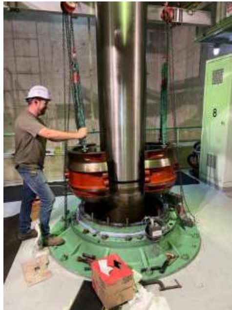
Staff replacing the intermediate bearing on a 12,500hp pump unit at Hinds pumping plant
