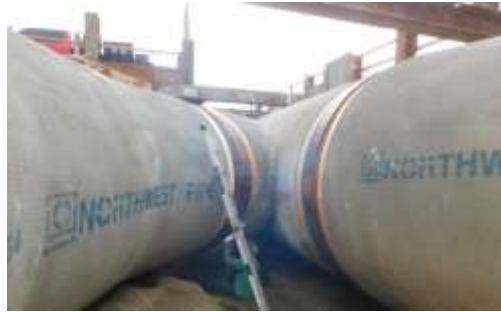
Casa Loma Siphon Seismic Upgrades—Welding 104-Inch Butt Strap on Welded Steel Pipe Wye Branch
