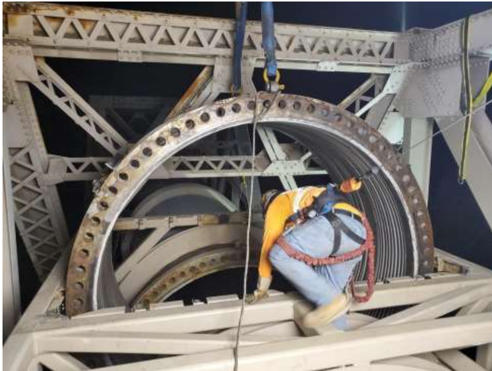
Contractor removing failed bellows joint from the Upper Feeder at the Santa Ana River bridge
