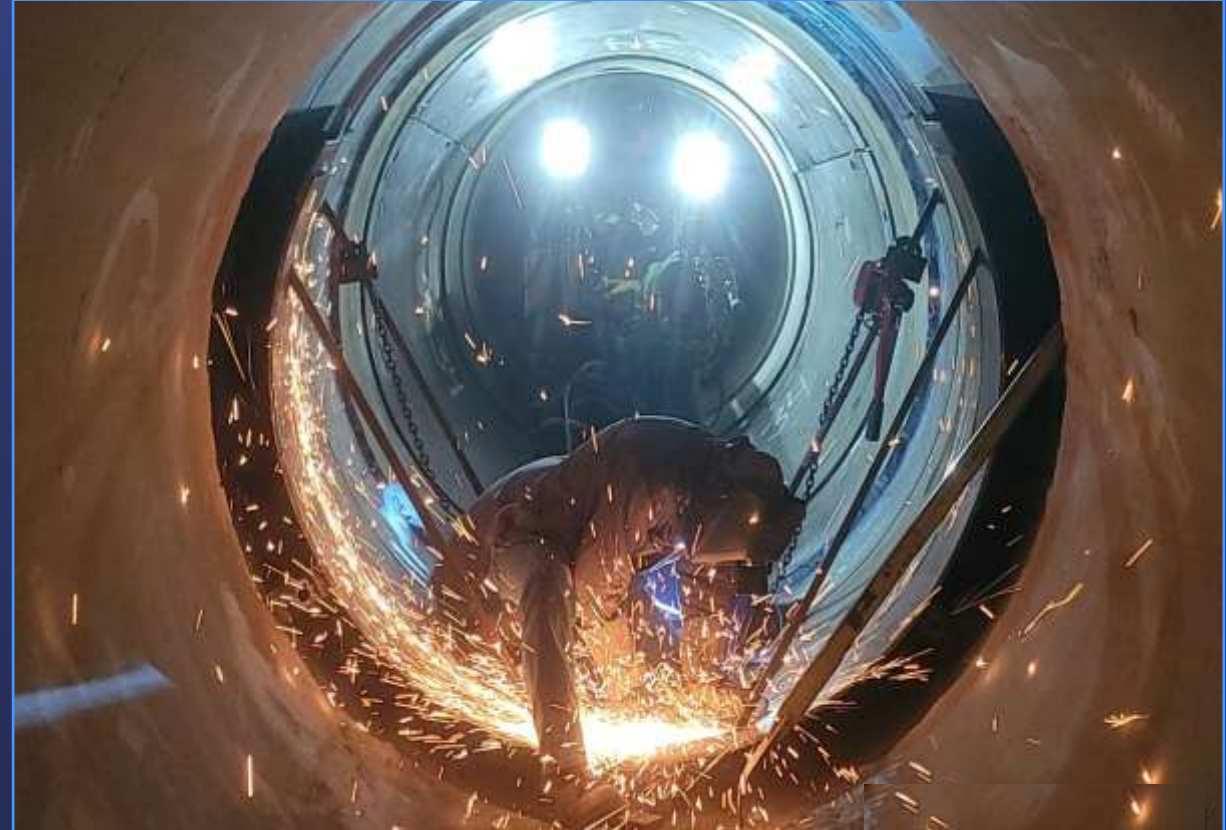
Second Lower Feeder – PCCP Rehabilitation
