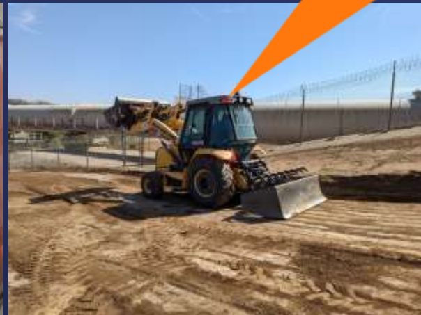
Clearing and Grading for Crane Pad
