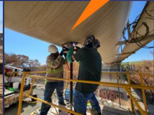
6-inch Valve Installation
