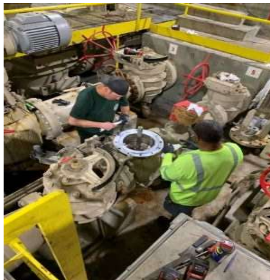
Staff rebuilding a globe valve at the San Gabriel PCS on the Lower Feeder
