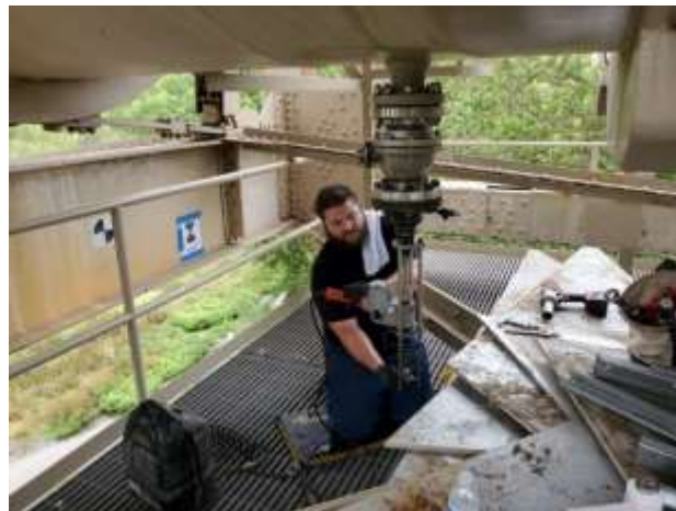
Contractor performing final hot tap of a flange and valve assembly on the Upper Feeder at the Santa Ana River bridge
