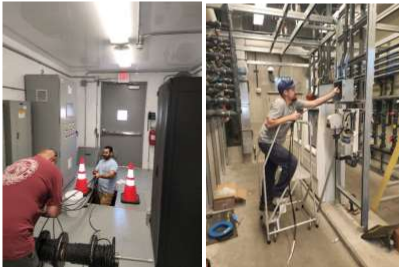
Staff installing SCADA cables (left) and power cables (right) for an additional chlorinator at the Weymouth plant
