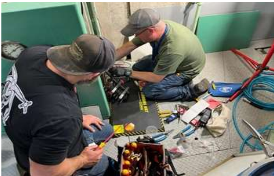
Staff repairing the discharge valve electrical components for the oil system at Hinds pumping plant
