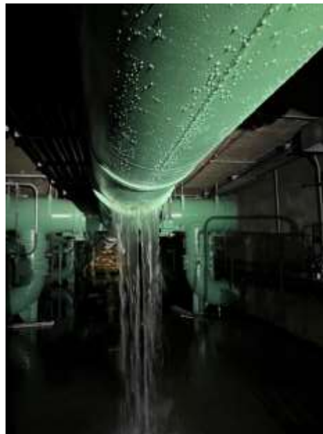
Separation of the backwash piping and flooding in the filter gallery at the Diemer plant
