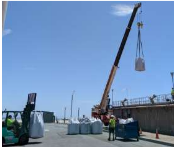
Staff using a crane to replenish filter media at the Diemer plant
