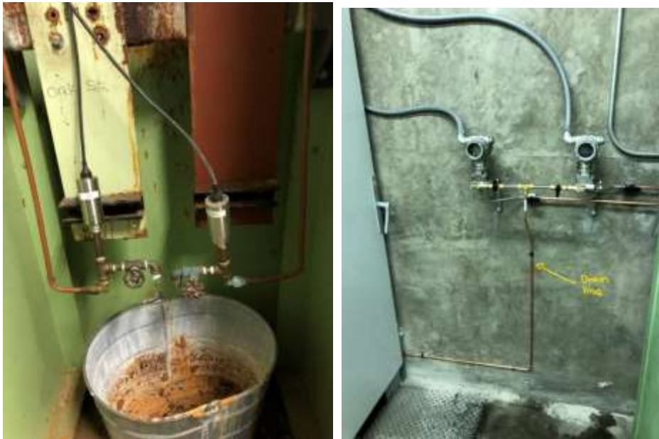
Before (left) and after (right) differential pressure cell replacement at Oak Street PCS
