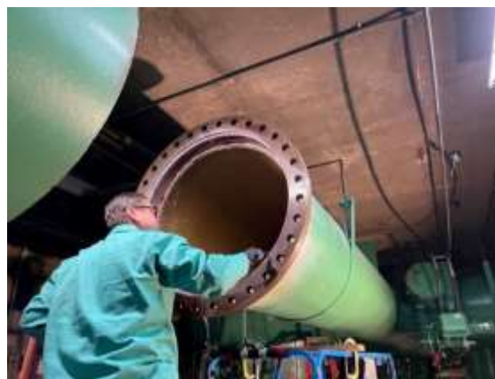
Staff welding a new flange on the backwash header piping at the Diemer plant
