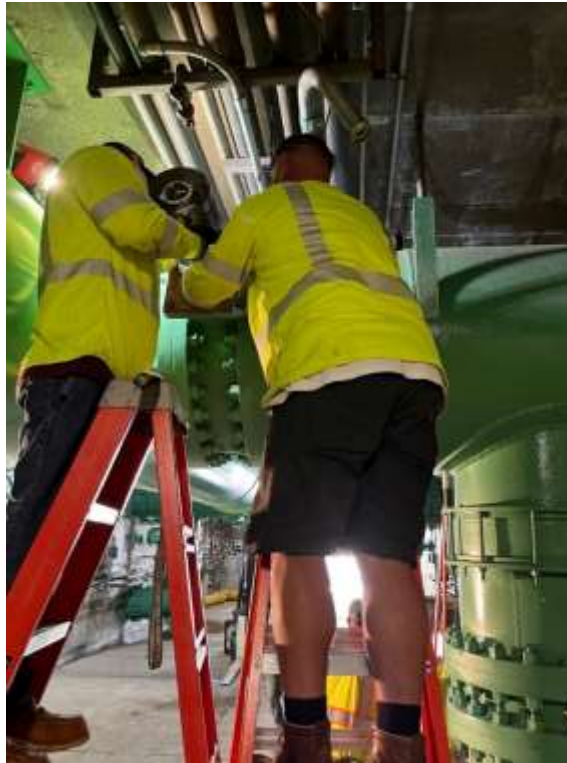
Staff replacing the backwash valve shear key at the Diemer plant
