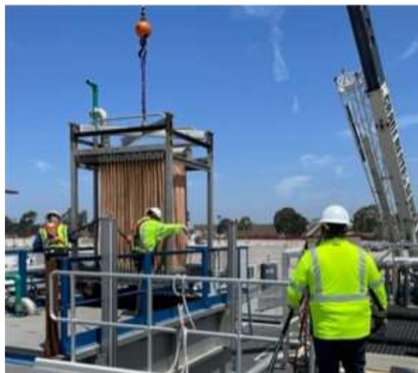
Staff intentionally damaging MBR fibers for challenge testing (left) and reinstalling the MBR cassette (right) at the demonstration facility
