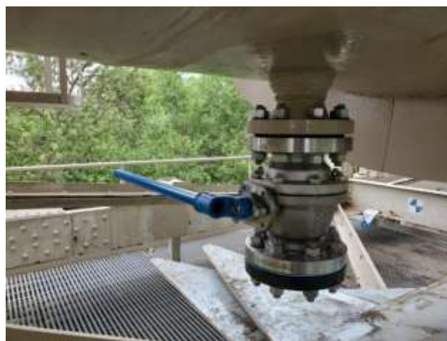
Installed flange and valve assembly on the Upper Feeder at the Santa Ana River bridge
