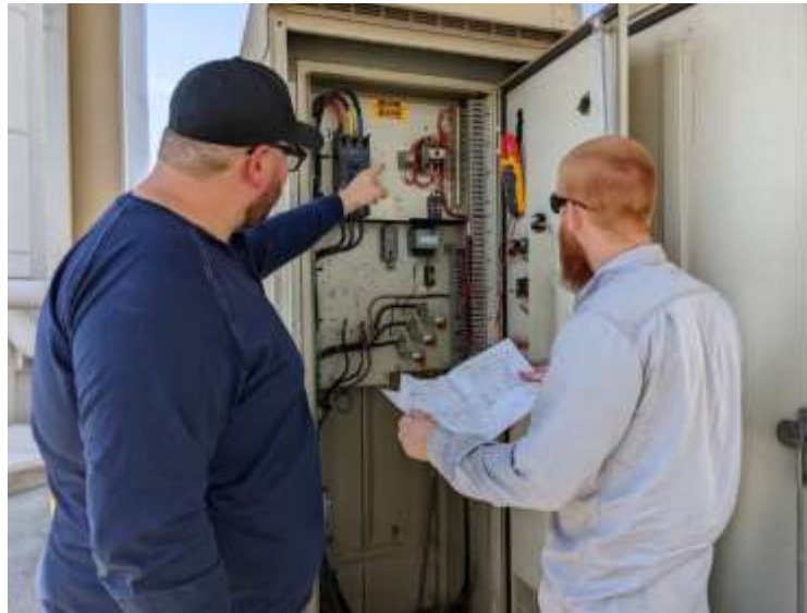
Electrical apprentice and journey installing a new variable frequency drive at the Diemer plant
