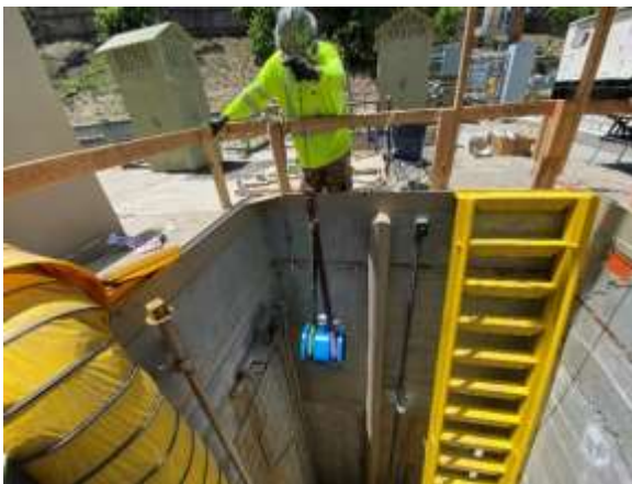
Staff installing a new magnetic flow meter (left) and the meter installed (right) for service connection WB-06B on the Palos Verdes Feeder
