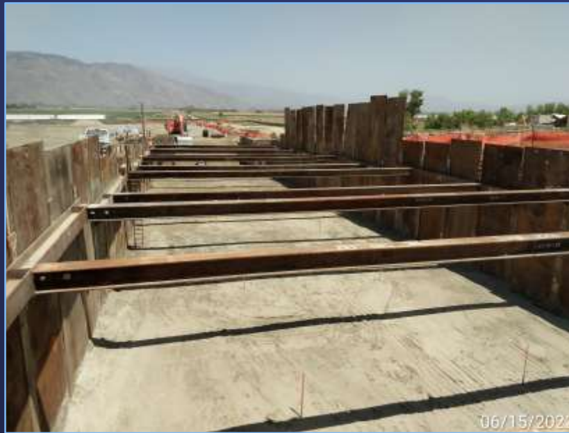
Supported Excavation for ERDIP Pipe
