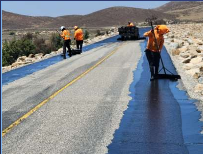
Slurry Paving of Dam Access Road
