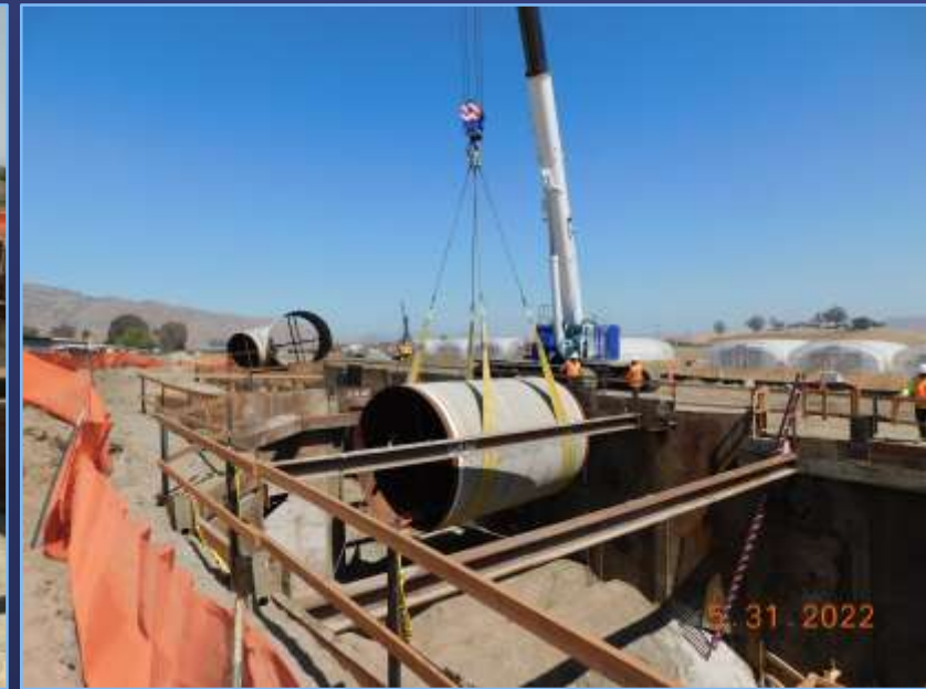
Placement of Steel Transition Pipe
