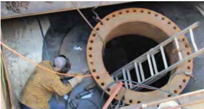
Welding Pipeline Outlet
