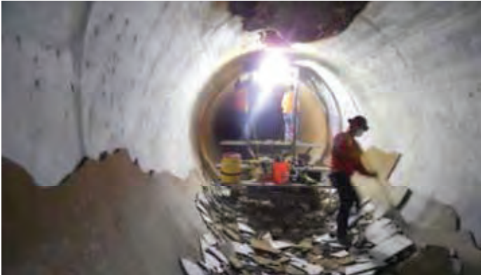
Mortar Lining Removal
