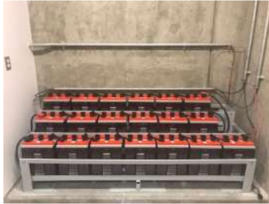
New batteries for high-voltage switchgear at the Jensen plant
