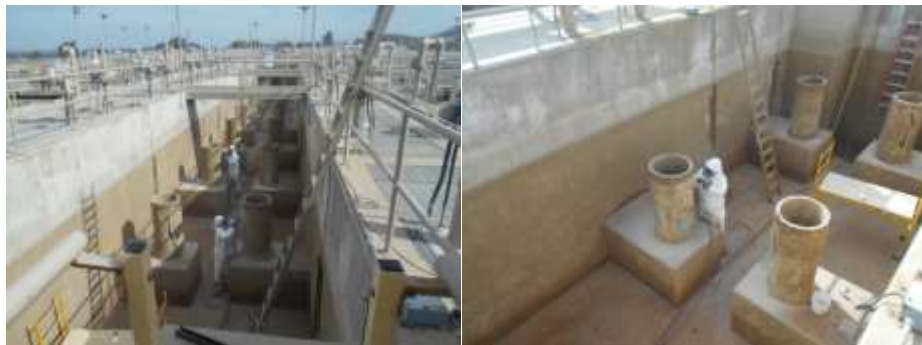
Staff chipping mortar lining on filter inlet goosenecks at the Skinner plant
