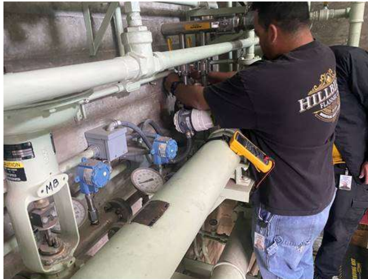
Staff troubleshooting an oil flow meter at a desert pumping plant
