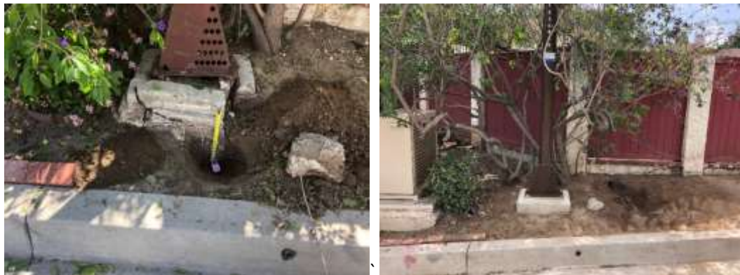
Corroded vent stack and damaged footing (left) and repaired vent stack and footing (right) on the Palos Verdes Feeder
