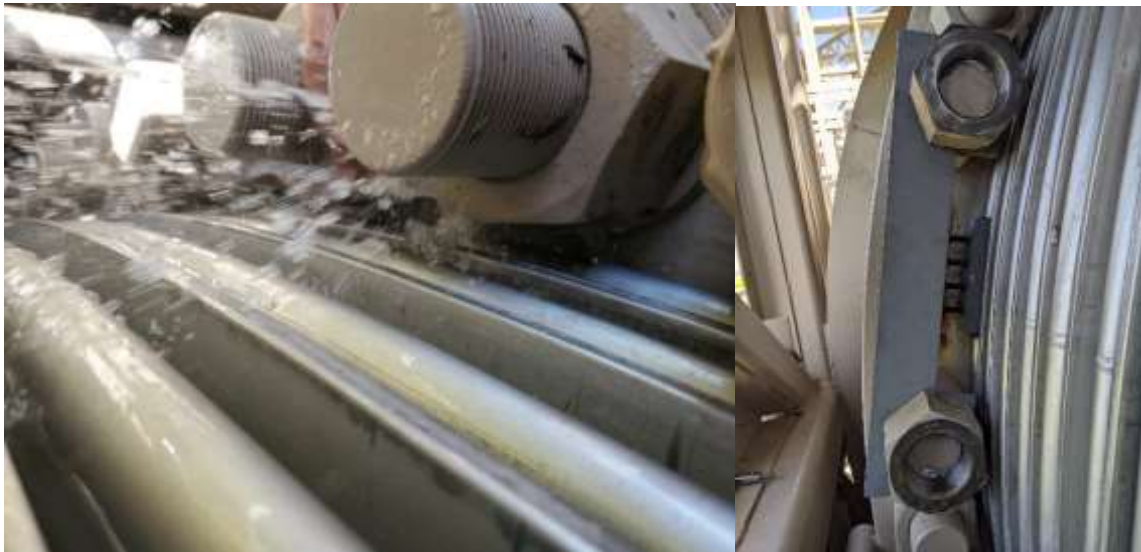
Leak on Upper Feeder bellows expansion joint (left) and temporary repair with custom bracket and plate (right)
