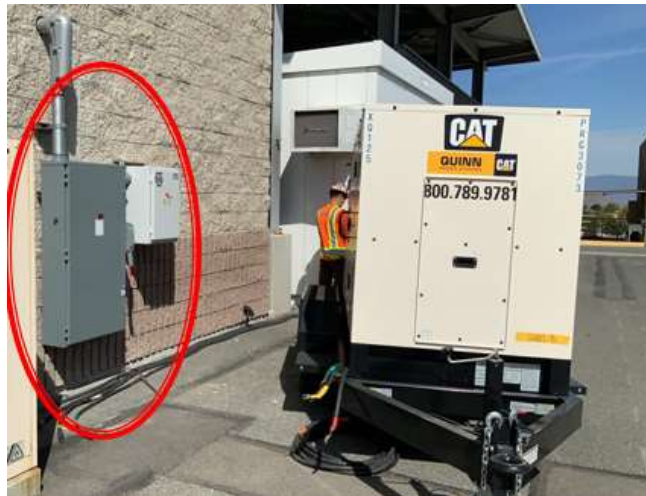
New generator connection point installed at the Mills plant
