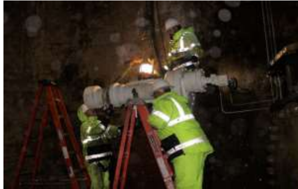
Staff installing hydraulic actuator at Tier 5 of the Lake Skinner outlet tower
