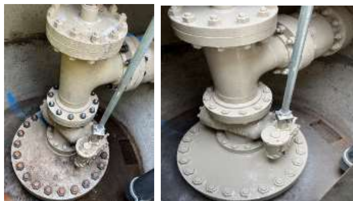
Vacuum air release station before (left) and after (right) coatings on the Second Lower Feeder
