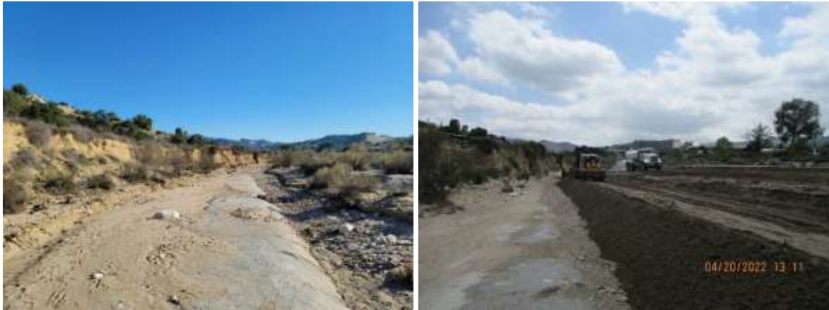
Exposed concrete section of the Foothill Feeder (left) and processing and placing fill material over the feeder (right)
