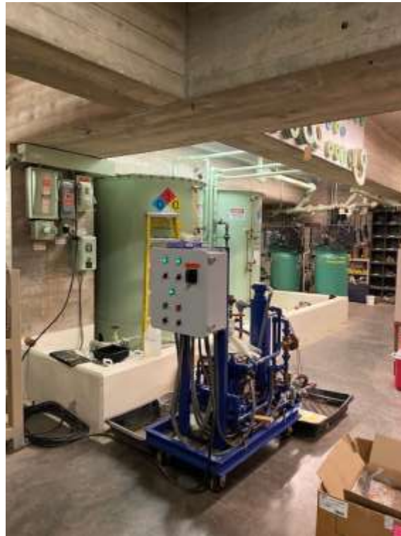
Processing used oil for re-use at a Desert pumping plant
