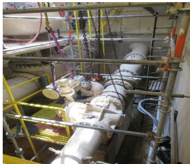
Staff removing the plug valve in the OC-44 service connection turnout structure on East Orange County Feeder No. 2
