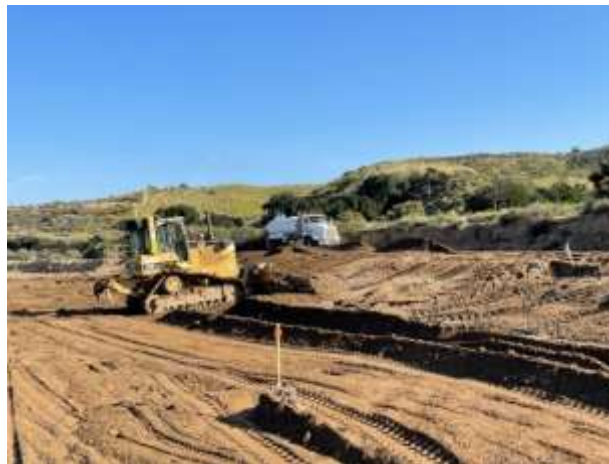
Cutting the slope for the fill placed over the Foothill Feeder
