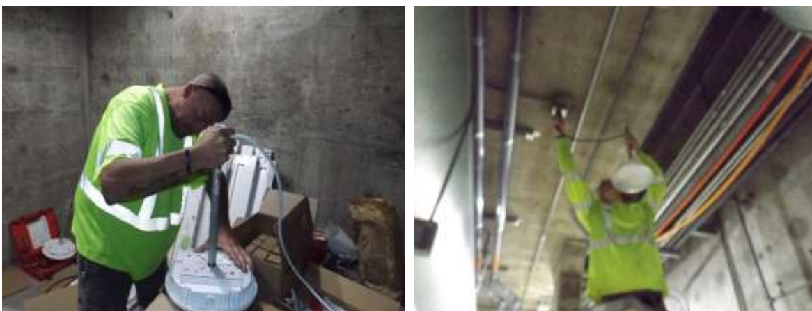
Staff assembling and installing new LED fixtures at the Weymouth plant
