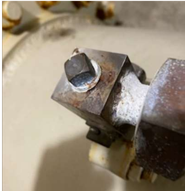
Old valve coupling before replacement along the Middle Feeder
