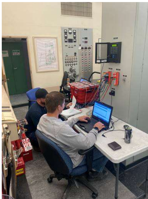
Staff testing replacement motor management relay at a Desert pumping plant
