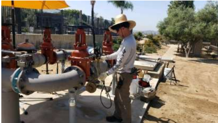
Staff testing and certifying newly installed backflow devices at the Weymouth plant
