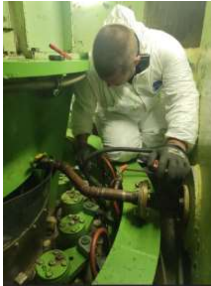
Staff making final adjustments to the wicket gates at Foothill HEP
