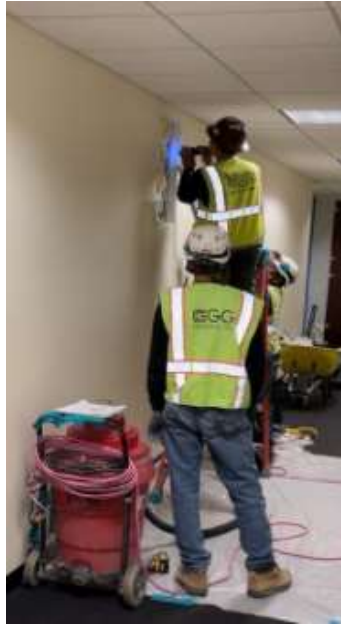
Headquarters Building Improvements—Replacement of fire alarm device
