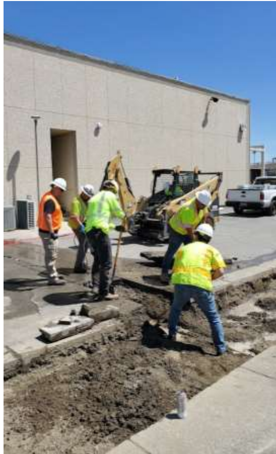
Staff excavating a sample line for repairs at the Skinner plant
