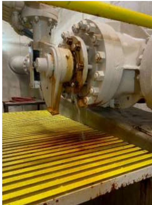
Leak on a plug valve at the OC-44 service connection turnout structure on East Orange County Feeder No. 2
