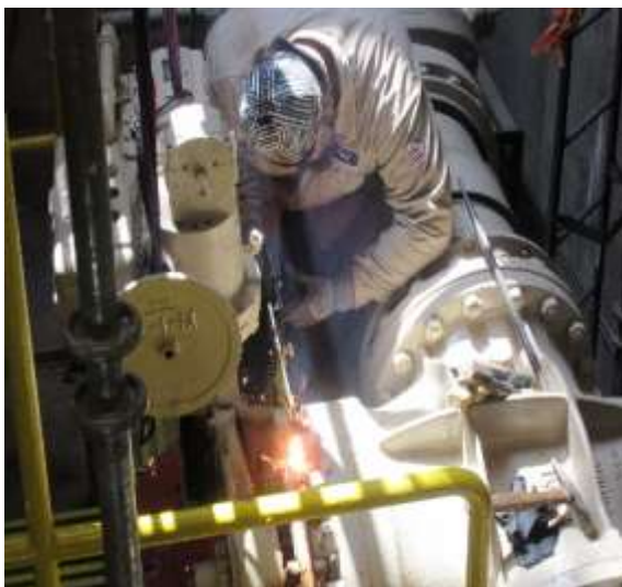
Staff removing the plug valve in the OC-44 service connection turnout structure on East Orange County Feeder No. 2
