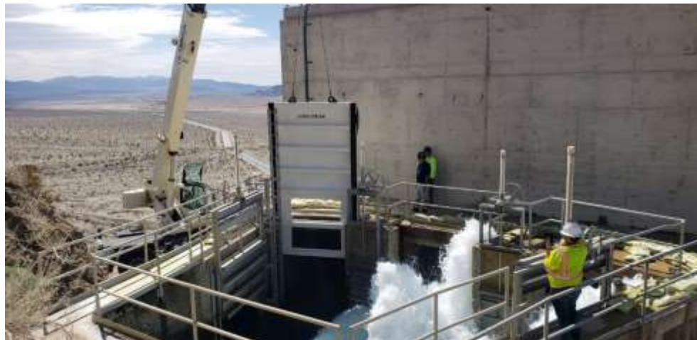
Staff removing the orifice gates at Hinds pumping plant
