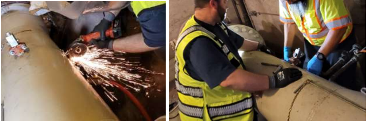
Staff cutting corroded bolts to remove hardware (left) and installing new hardware (right) for revenue meters along the Middle Feeder
