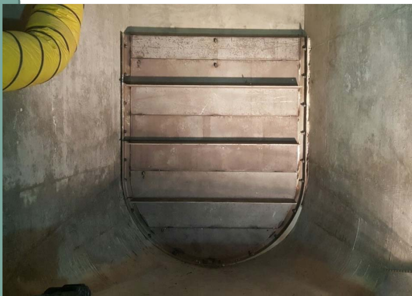
Example of a temporary bulkhead that will be installed on Second Lower Feeder Reach 3A
