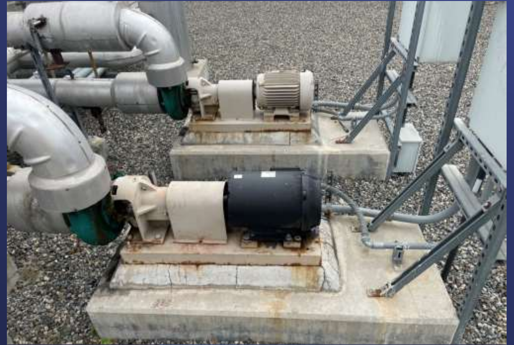
Existing chilled water pumps
