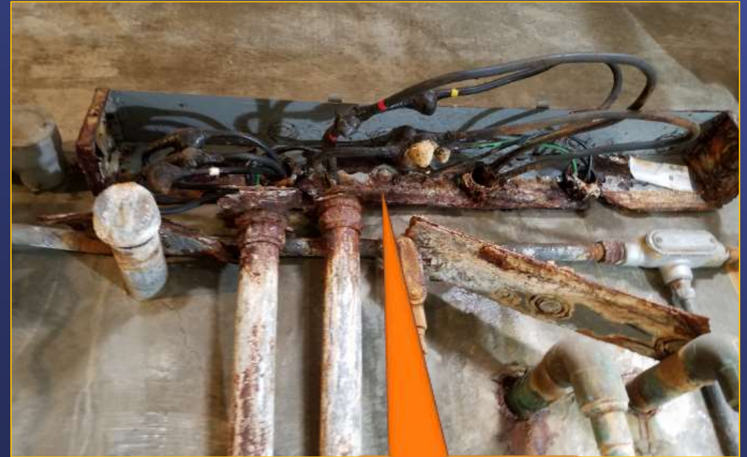
Corroded Equipment
