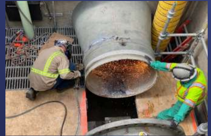
Pipe Spool Removal
