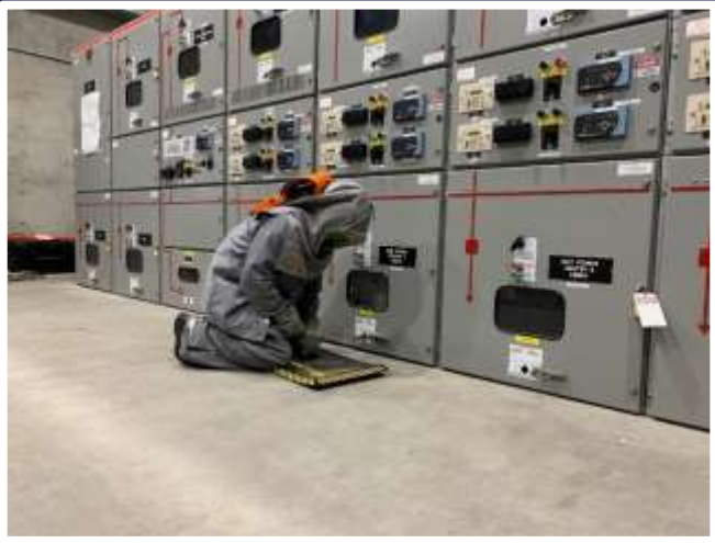
Staff isolating equipment for maintenance at Skinner WTP
